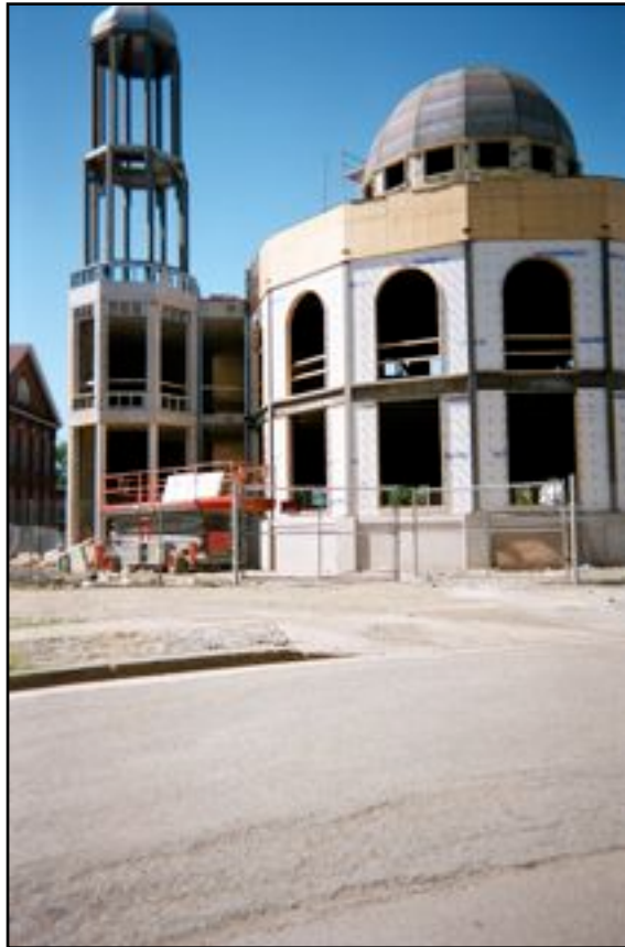
Photograph 85: UMMAH Under Construction (Amira 2009)
