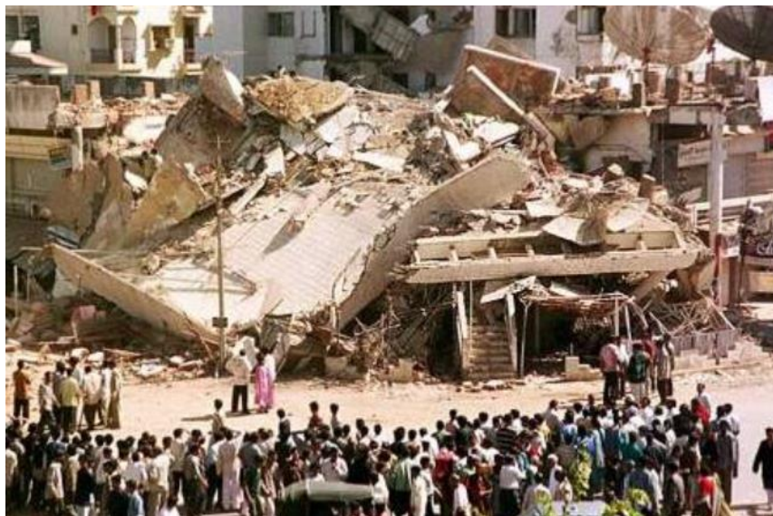
Fig. 4. Map showing collapsed buildings on the west side Image source: (Sairam et al., 2015)
