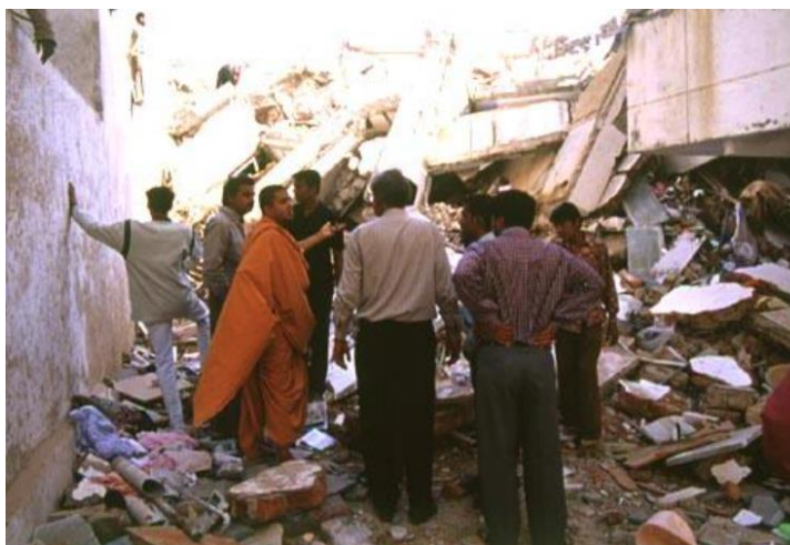
BAPS workers near collapsed building sites, Ahmedabad, 2001
