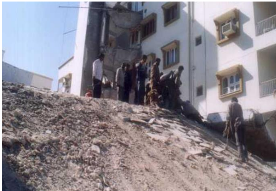
Picture of collapsed wing of Sangemarmar building, 2001
