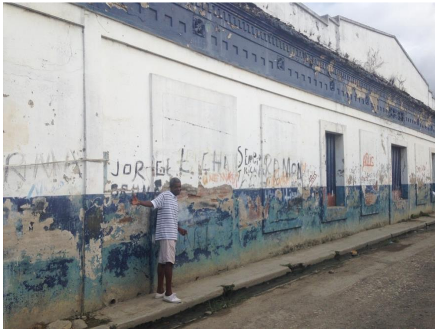
Figure 12: I stop to snap a photo of the common sight of unfinished roads and sidewalks that frustrated so many of those I spoke with, as a friend jumps in front of the camera asking, “Do you want me in your photo?” Photo by author, 2017.
