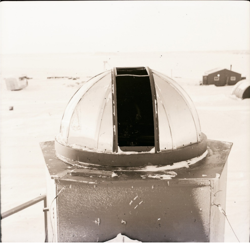
Figure 4. Isachsen's pibal dome, 1953. If you zoom in, you can see the theodolite inside the dome. Bill Nemeth personal collection.
