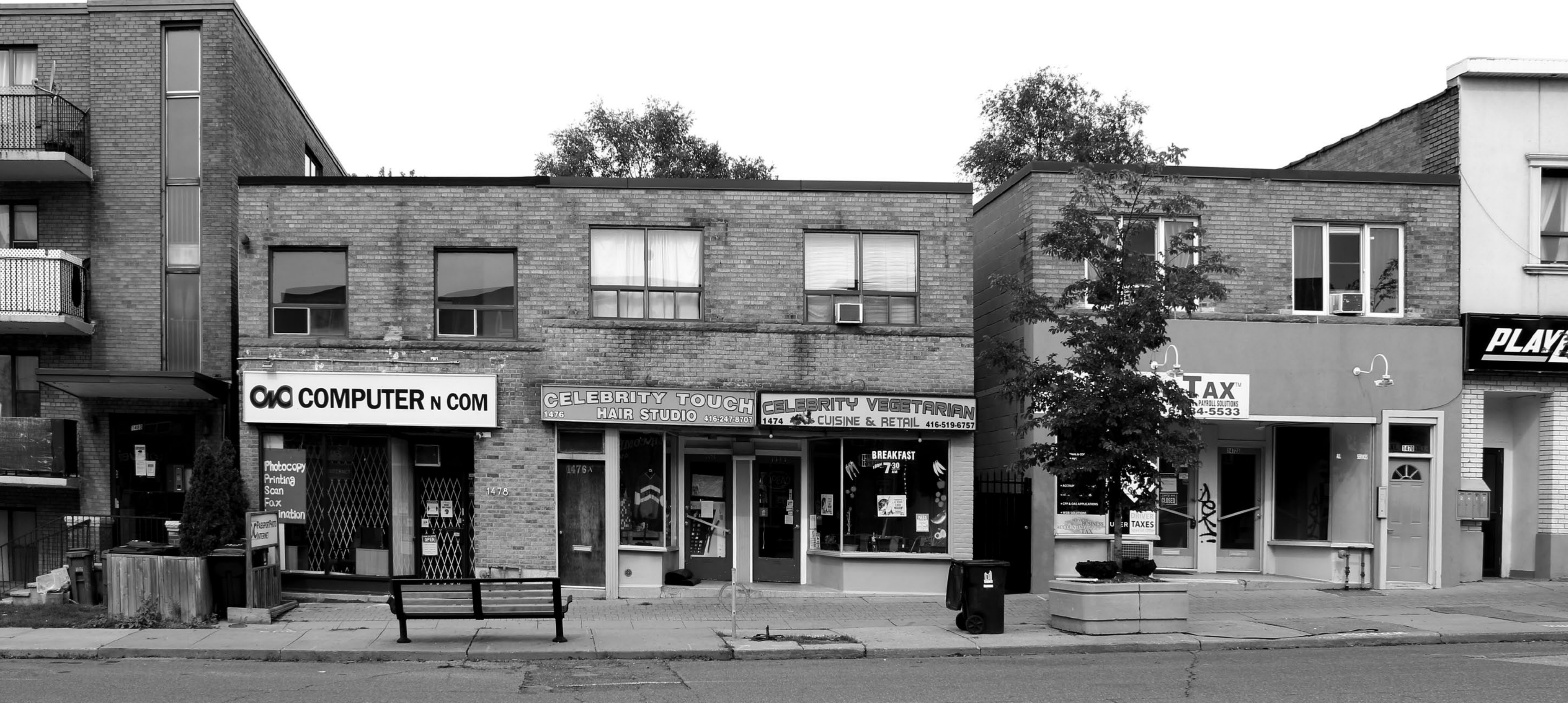
Fig. 050 1474-1480 Eglinton Avenue West photograph showing the frontage on August 15, 2021.
