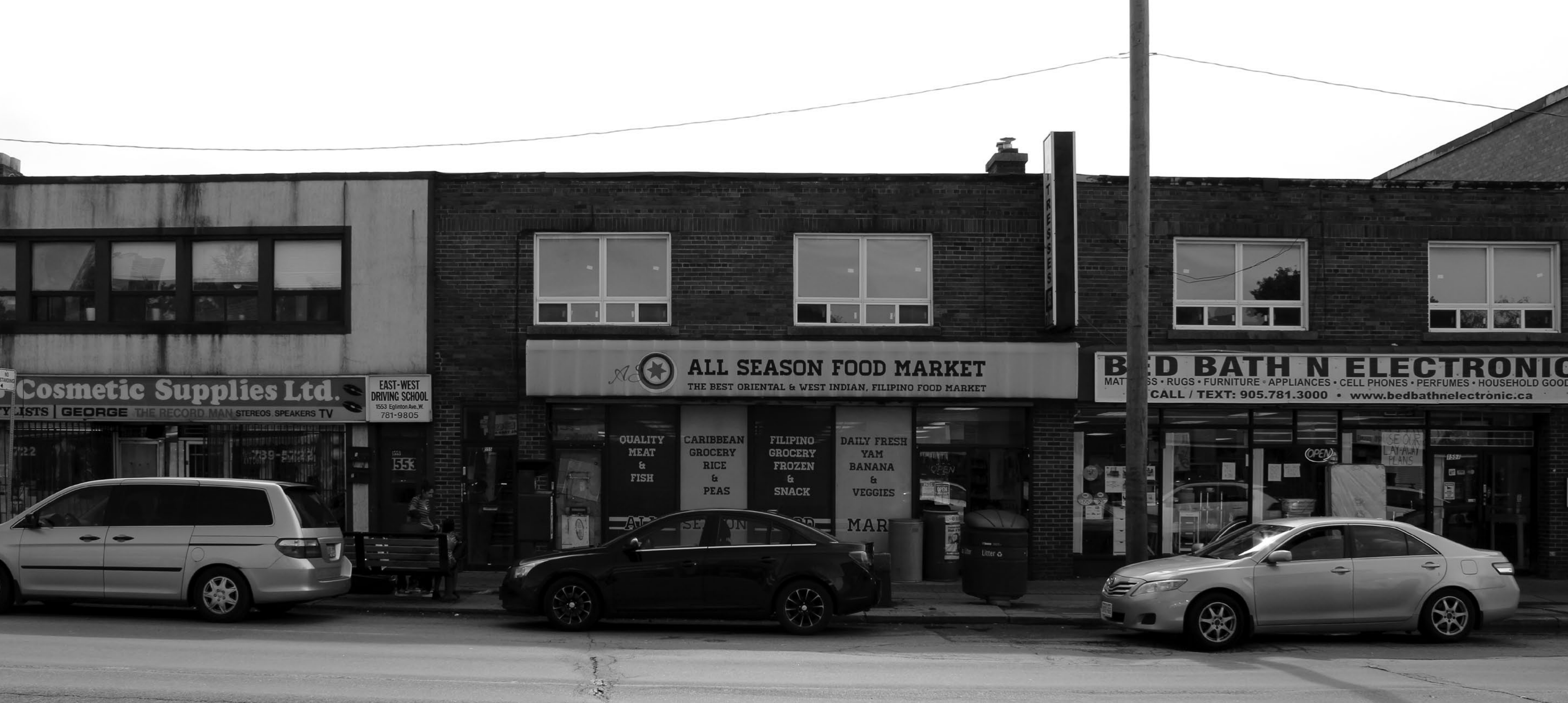
Fig. 042 1555-1557 Eglinton Avenue West photograph showing the frontage on August 15, 2021.
