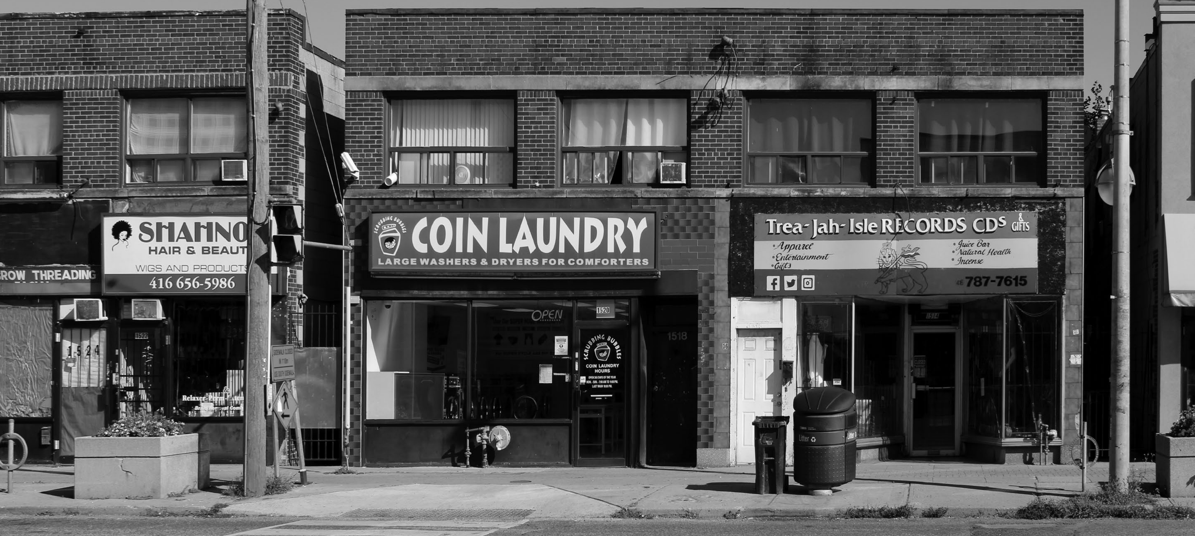
Fig. 047 1514-1520 Eglinton Avenue West photograph showing the frontage on August 15, 2021.
