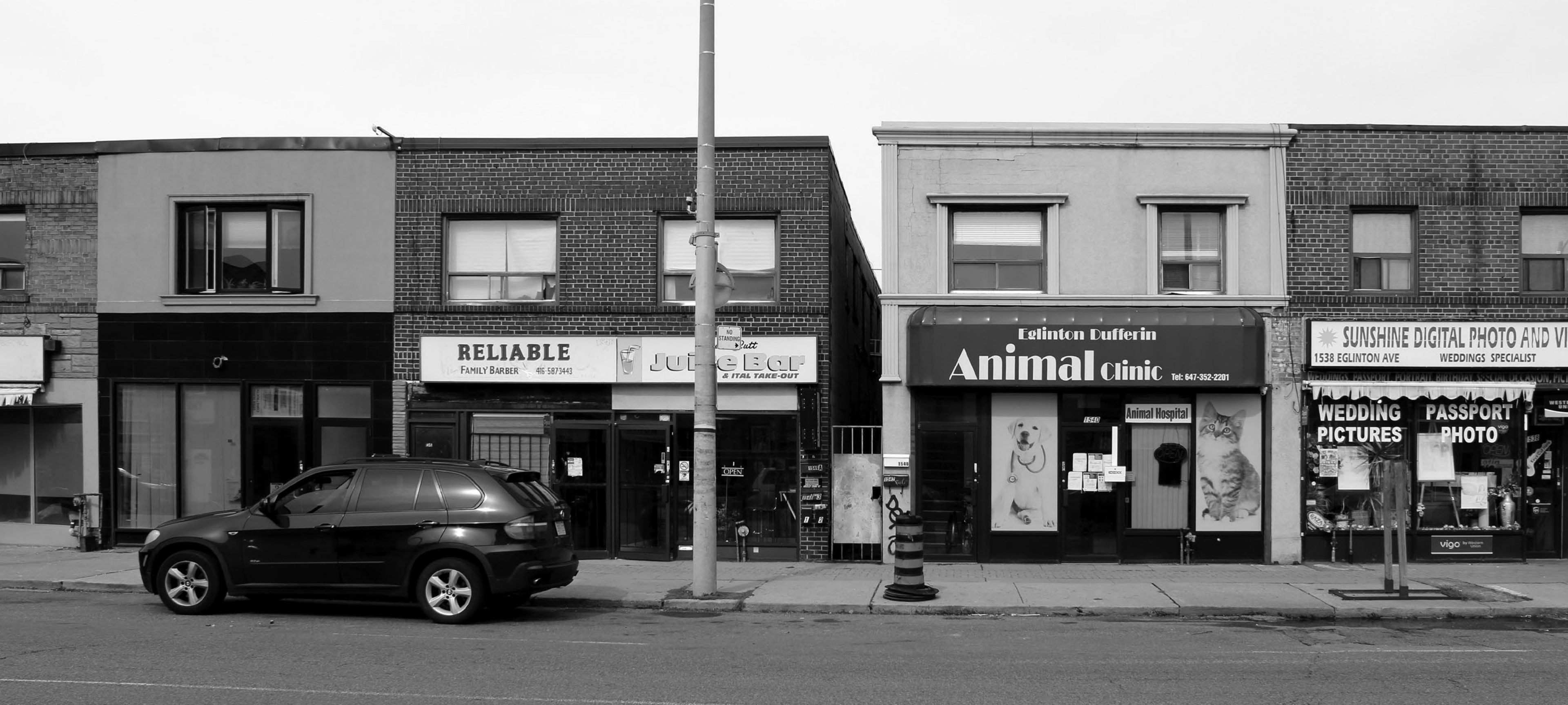
Fig. 045 1542-1547 Eglinton Avenue West photograph showing the frontage on August 15, 2021.
