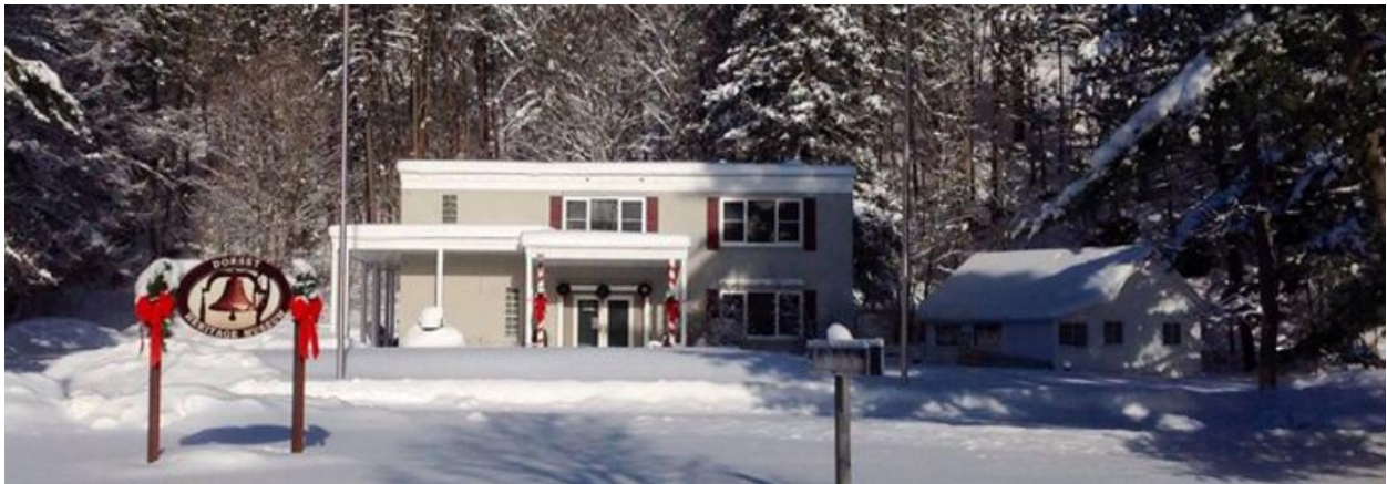
Fig 2. Dorset Heritage Museum in Winter. Former Forest Ranger Base, the site has undergone extensive renovations in order to become the fully operating museum that is on site today. image: Dorset Heritage Museum
