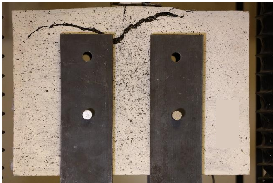
Figure 5-19 Surface cracking at termination of the experiment for specimen CMK2-5-B.
