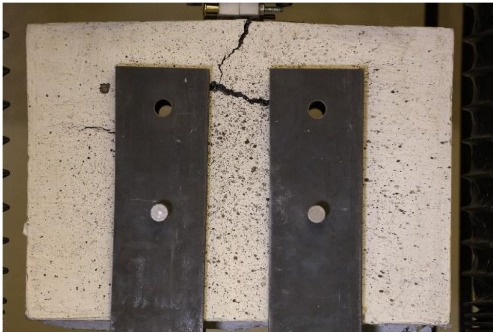
Figure 5-65 Surface cracking at termination of the experiment for specimen IHRT2-5-B.
