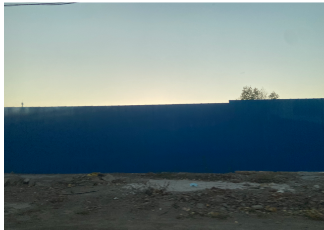
Figure 52. Site of demolished Luoma Lake Art District in 2022. Photograph by the author.
