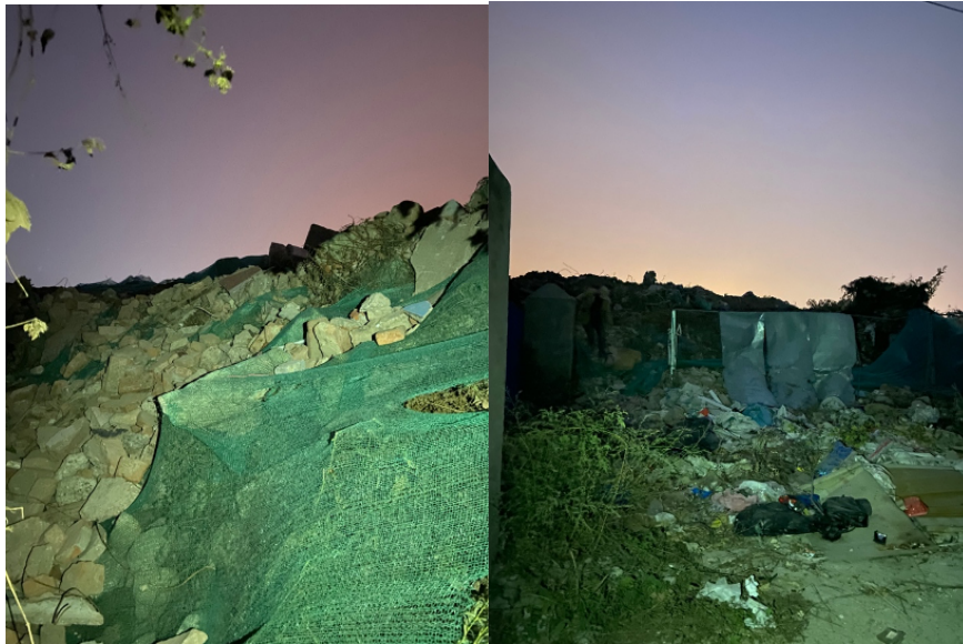
Figure 39. The demolished site of 1005, 2022. Photographs by the author.
