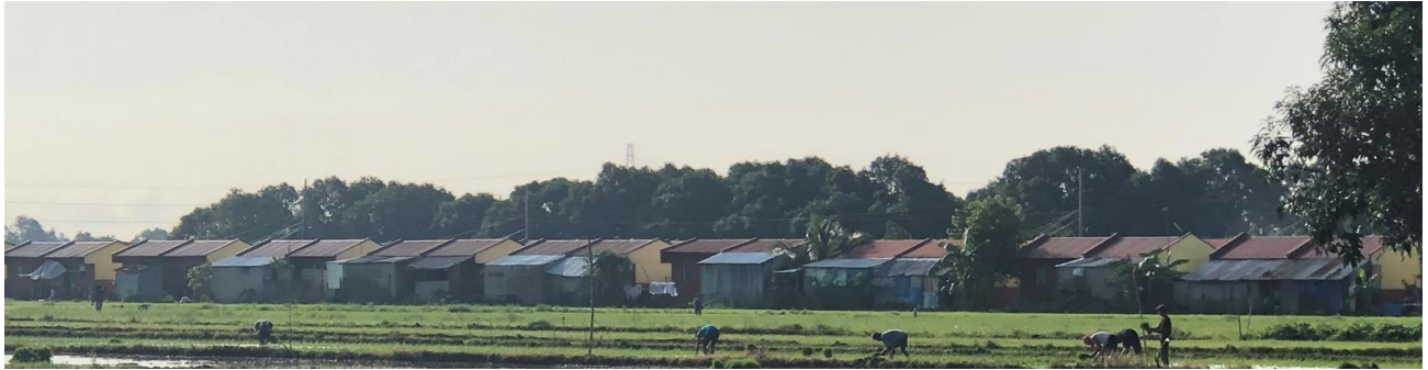
Figure 13 Vancouver Homes village with units that have concrete block kitchens attached.
