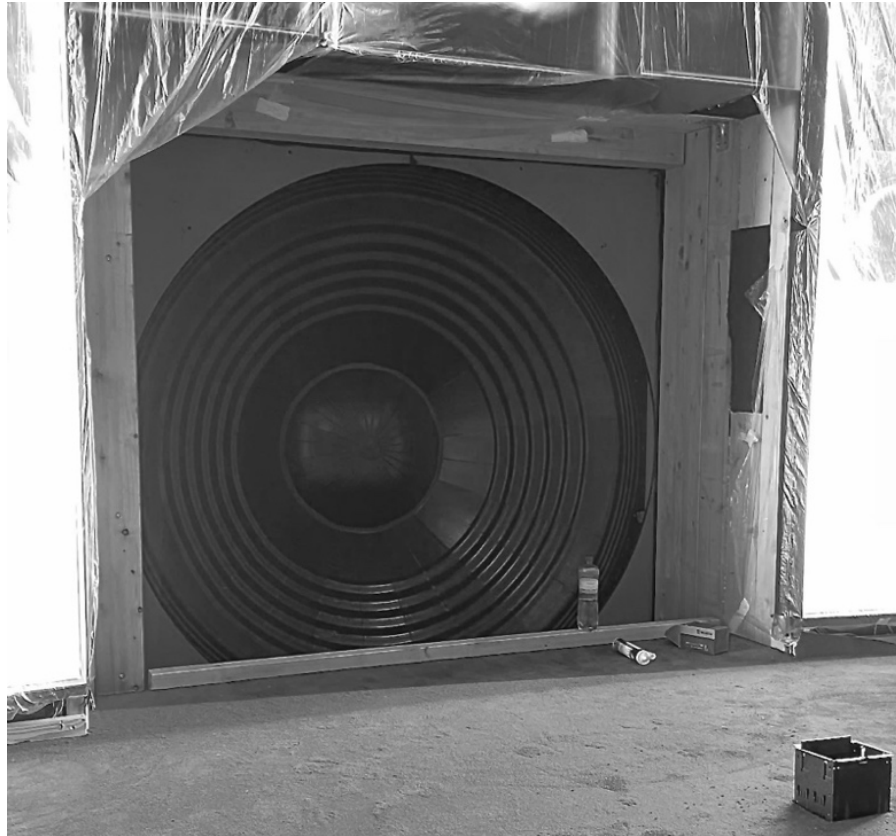
Figure 5: The ASCENDO 80” cinematic subwoofer is custom designed for infrasound.
