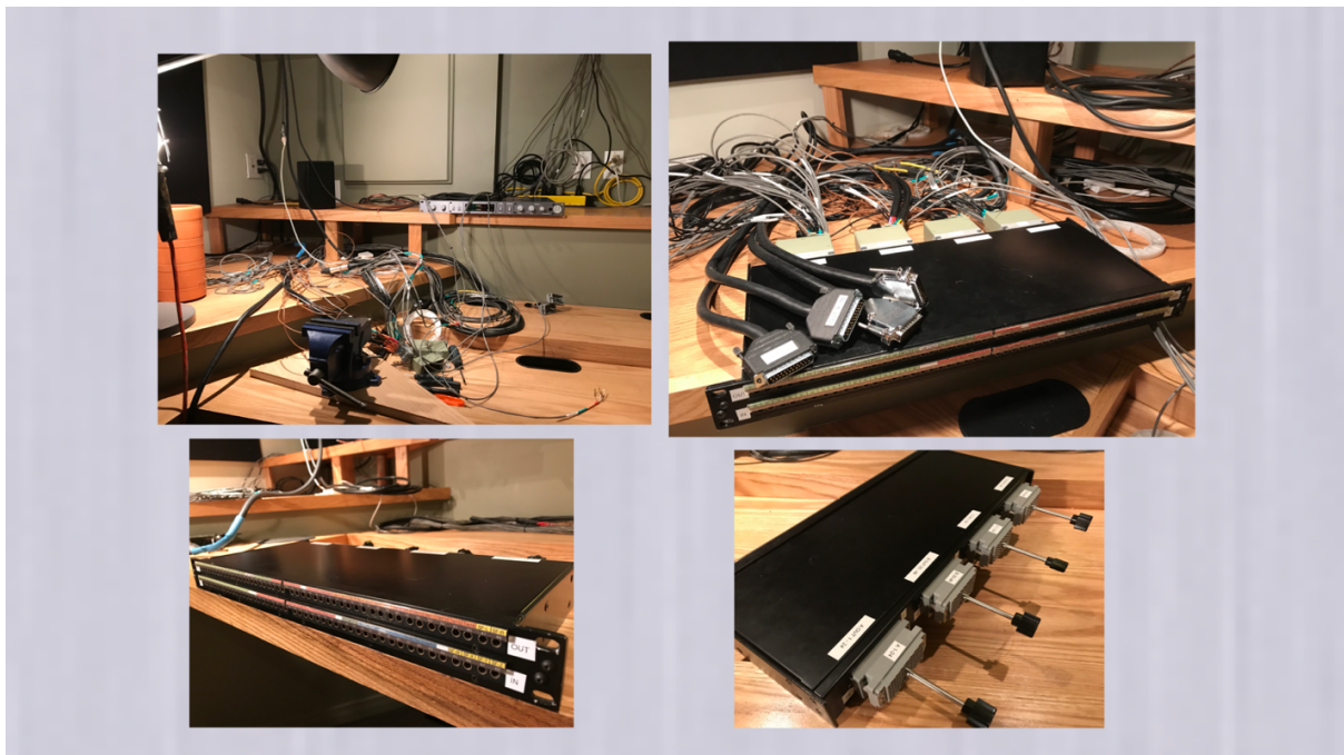
Figure 33: Building the HN-FTS, patch bay with connectors.
