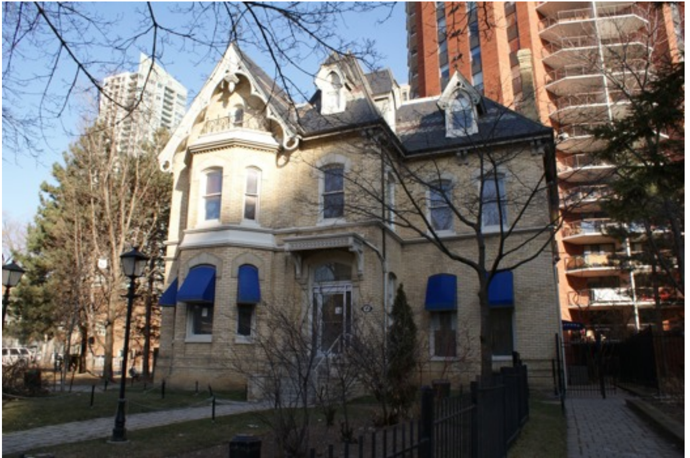
Figure 6.1: 471 Jarvis Street, Toronto
