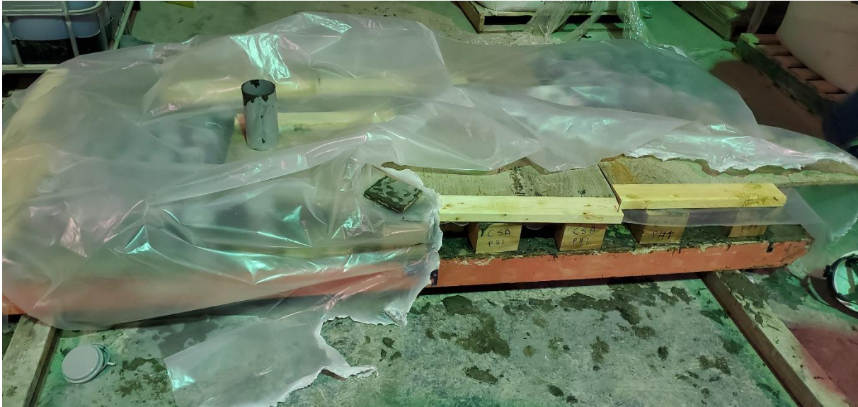
Figure 21: Filled mold covered with plastic to prevent moisture from evaporation.
