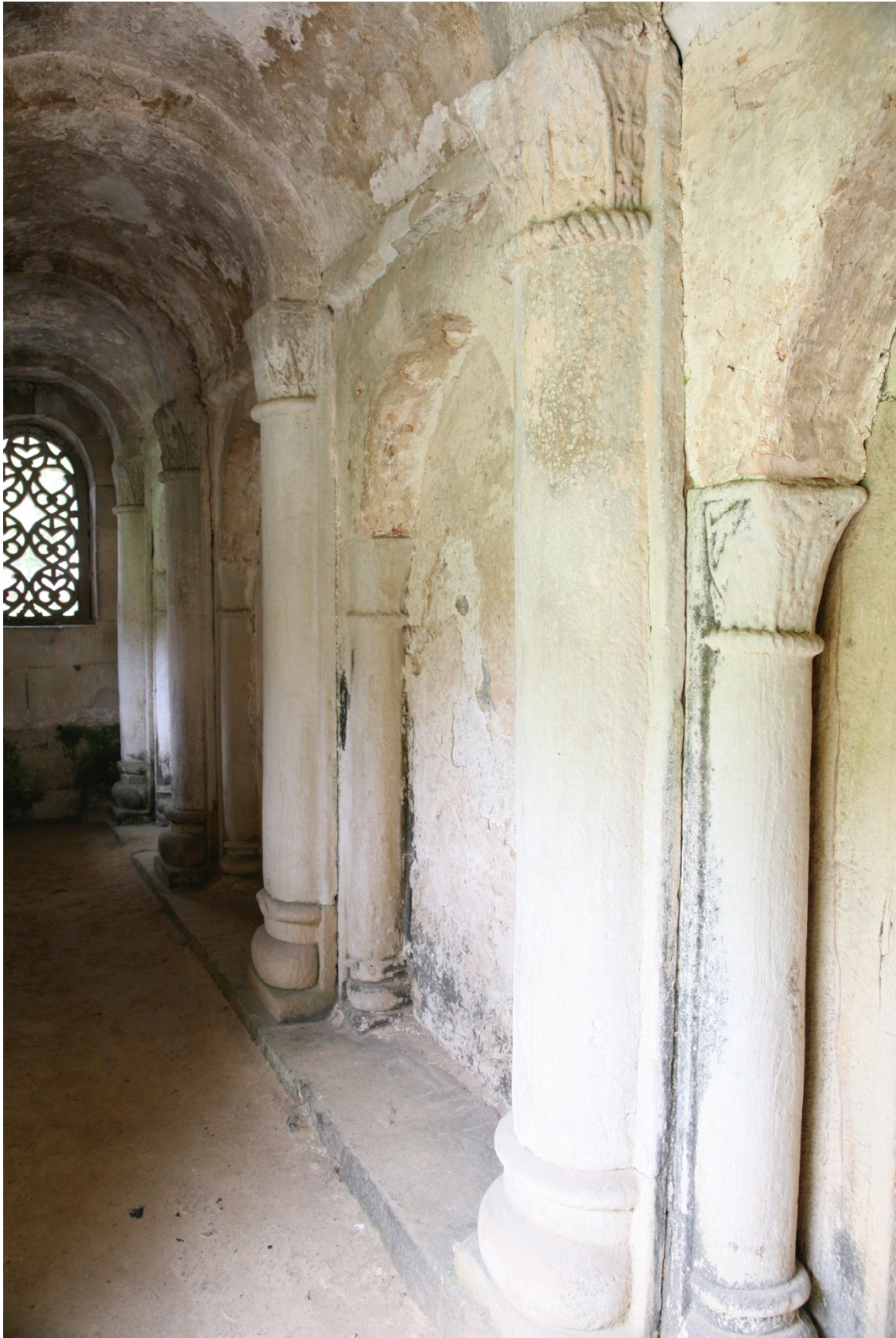
Figure 25.6: San Salvador de Valdediós, Asturias, detail, blind arcade, south porch.
