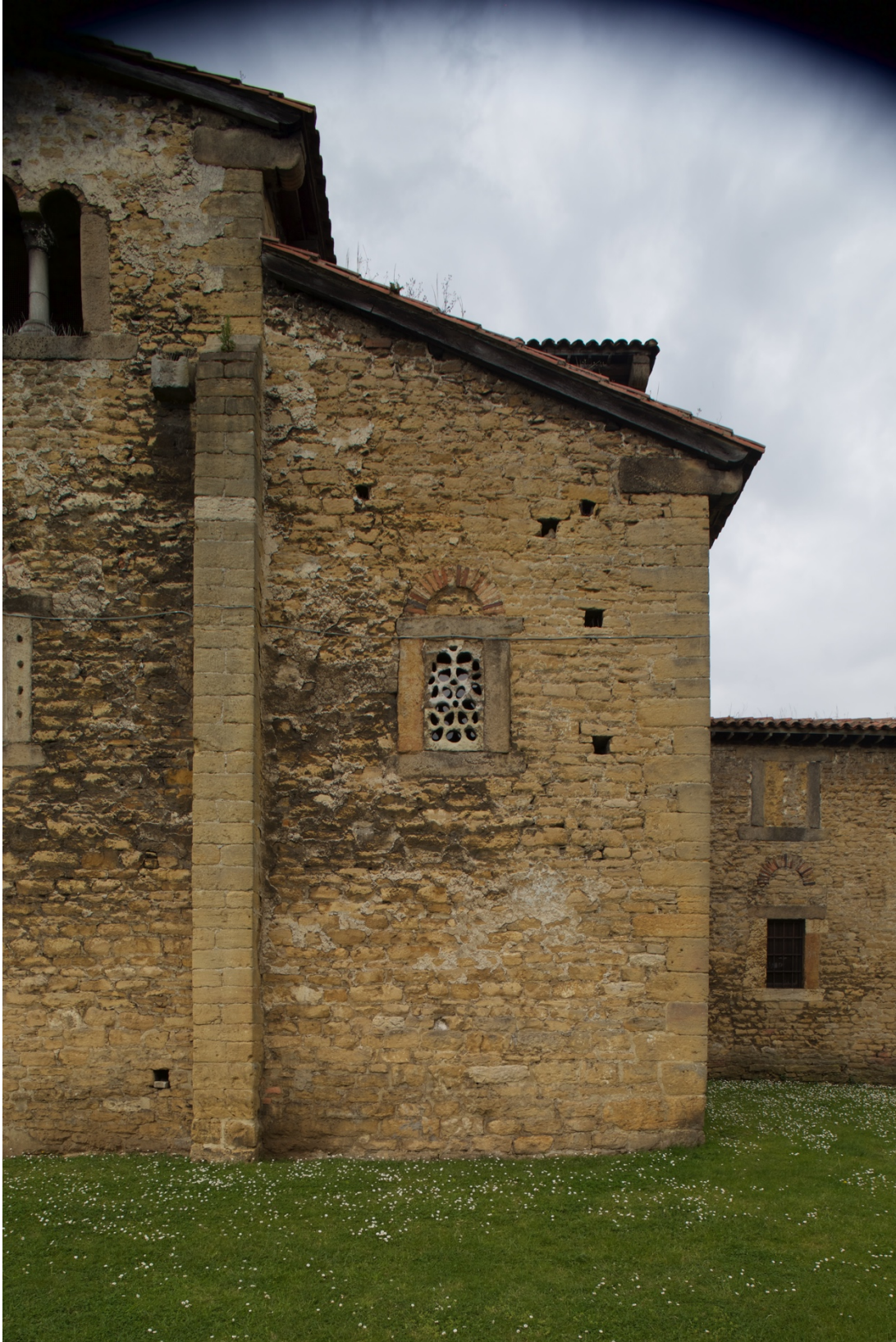
Figure 30.5: San Julián de los Prados, Asturias, exterior east wall, north chapel.
