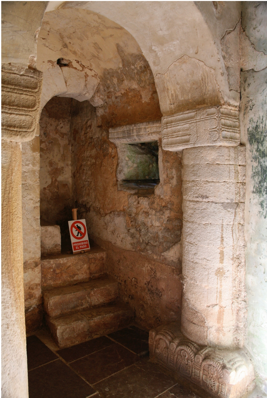
Figure 21.8: San Miguel de Lillo, Asturias, north staircase.
