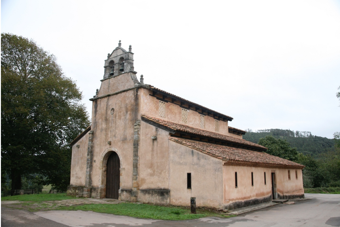
Figure 27: San Salvador de Priesca, Asturias, west façade from south west angle.
