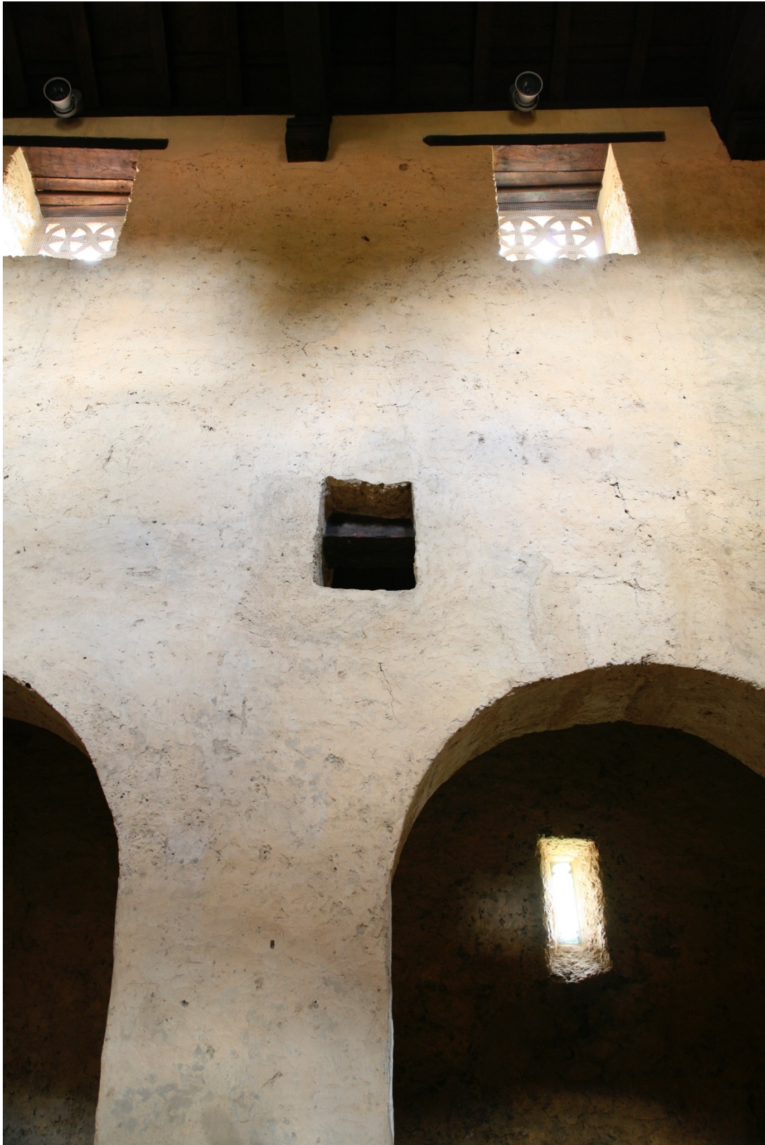
Figure 26.10: San Adriano de Tuñón, Asturias, detail, putlog hole, south nave architrave towards west.
