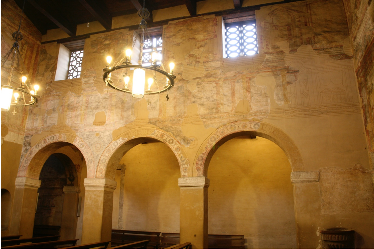
Figure 30.16: San Julián de los Prados, Asturias, south nave arcade.
