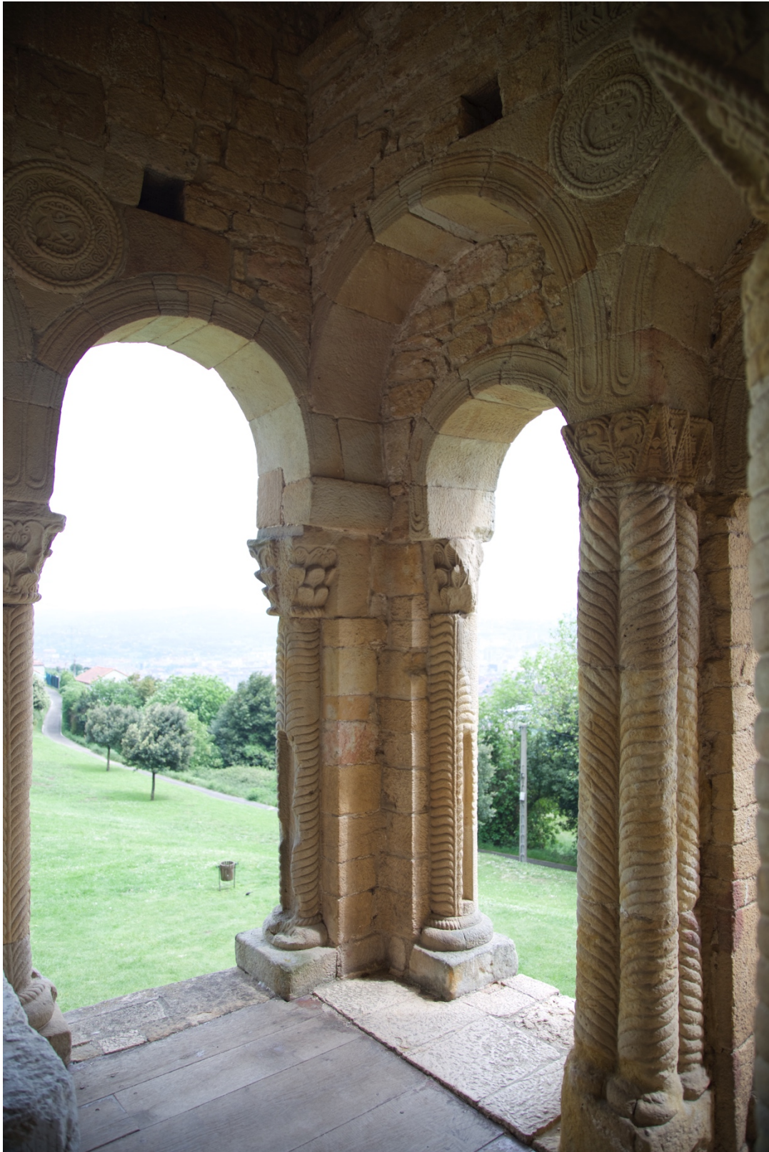
Figure 20.23: Santa María de Naranco, Asturias, supports with incisions for screens, south east angle, east atrium, piano nobile .
