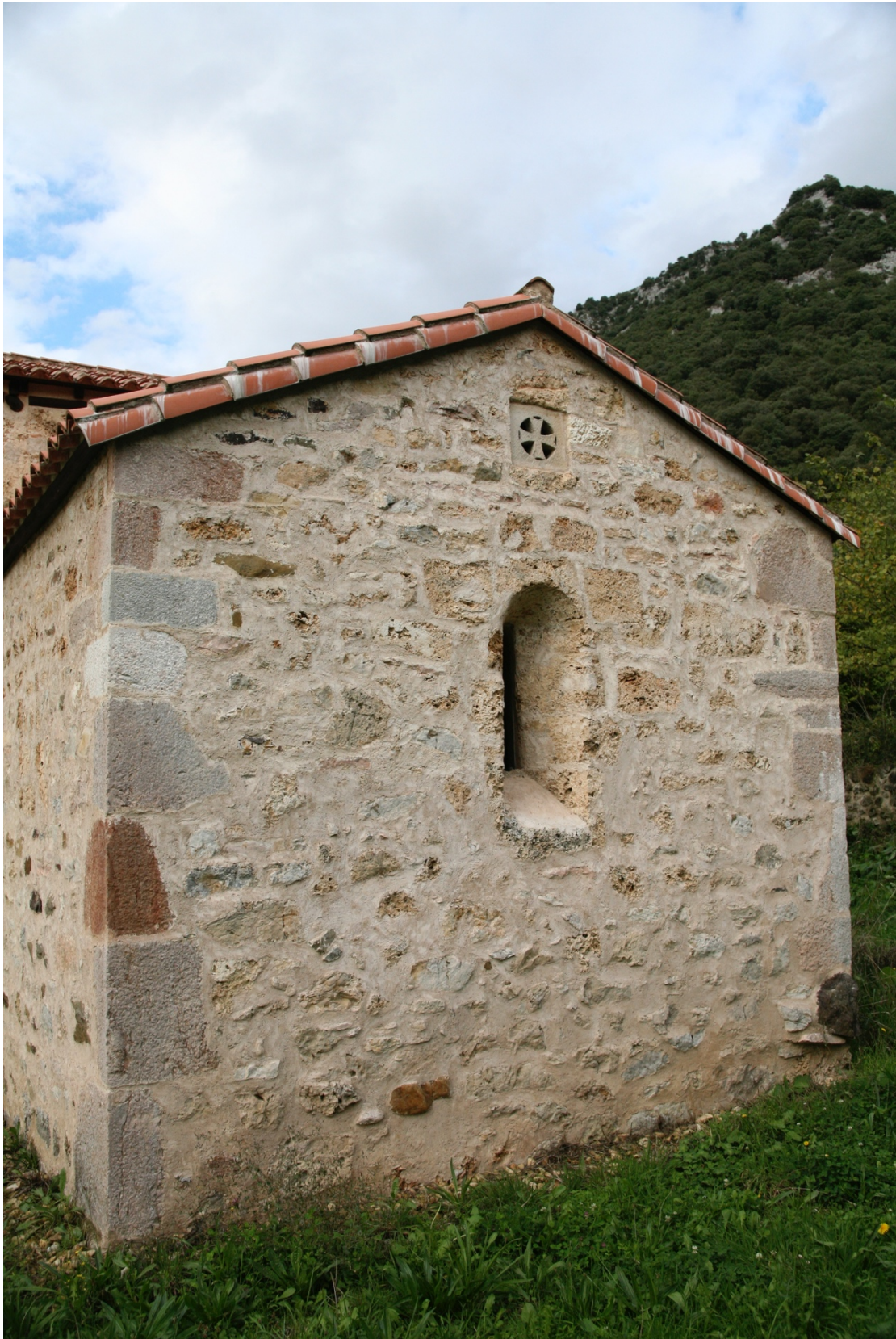
Figure 26.3: San Adriano de Tuñón, Asturias, south wall, south porticus.
