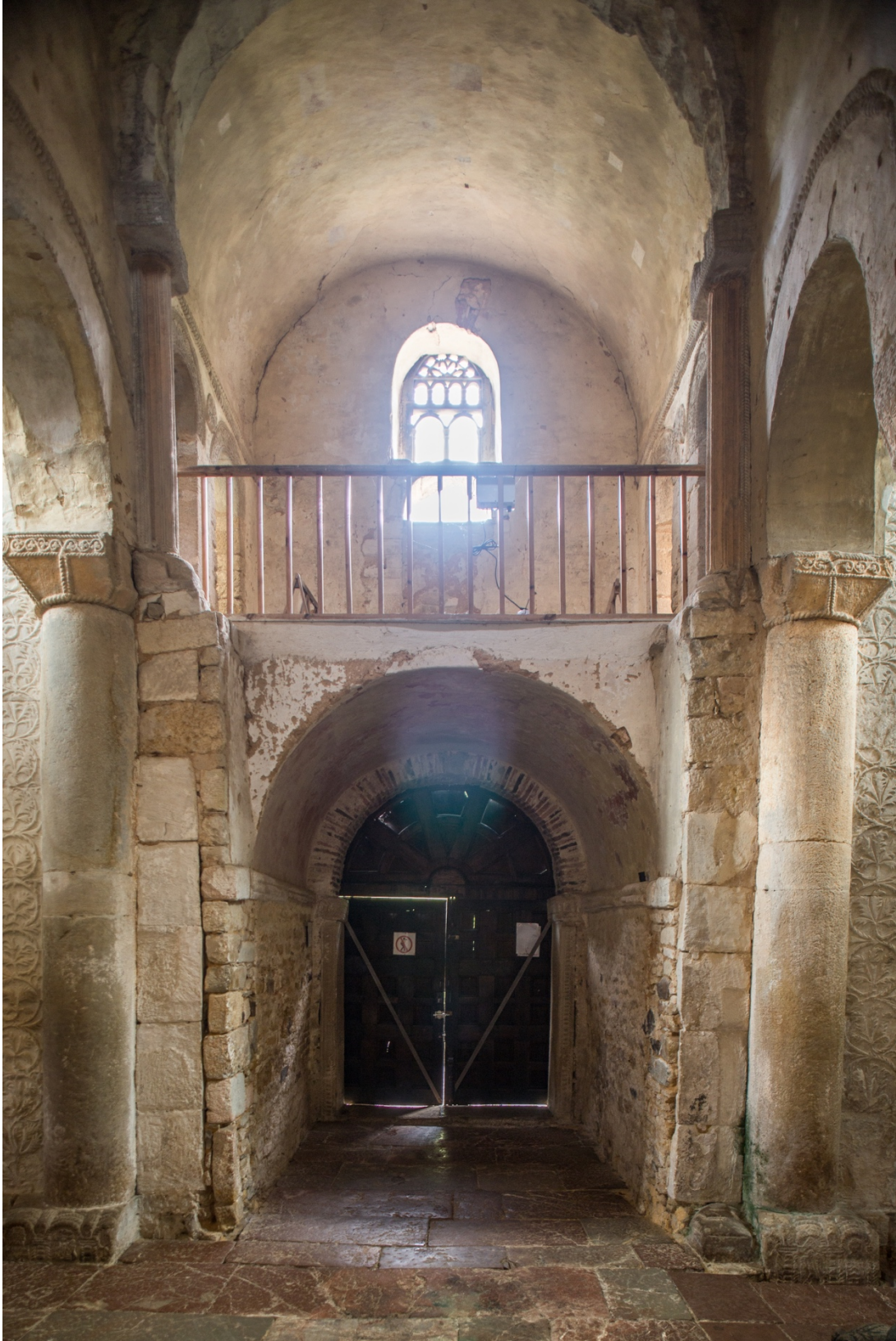
Figure 21.7: San Miguel de Lillo, Asturias, interior west portal barrel vault and tribune.
