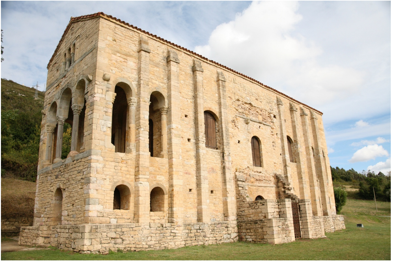
Figure 20.5: Santa María de Naranco, Asturias, south façade from south west angle.
