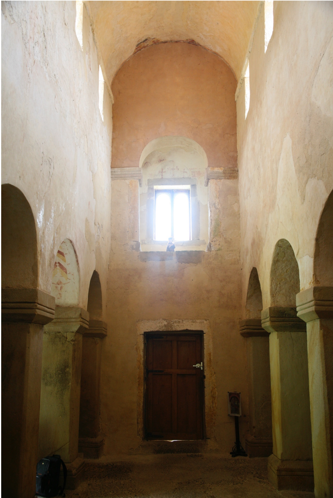
Figure 25.17: San Salvador de Valdediós, Asturias, nave looking west towards tribune.
