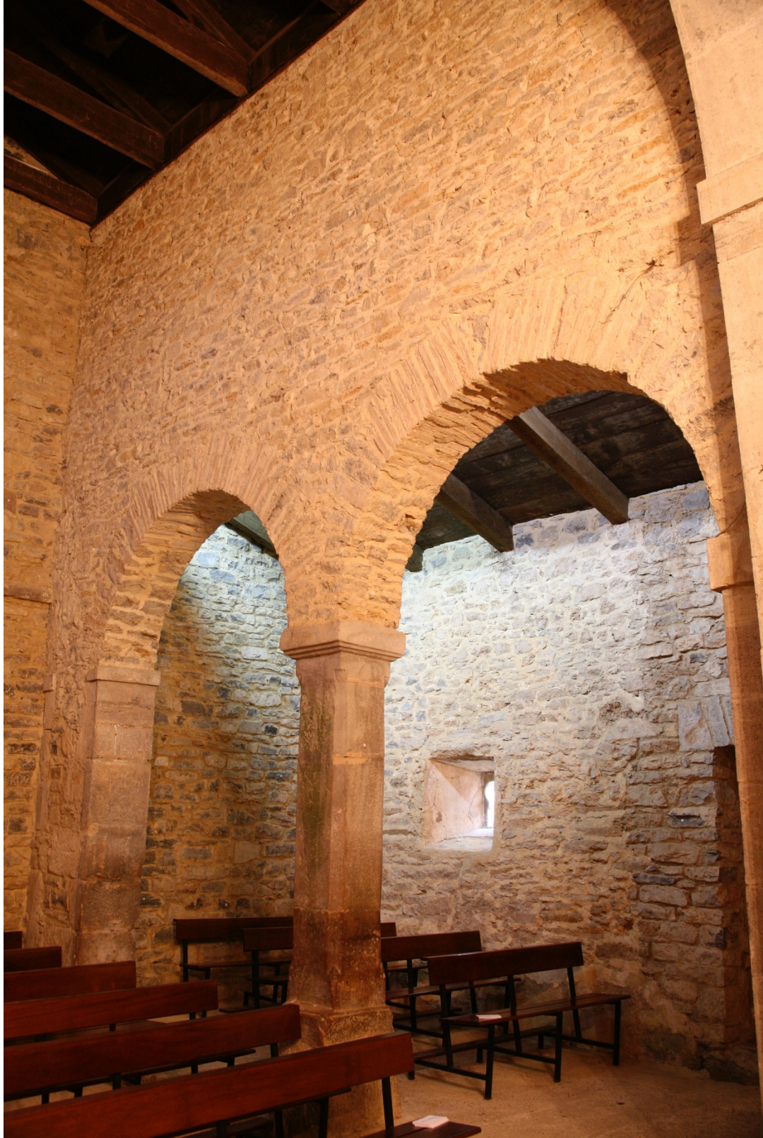
Figure 11.4: Santianes de Pravia, Asturias, south nave arcade looking west.
