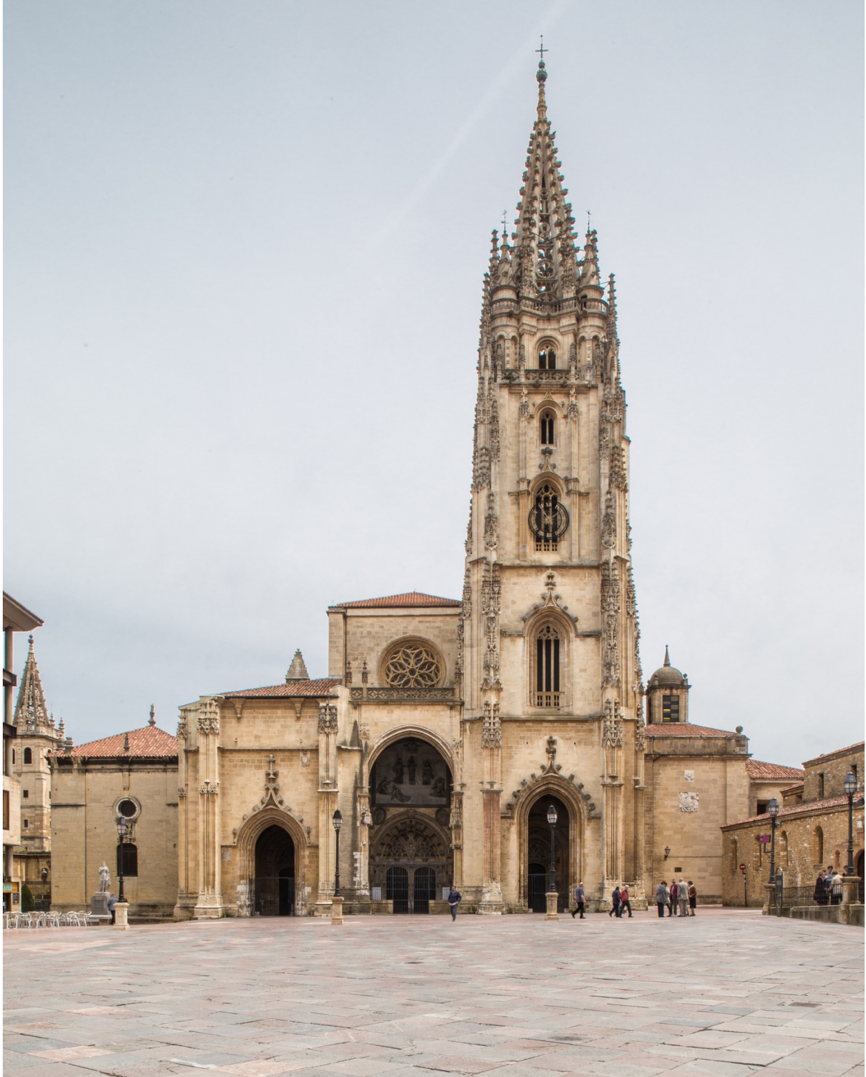
Figure 13: Cathedral of Oviedo, Asturias, west façade.
