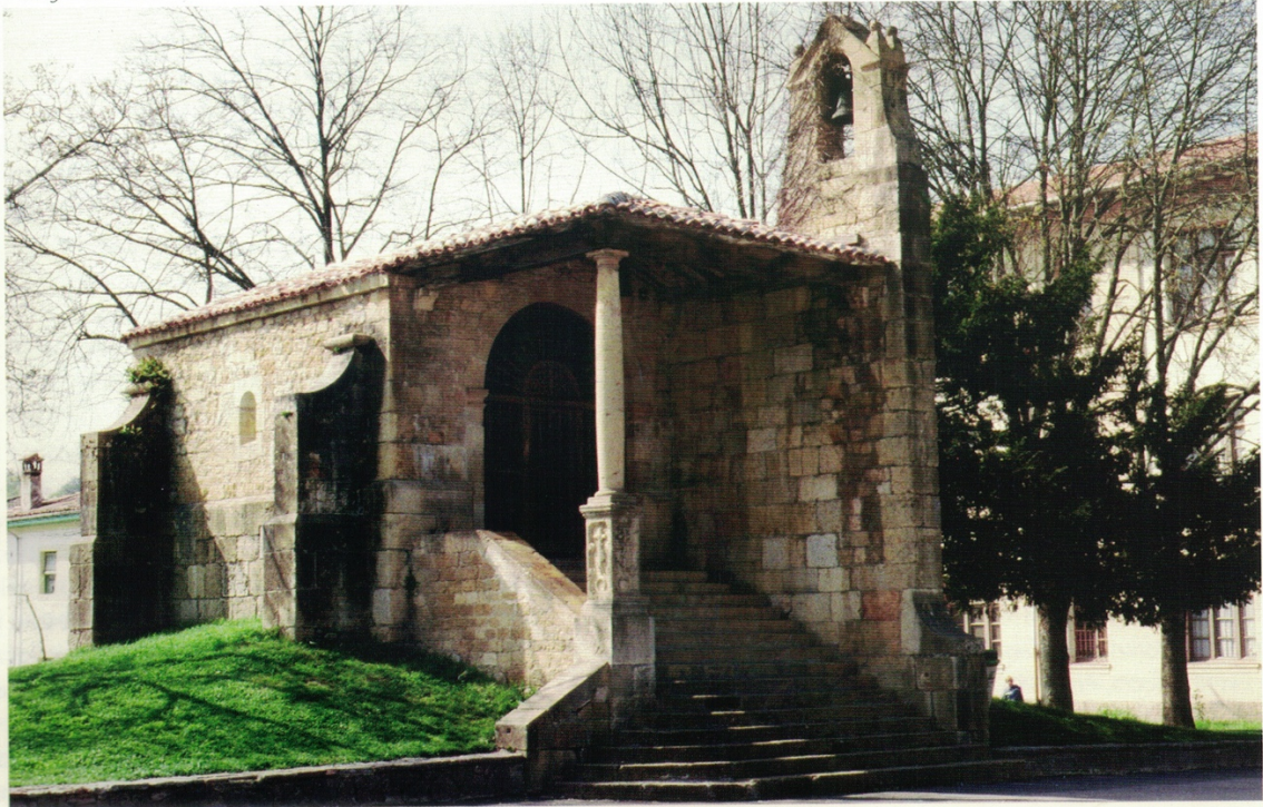
Figure 9: Santa Cruz, Asturias, exterior, west façade from north west angle. After Arias, Encyclopedia , 139.
