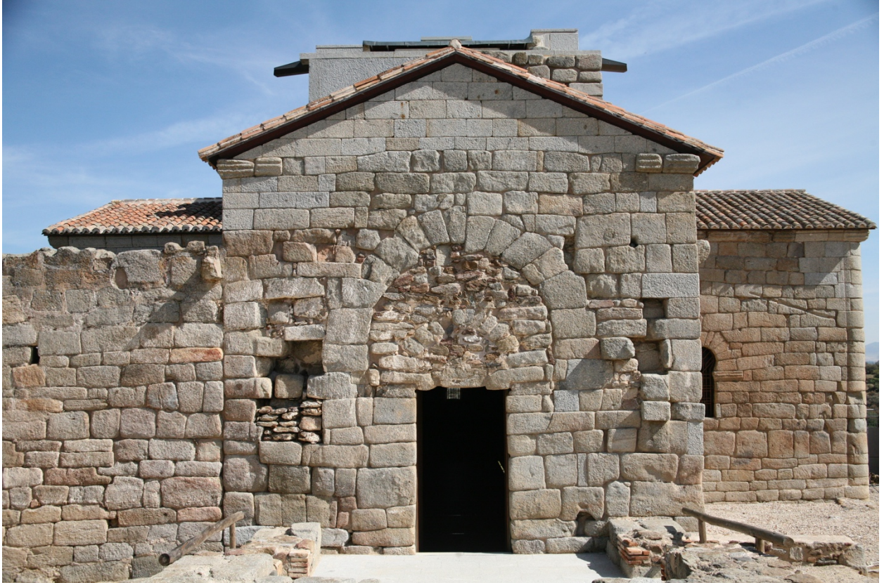
Figure 2.2: Santa María de Melque, Toledo, trabeated arched-portal with pediment, west façade.
