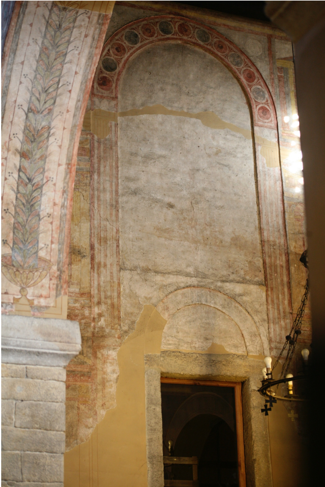
Figure 30.43: San Julián de los Prados, Asturias, detail, upper portal and filled-in arched window, north transept wall.
