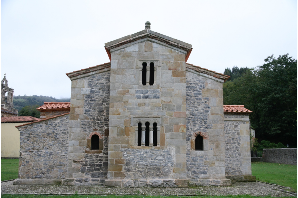
Figure 25.14: San Salvador de Valdediós, Asturias, east façade.
