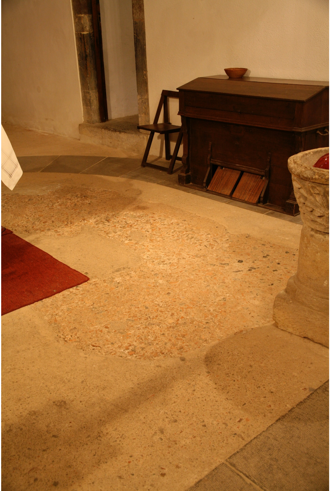
Figure 11.6: Santianes de Pravia, Asturias, detail, eastern apsidal foundation opus signinum .
