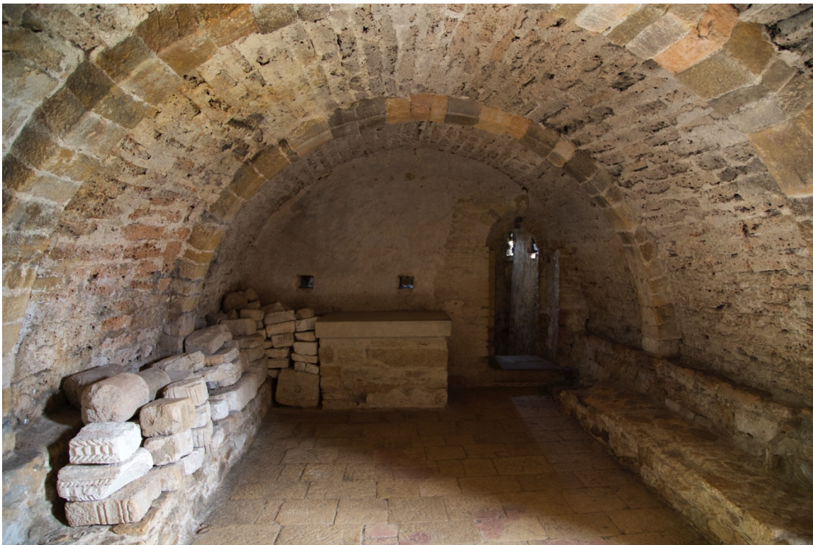
Figure 20.13: Santa María de Naranco, Asturias, undercroft looking east.
