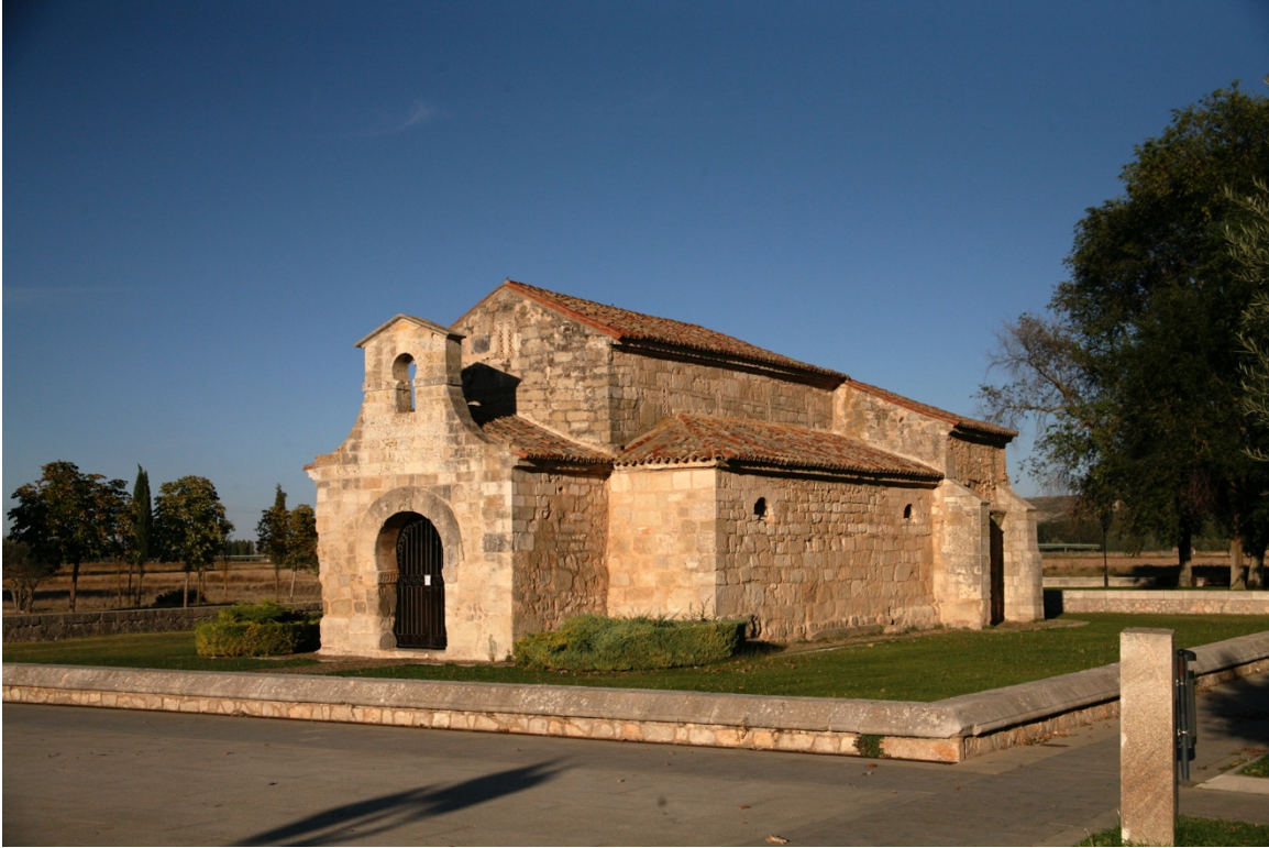
Figure 28: San Juan de Baños, Palencia, west façade from south west angle.
