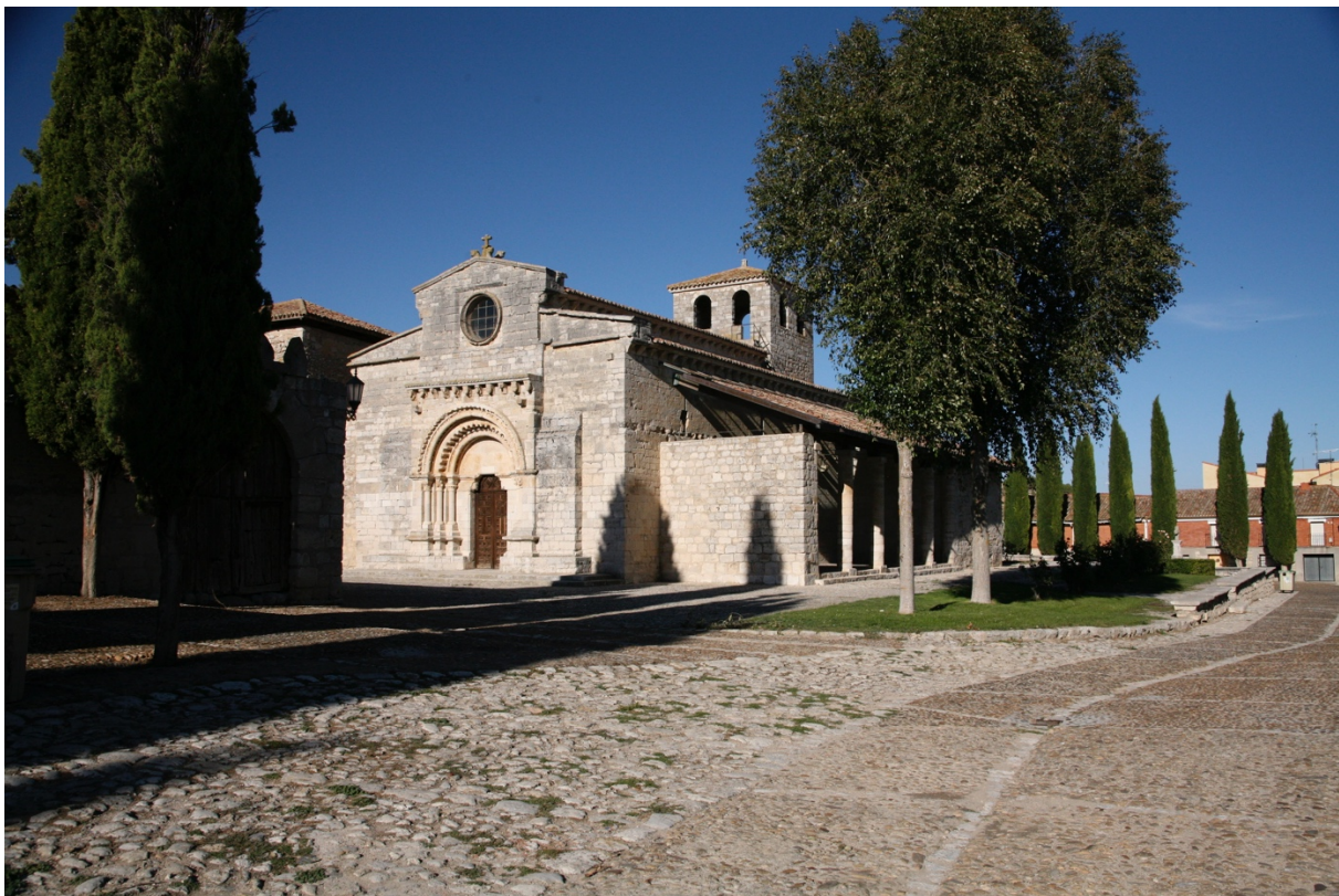
Figure 1.5: Santa María de Wamba, Valladolid, west façade from south west angle.
