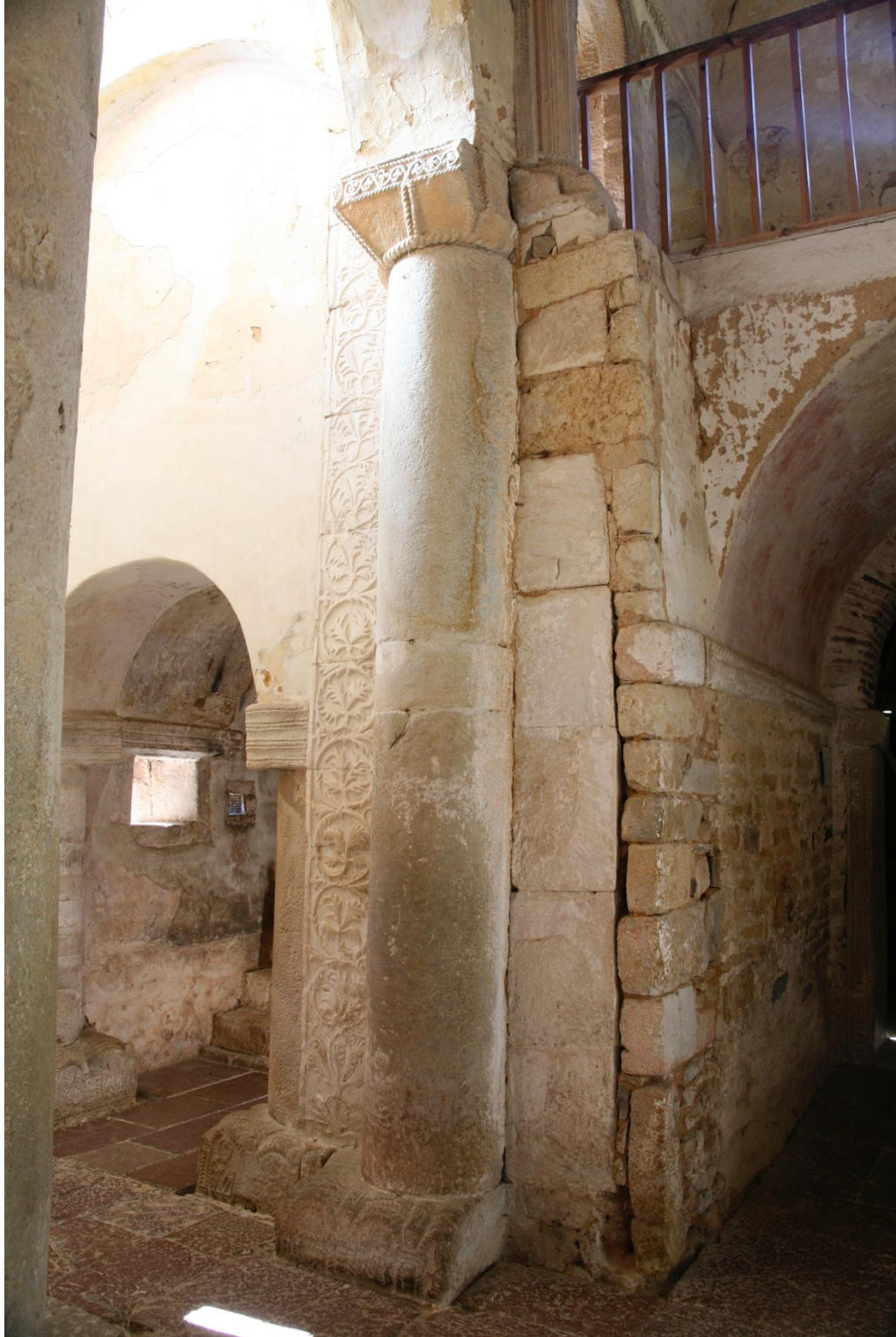
Figure 21.17: San Miguel de Lillo, Asturias, engaged column and pilaster, south nave arcade support.
