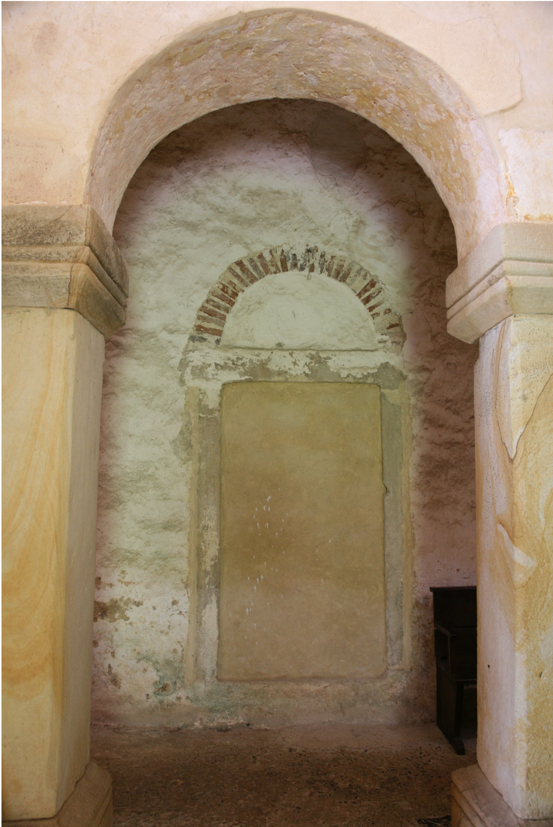
Figure 25.8: San Salvador de Valdediós, Asturias, north west aisle portal.
