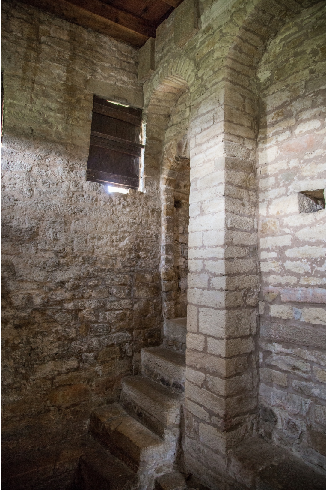
Figure 20.14: Santa María de Naranco, Asturias, doorway leading to subterranean bath in the east end of undercroft.
