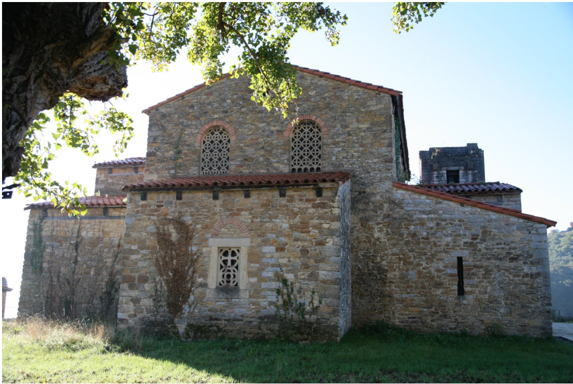
Figure 18.7: Santa María de Bendones, Asturias, north façade with porticus.
