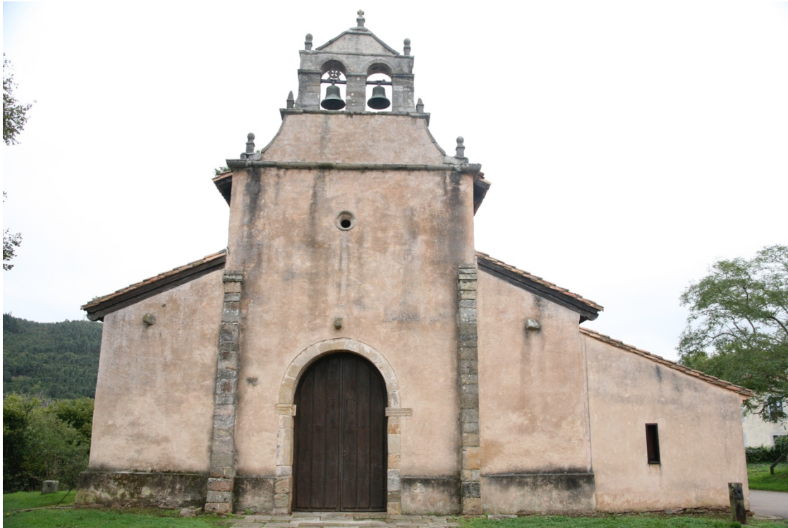
Figure 27.2: San Salvador de Priesca, Asturias, west façade.
