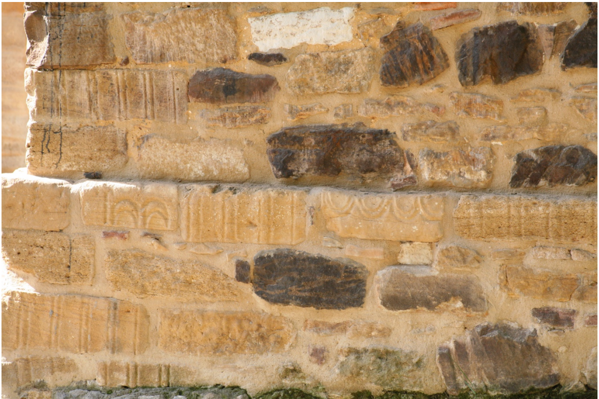
Figure 21.6: San Miguel de Lillo, Asturias, detail, reused masonry in eastern chancel wall.
