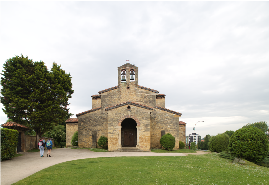
Figure 30: San Julián de los Prados, Asturias, west façade.
