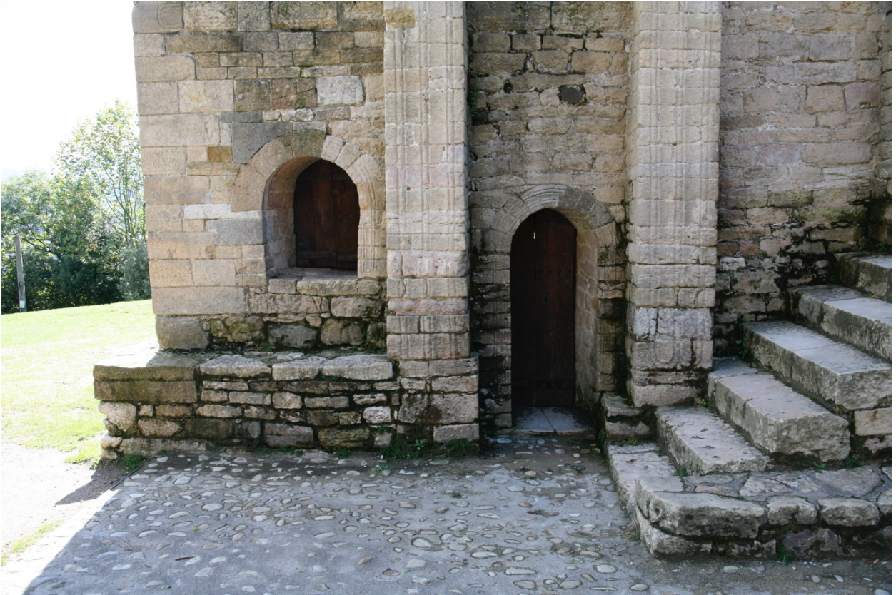
Figure 20.15: Santa María de Naranco, Asturias, detail, portal leading to bath, north façade wall.
