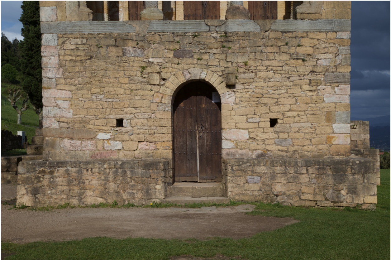
Figure 20.7: Santa María de Naranco, Asturias, detail, ground-level portal, west façade.
