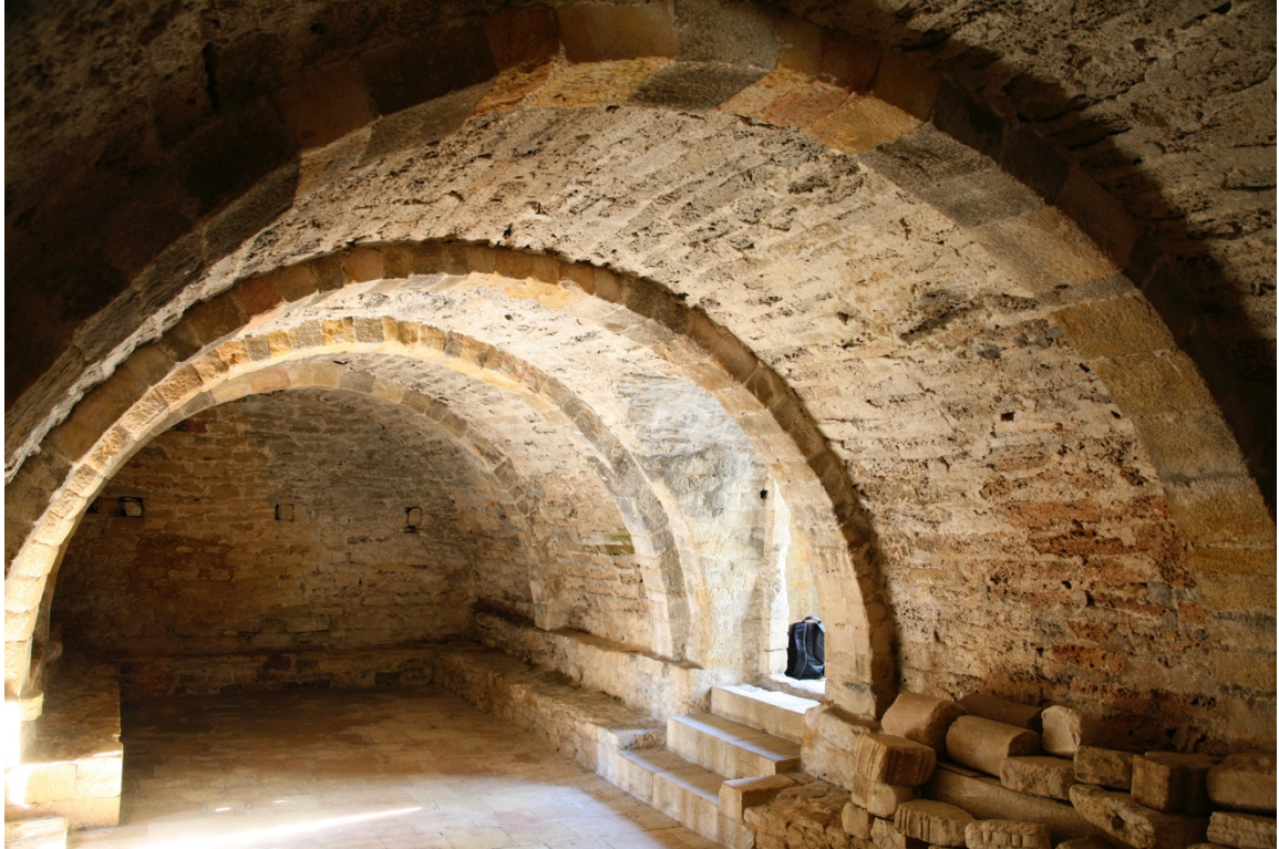
Figure 20.12: Santa María de Naranco, Asturias, undercroft looking west.
