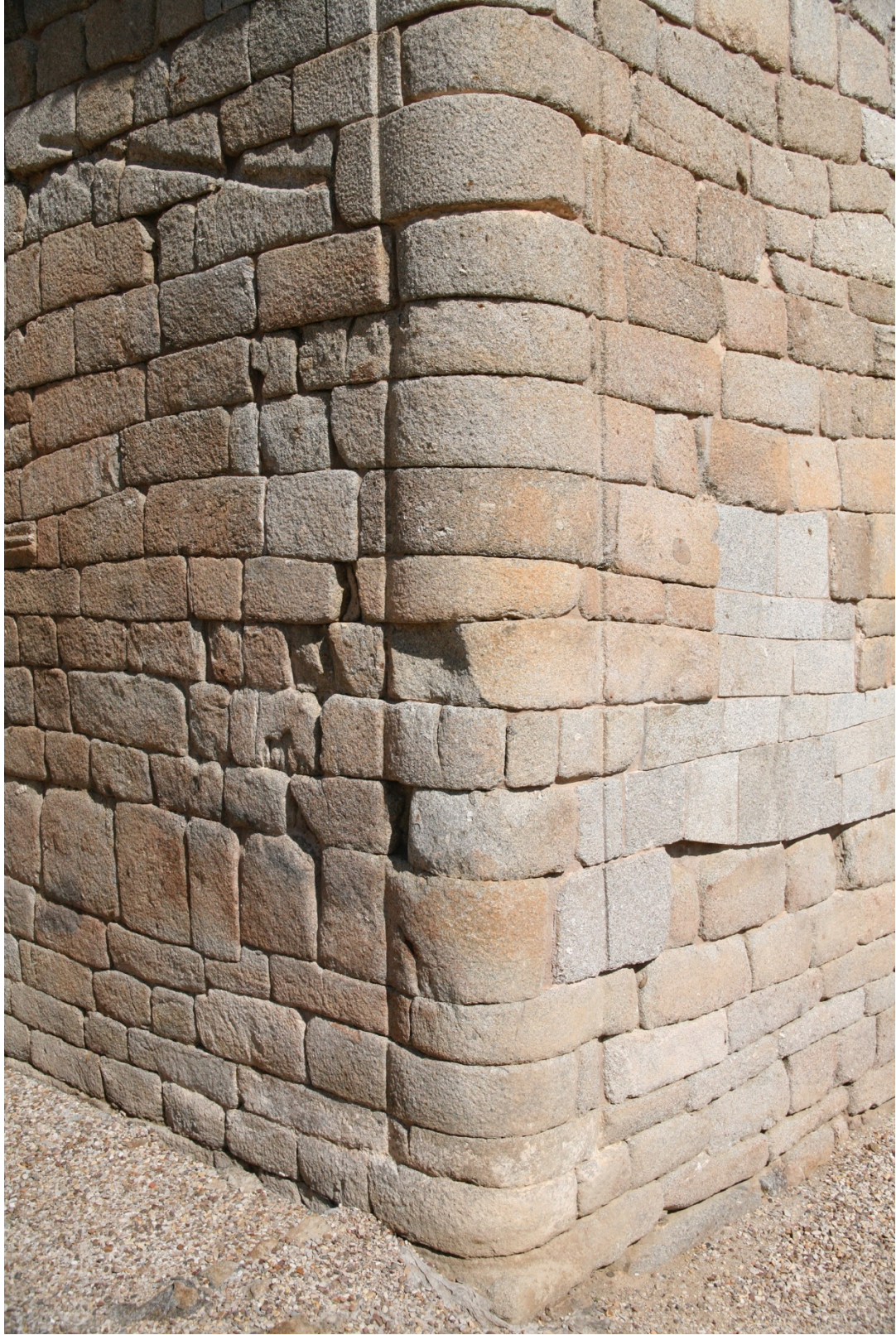
Figure 2.1: Santa María de Melque, Toledo, detail, rounded exterior quoin, south west angle of south transept.
