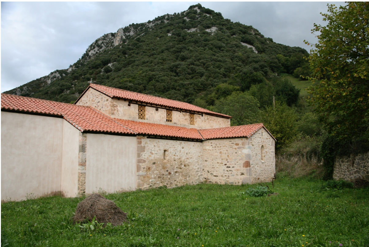
Figure 26: San Adriano de Tuñón, Asturias, south façade from south west angle.
