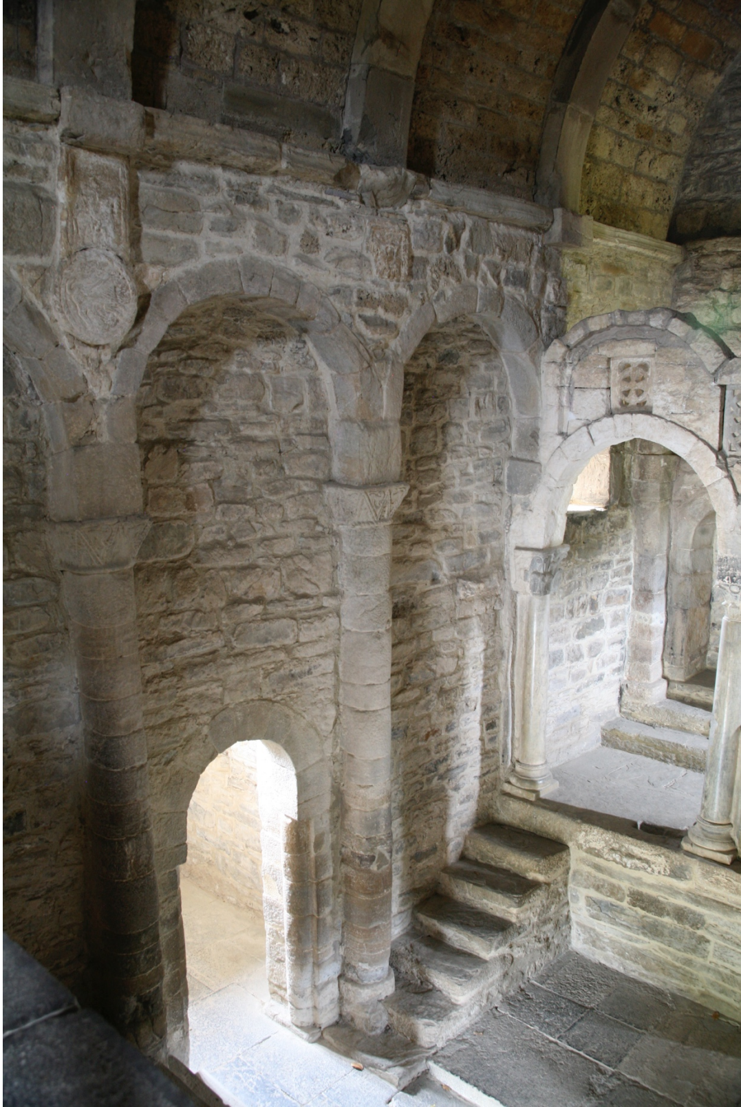
Figure 22.8: Santa Cristina de Lena, Asturias, north nave blind arcade looking east from tribune.
