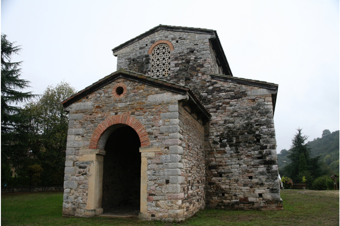
Figure 19: San Pedro de Nora, Asturias, west façade from south west angle.
