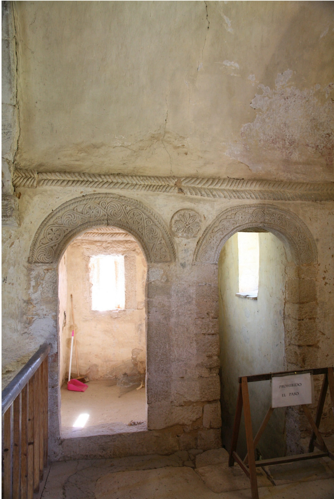
Figure 21.14: San Miguel de Lillo, Asturias, south wall of tribune, showing carved hood mouldings, spandrel roundels, and stringcourse.
