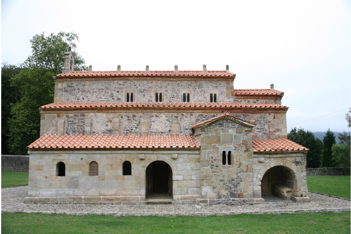
Figure 25.4: San Salvador de Valdediós, Asturias, south façade.
