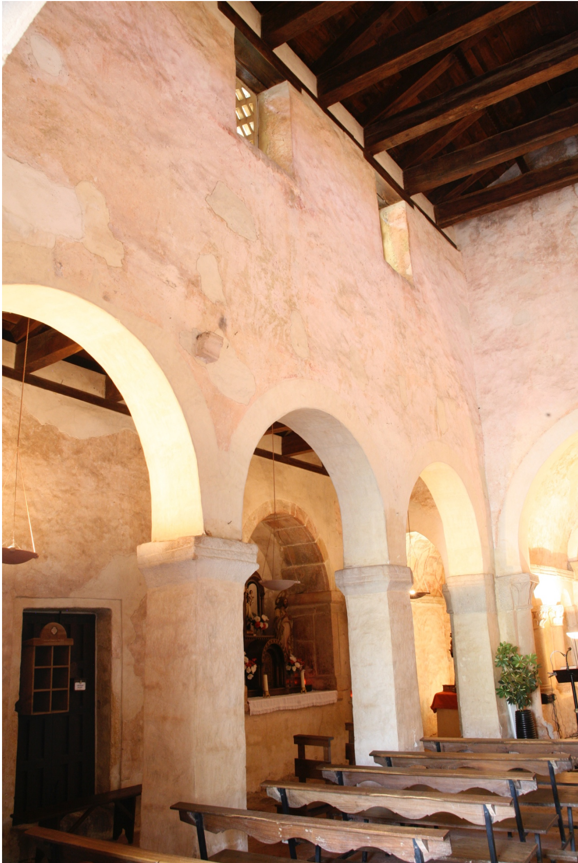
Figure 27.10: San Salvador de Priesca, Asturias, north nave aisle looking east.
