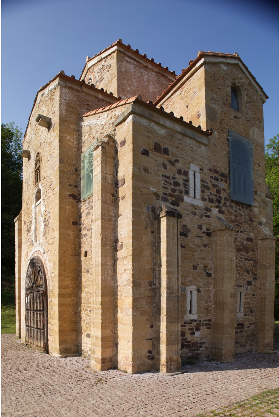
Figure 21.1: San Miguel de Lillo, Asturias, south façade from south west angle.
