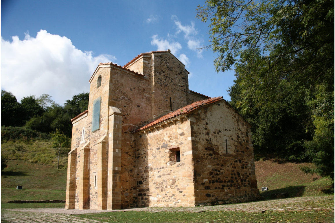
Figure 21.5: San Miguel de Lillo, Asturias, eastern chancel addition from south east angle.
