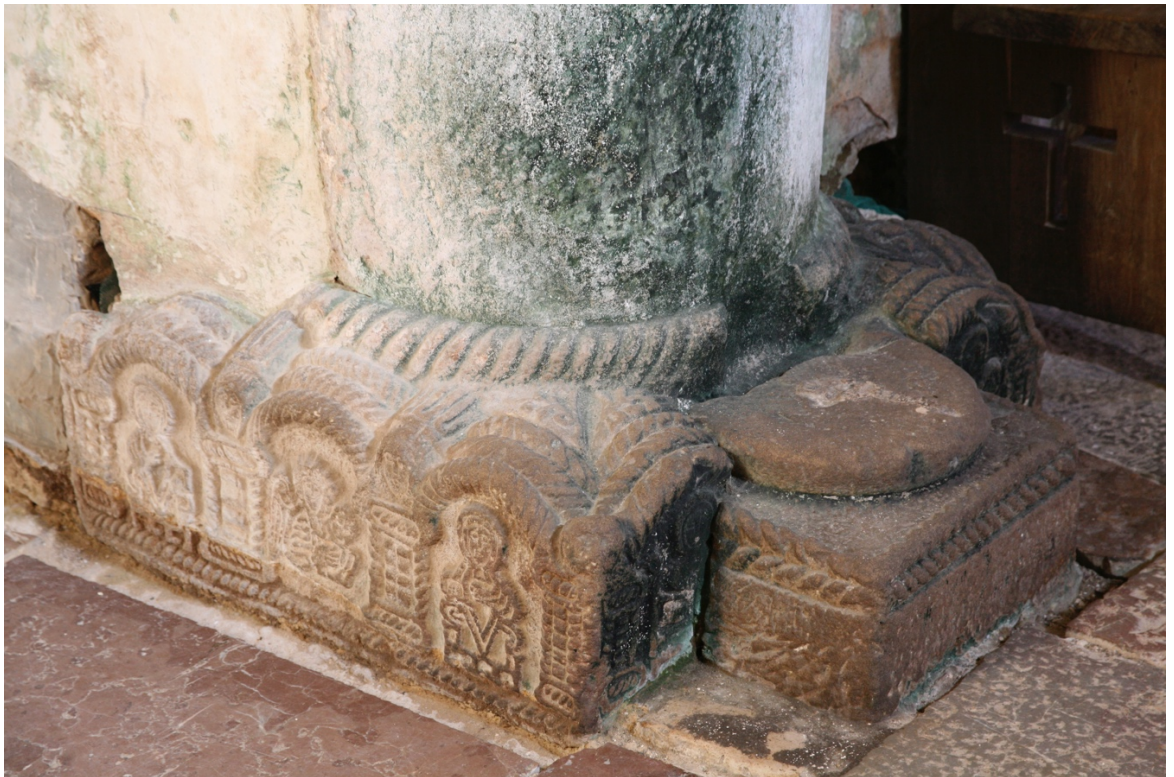
Figure 21.21: San Miguel de Lillo, Asturias, detail, carved base with later addition, north nave arcade support.
