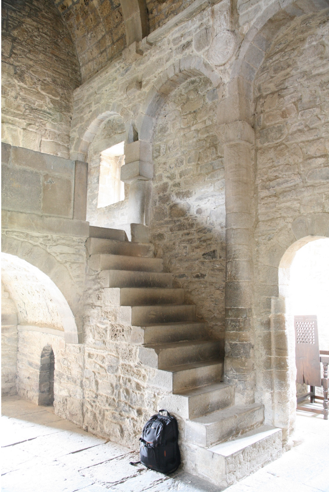
Figure 22.6: Santa Cristina de Lena, Asturias, north staircase leading to tribune.
