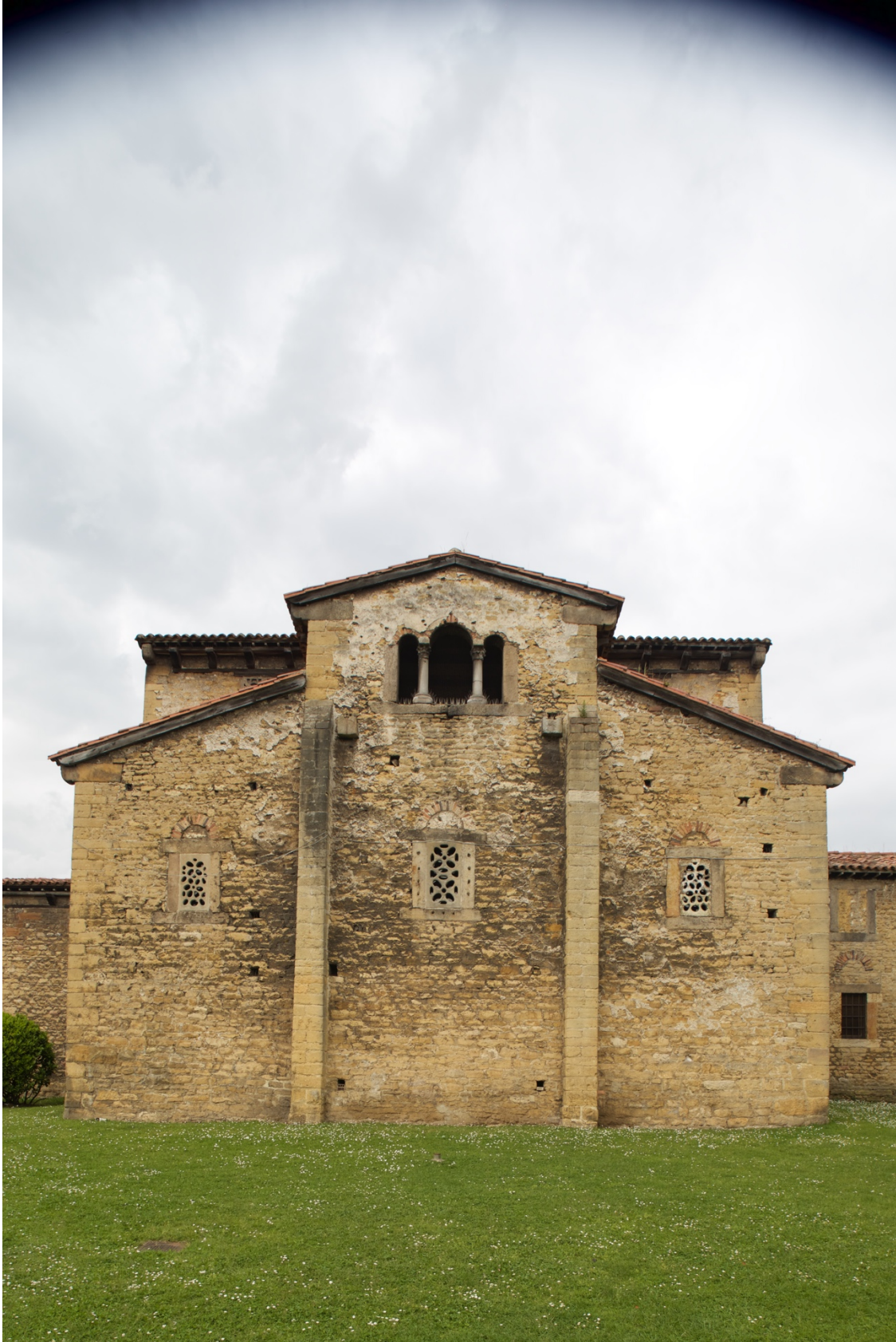
Figure 30.7: San Julián de los Prados, Asturias, east façade.
