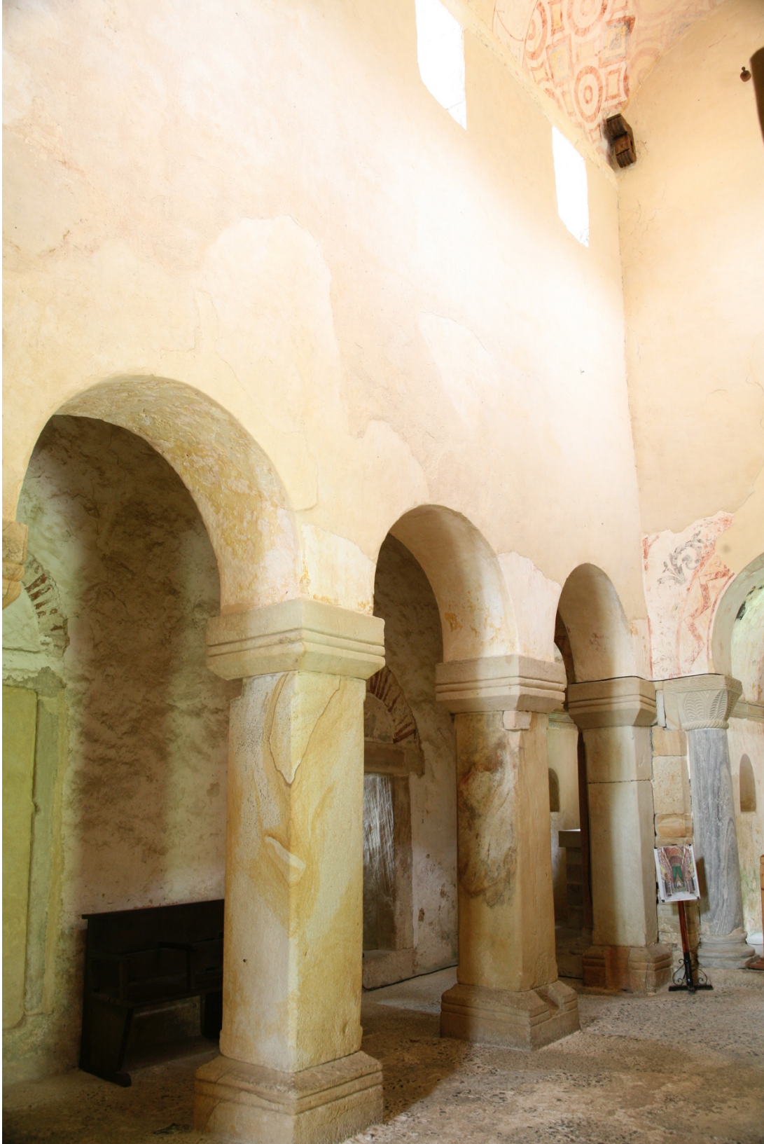
Figure 25.24: San Salvador de Valdediós, Asturias, north nave arcade looking east.
