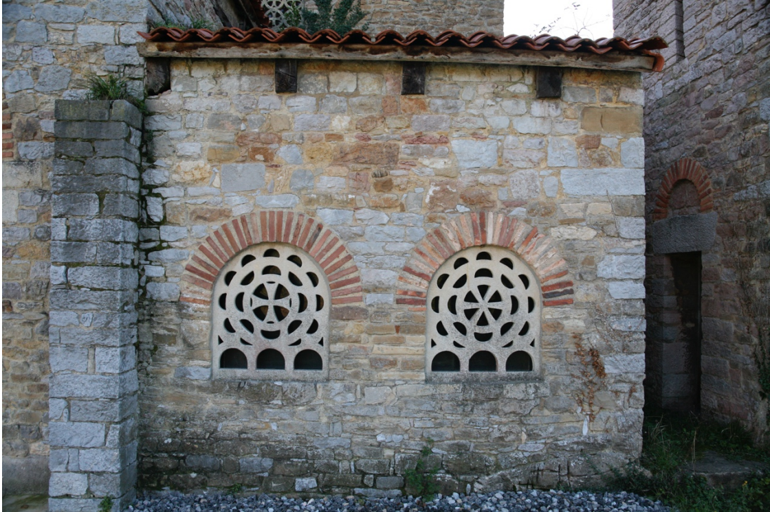
Figure 18.6: Santa María de Bendones, Asturias, round headed windows with red brick arches, south chamber flanking western porch.
