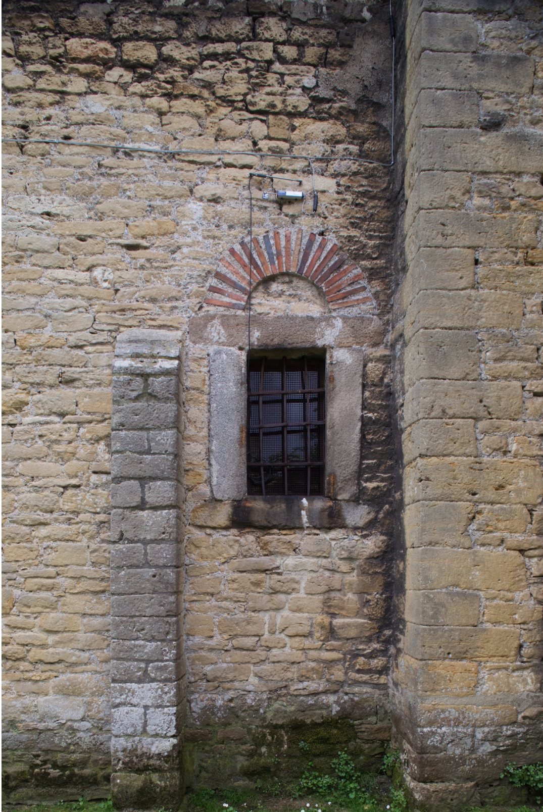
Figure 30.4: San Julián de los Prados, Asturias, trabeated arched-window, north west wall, north chapel.
