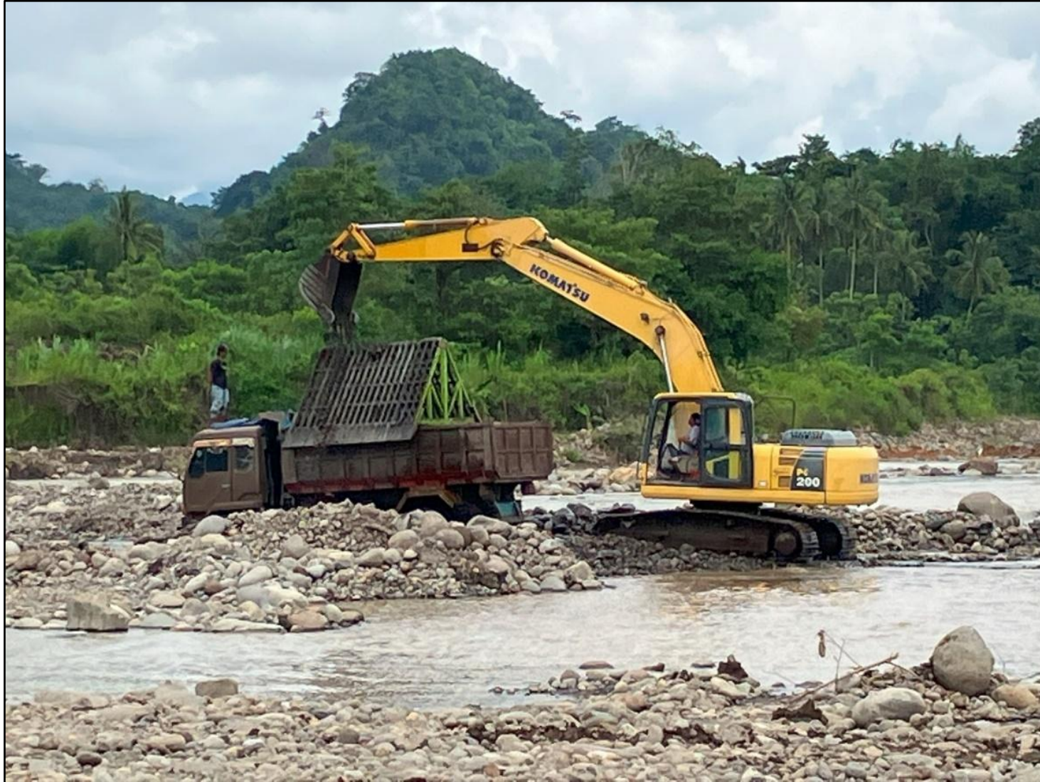
Photo 3.20. Sieving Sand in the Jeneberang River Channel during the rainy season (Kelurahan Lanna, Parangloe, 2022).
