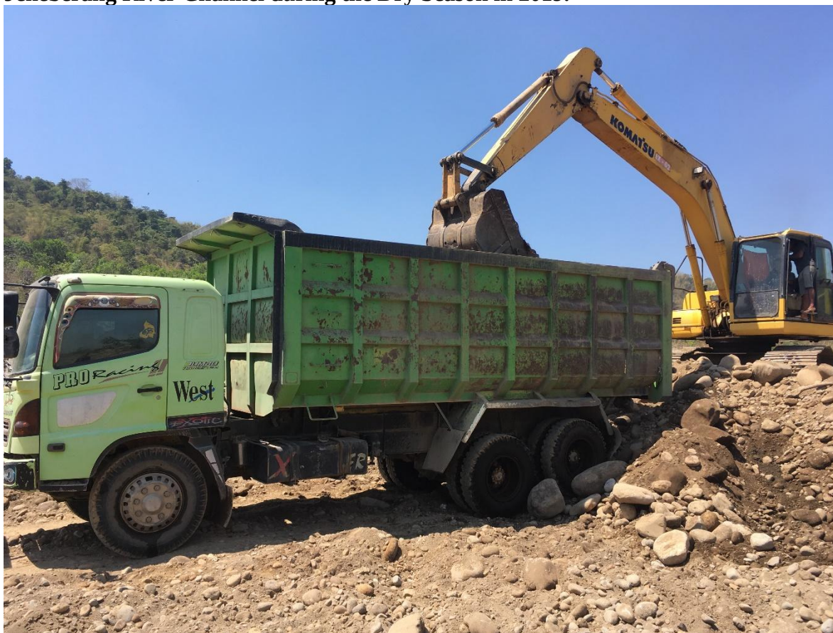
Photo 3.19. A Komat'su excavator removing sand and stone materials from the Jeneberang River Channel during the Dry Season in 2019.
