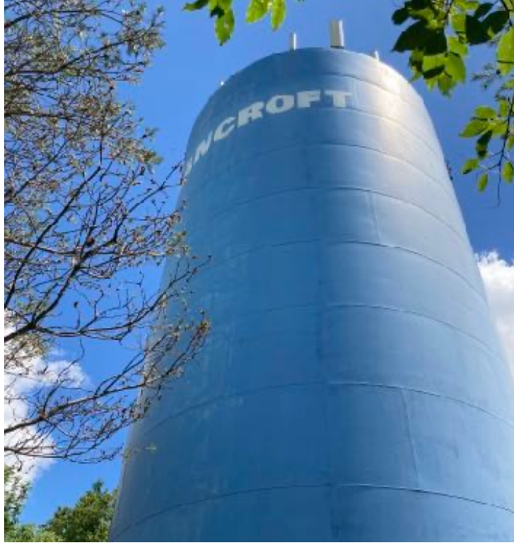
Figure 47: Bancroft Water Tower (Photograph by Author)
