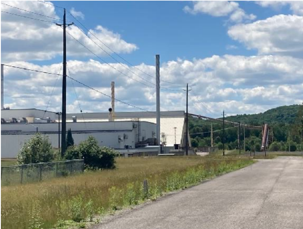
Figure 31: Former Flakeboard Factory, Outside Bancroft (Photograph by Author)
