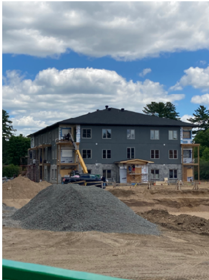
Figure 59: New Development on Old School Site (Photograph by Author)
