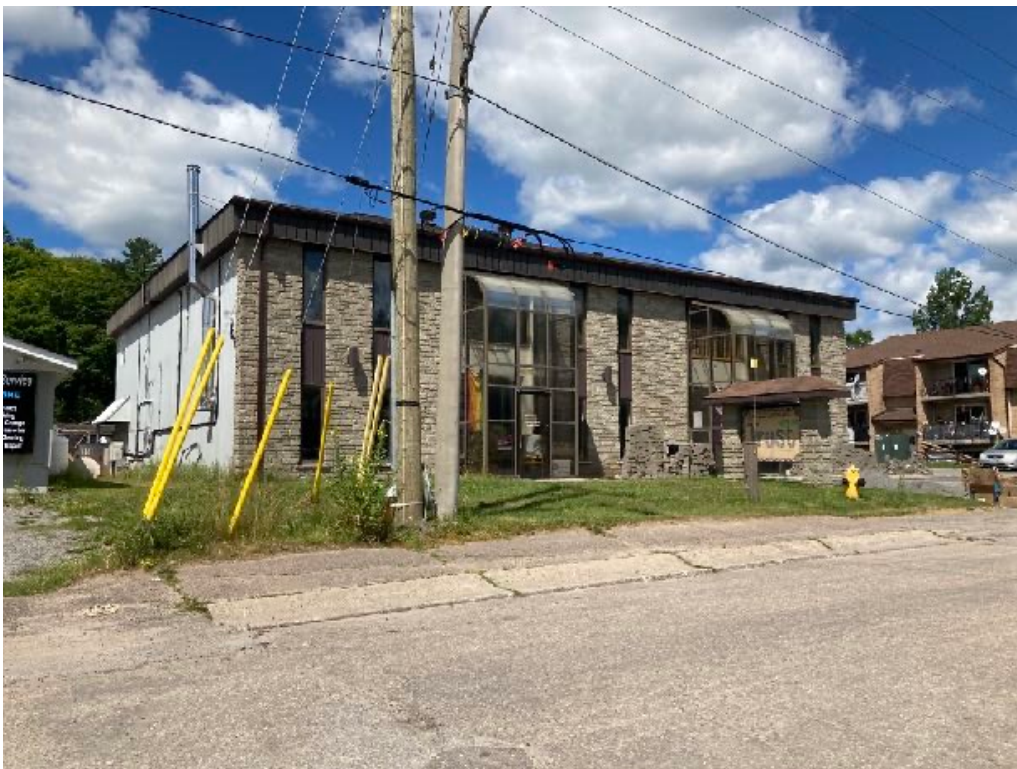
Figure 60: New Home Of NHCT (Photograph by Author)
