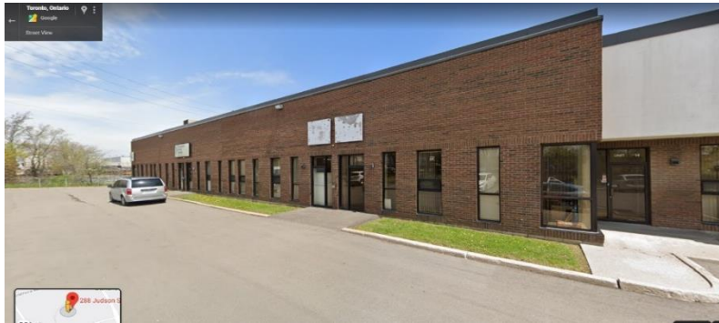
Figure 2: Image of Exterior Community Living SWACA program, 288 Judson Avenue, Unit 17, Retrieved from https://www.google.com/maps/
