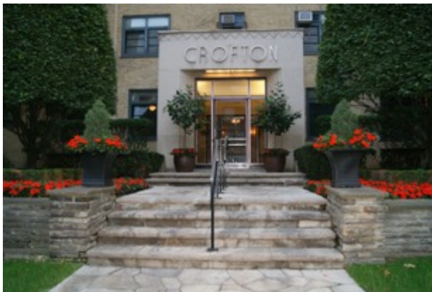
Figure 11. The Crofton condo building
