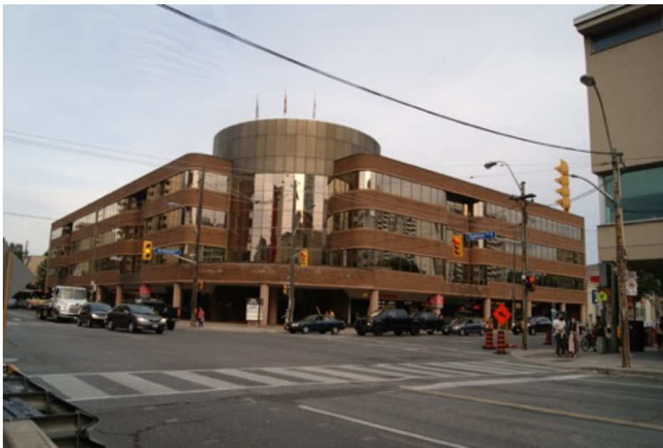
Figure 7. The intersection of Eglinton and Mount Pleasant road
