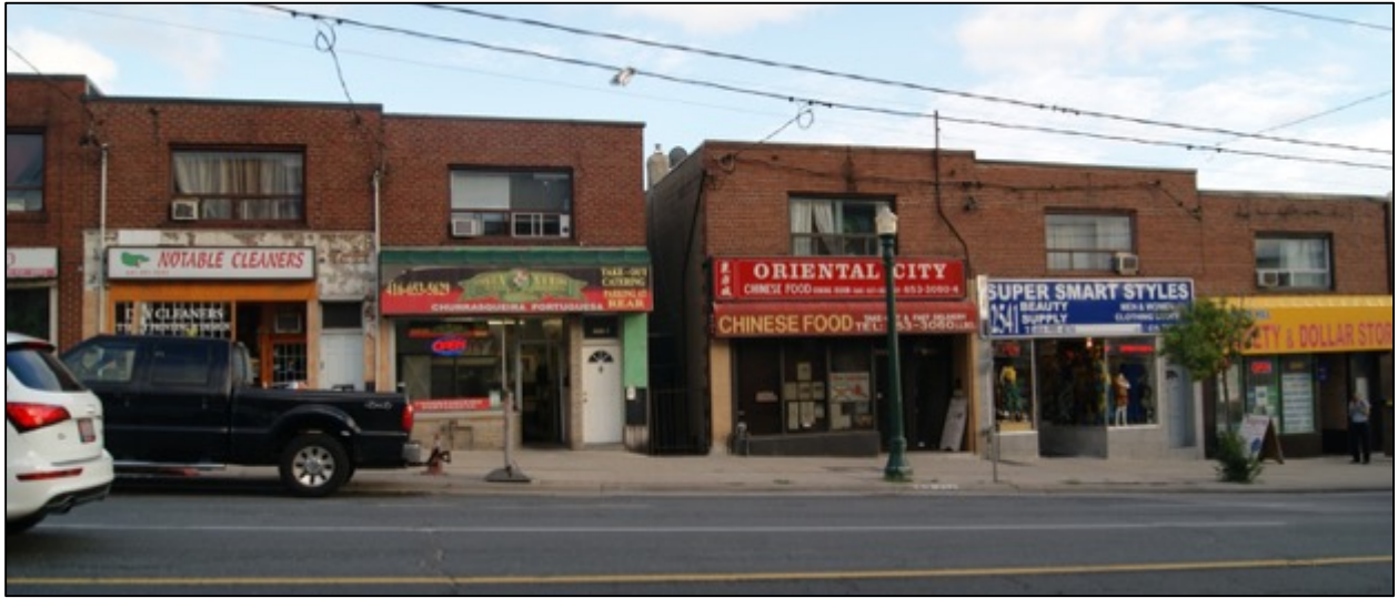
Figure 13. 2-storey developments with local ethnic businesses on the lower level and residential on the second floor
