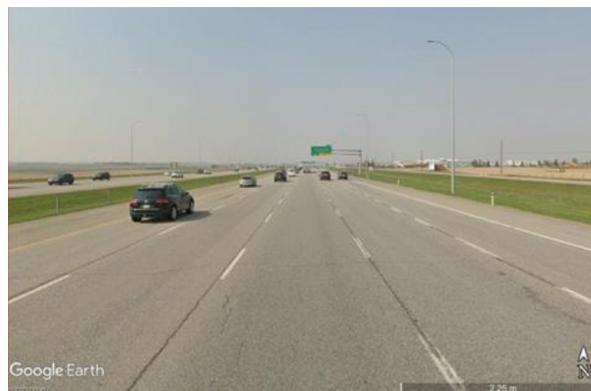
Figure 3.2: A typical divided highway ((a) Vanek, et al. 2014; (b) Highway No.2, in the north of Calgary, AB, Canada: Google Earth 2023)
