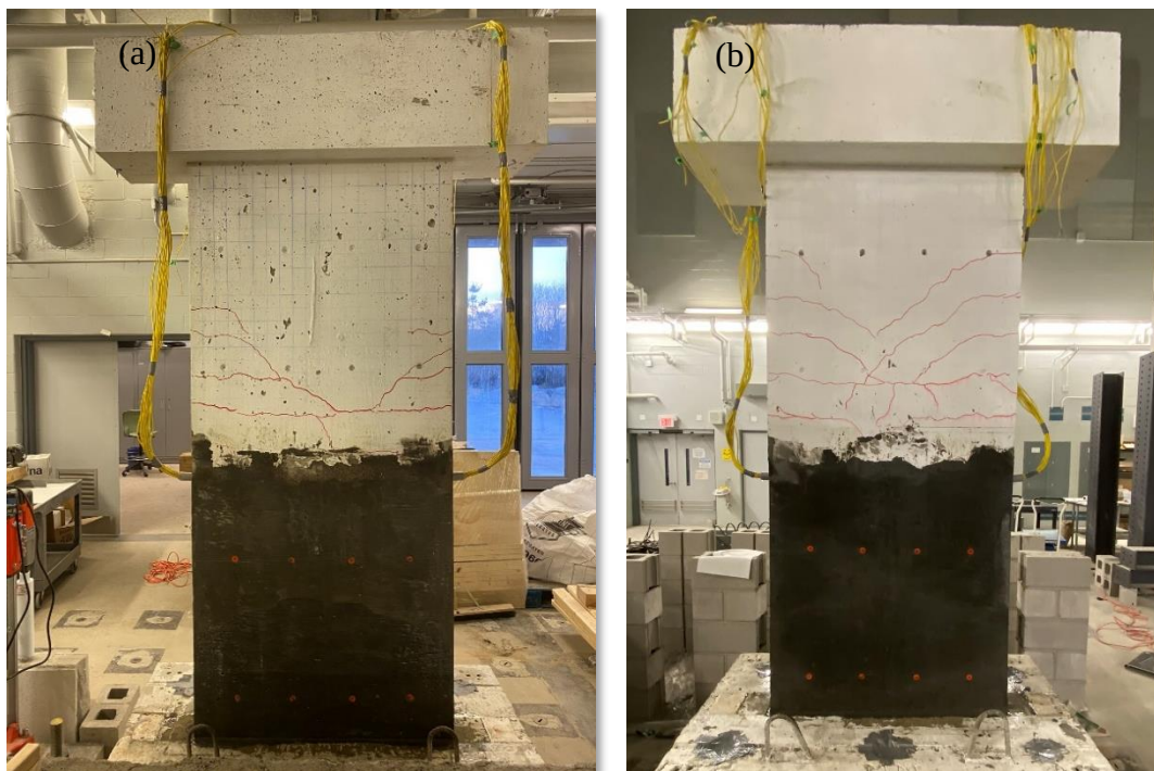
Figure 4.31 Demolding of formwork: (a) Wall SWS-R; and (b) Wall SWN
