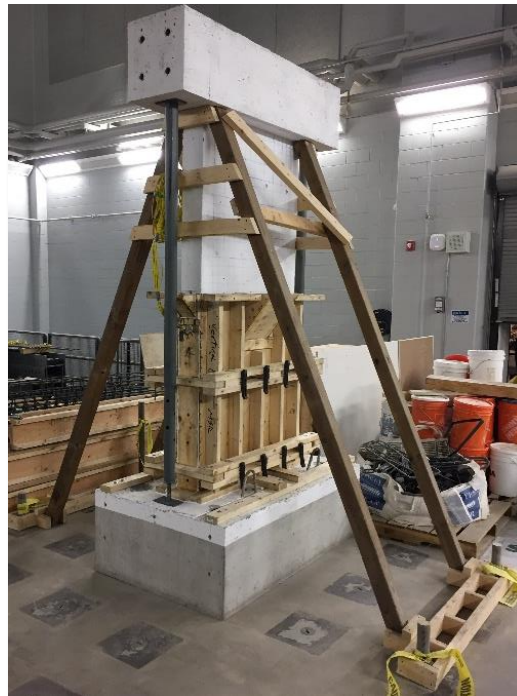
Figure 4.27 Formwork installed on Wall SWN
