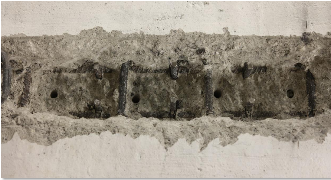
Figure 4.21 Drilled holes for starter bars
