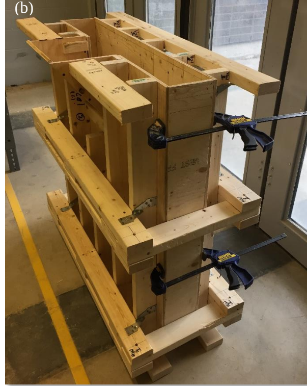
Figure 4.26 Constructed formwork: (a) top view; and (b) side view
