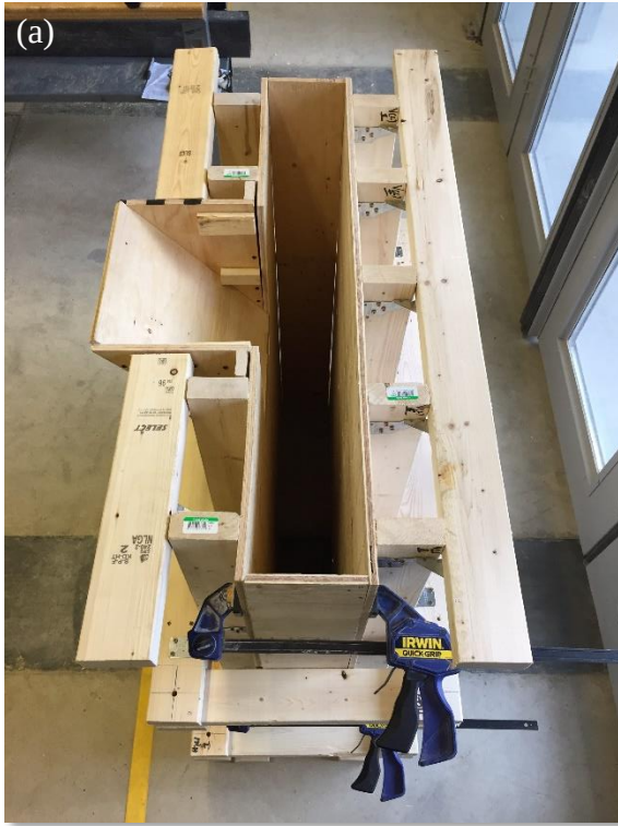
Figure 4.26 Constructed formwork: (a) top view; and (b) side view
