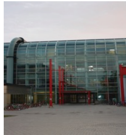
3. University of Waterloo Davis Center Library
