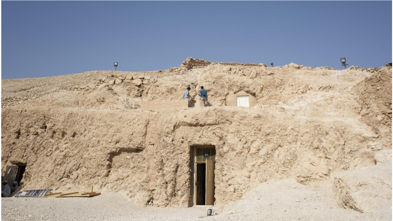
Figure 5: Entrance and facade of TT95. The image highlights the direct exposure of the rock to the climate at the ground surface. The infilled open fracture can be seen to the left of the entrance.
