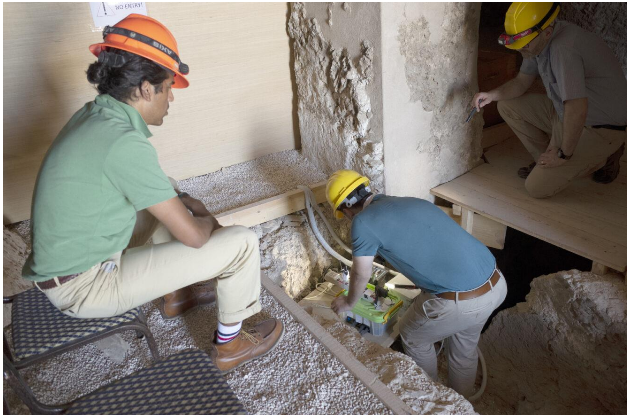
Figure 15: Installation of monitoring system hub in the underground pit beneath the ground level of the tomb, adjacent to the vertical shaft leading to the bottom chamber of TT95
