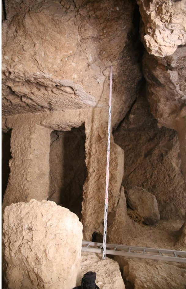
Figure 10: Main open fracture crossing the south hall of the main chamber (left). Open fracture crossing the critical pillar K (right).
