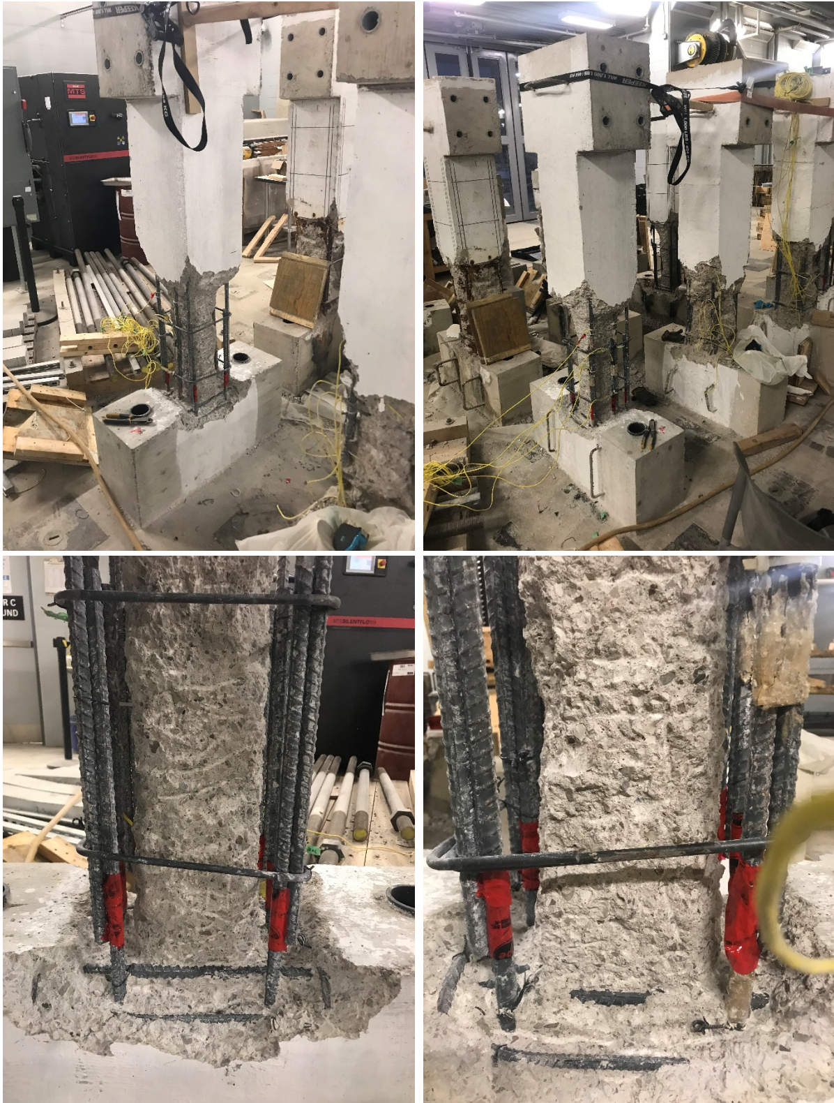
Figure C.12. Process of removal of cover and part of the core concrete for specimen CT1-15M-S.
