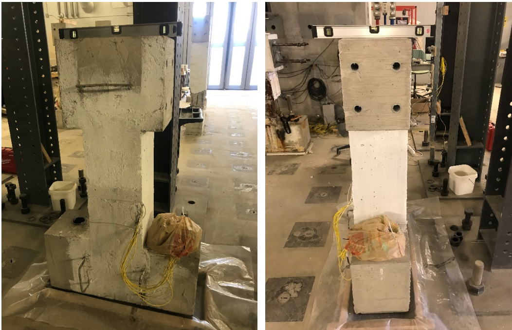
Figure 6.10. Placement of plaster layer under the column footings for leveling.
