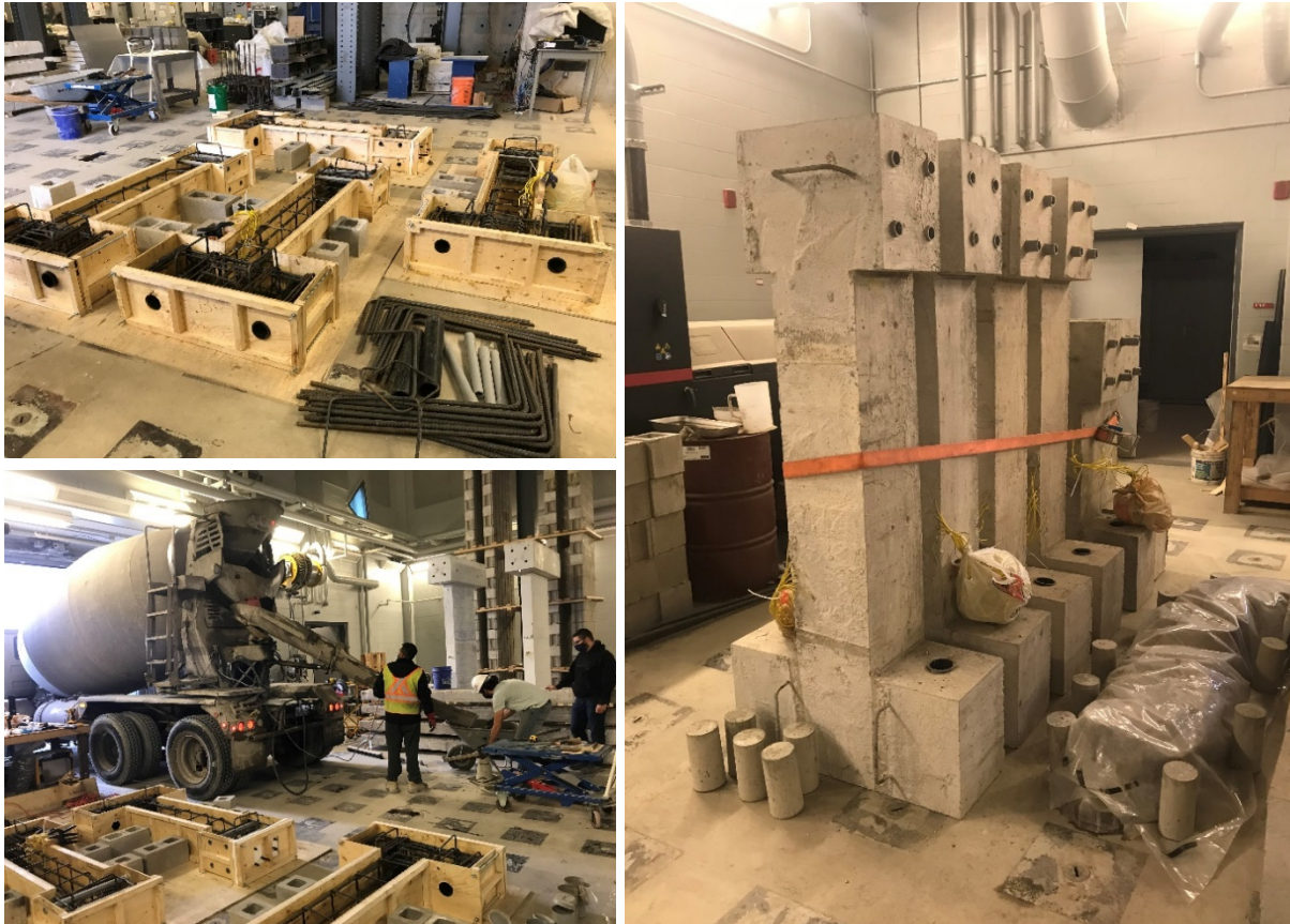
Figure C.3. Casting of specimens; total number of specimens completed.
