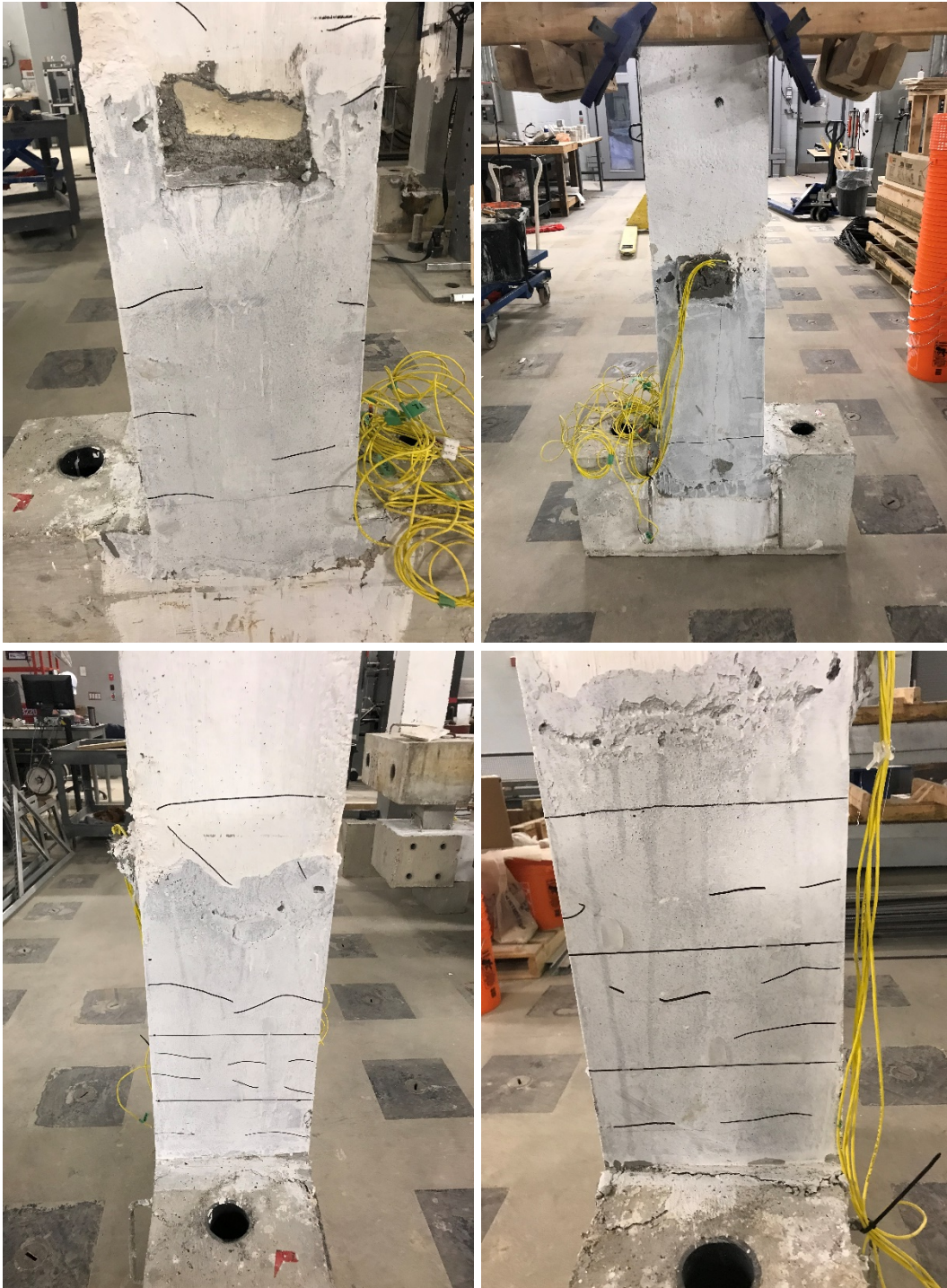
Figure C.19. Sides of specimen CT1-15M-SA after termination of test.
