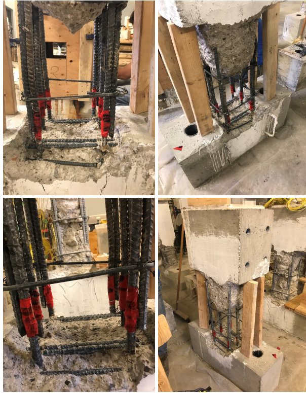
Figure C.8. Process of removal of damage cover and core concrete for specimen CS3-15M-R.
