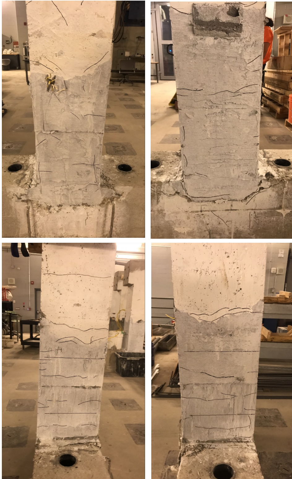
Figure C.18. Sides of specimen CT1-15M-R after termination of test.
