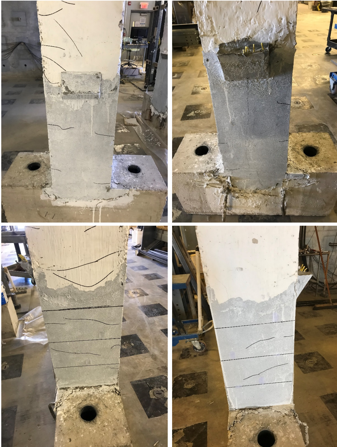
Figure C.22. Sides of specimen CT2-20M-S after termination of test.
