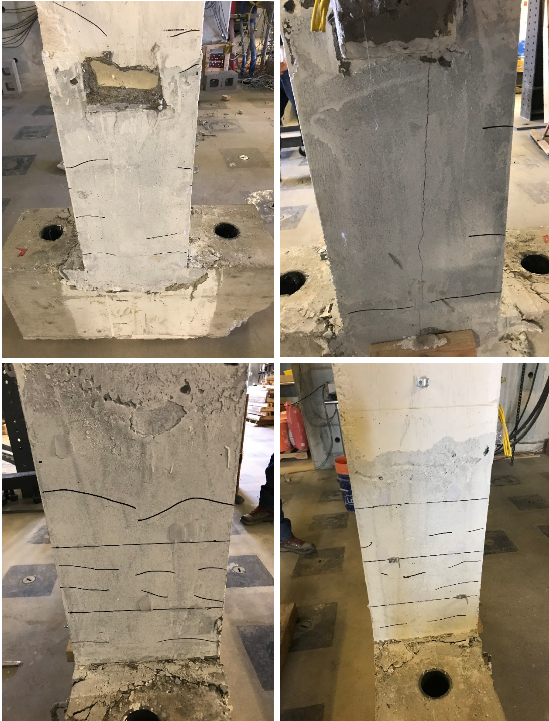
Figure C.20. Sides of specimen CT1-15M-SB after termination of test.
