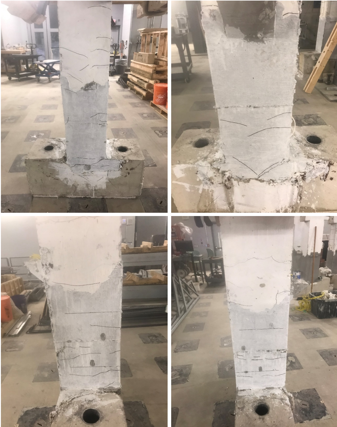
Figure C.21. Sides of specimen CT2-20M-R after termination of test.
