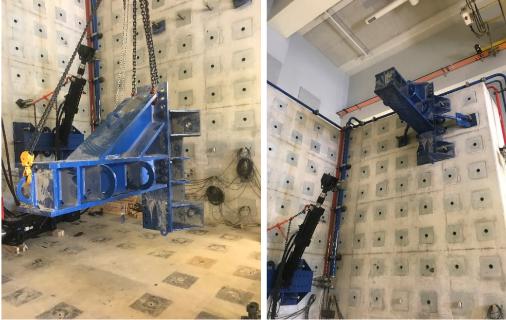
Figure 6.8. Placement of mount for vertical MTS actuator.
