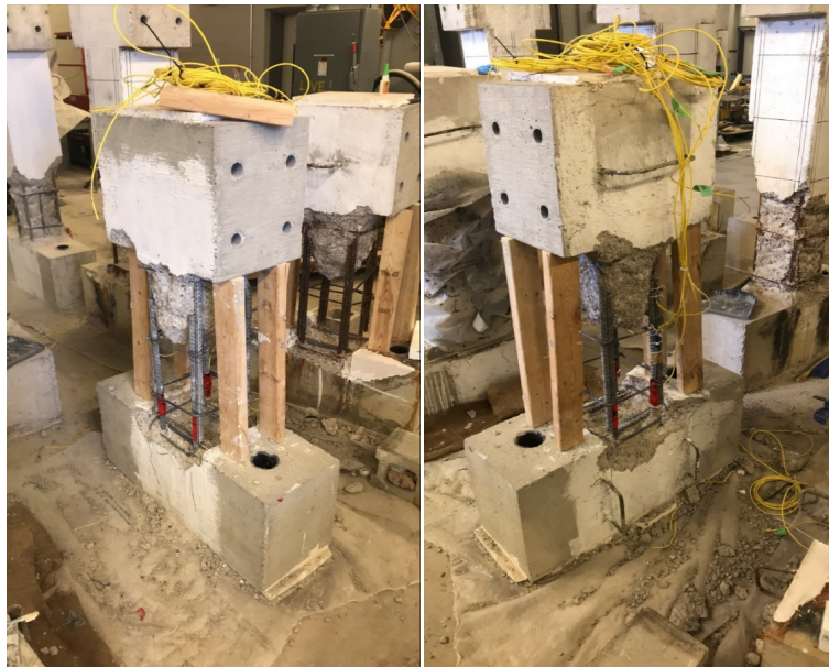
Figure C.9. Process of removal of damage cover and core concrete for specimen CS3-20M-R.
