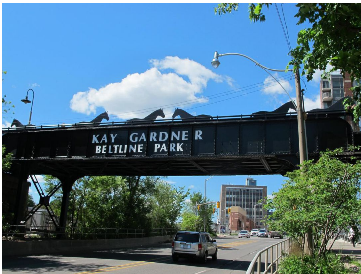
FIGURE 6-2: KAY GARDNER BRIDGE INSPIRATION FOR THE FINCH CORRIDOR. SOURCE: TORONTO STAR.
