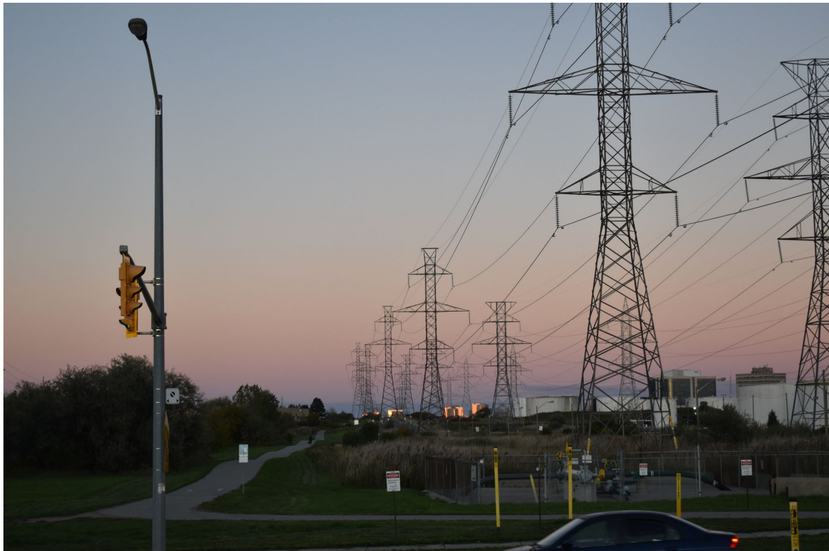
FIGURE 5-6: APPROACHING THE INDUSTRIAL SECTION OF THE TRAIL WITH VISIBLE TANK FARMS. SOURCE: ORIANA NANOA, 2021.
