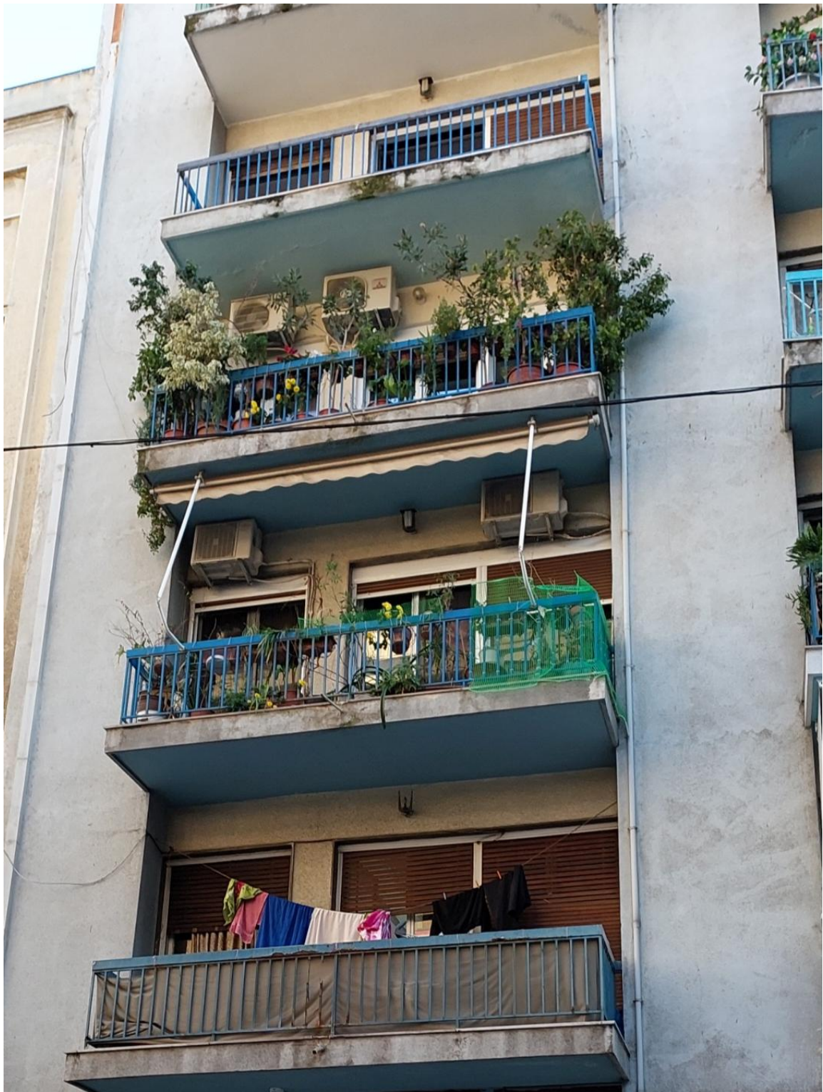
Figure 5.6: Athenian balconies in Kato Patisia (Nafsika, 2020).
