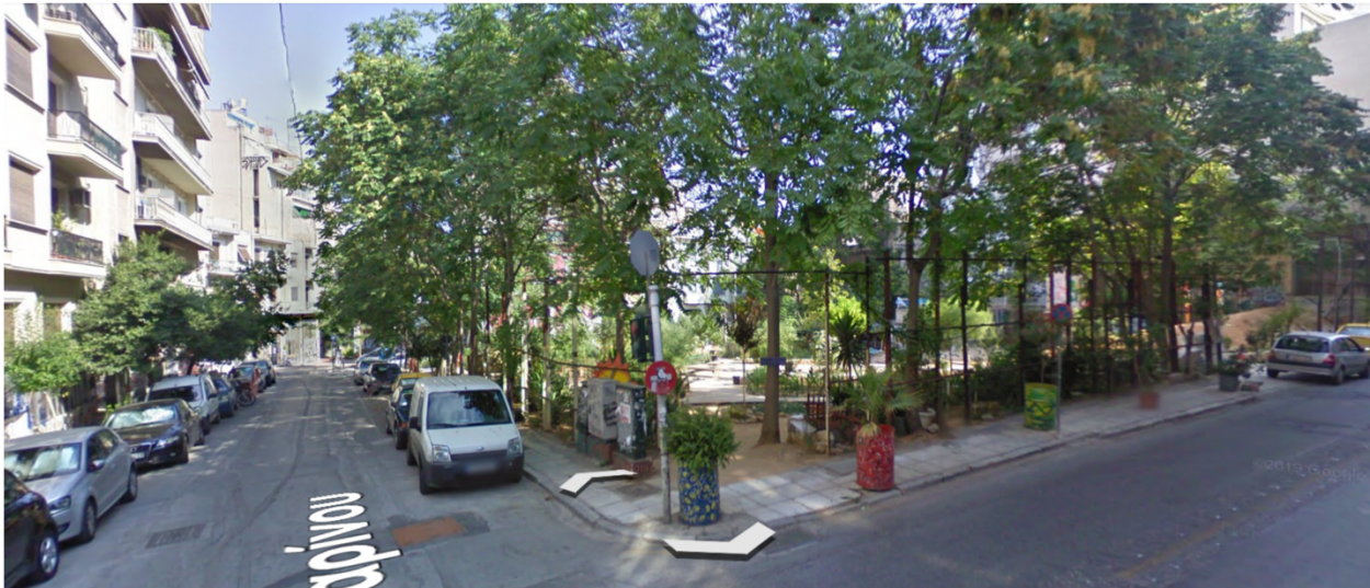
Figure 4.4: Street view of Navarinou Park, taken from Google Earth (Katsikana, 2023).
