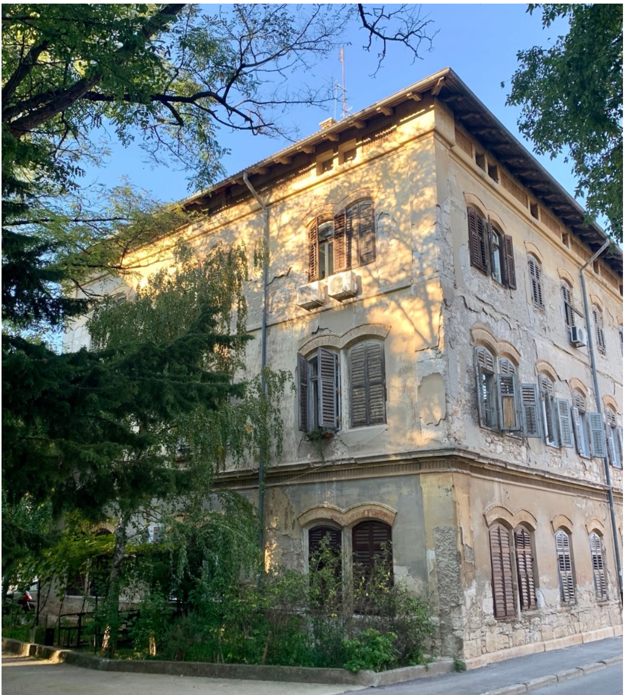
Figure 3-3, The building on the left. One of the matching buildings Gorana and I stopped in front of. Taken by Lea Alilović in October 2021.
