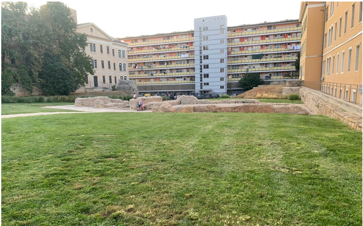
Figure 2-2, The open field behind the former knitwear factory. Initially excavated with the intent to build a parking lot. Picture taken by Lea Alilović, August 15, 2021.
