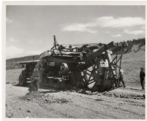
Image 10: Ditching a trench for the pipeline.
