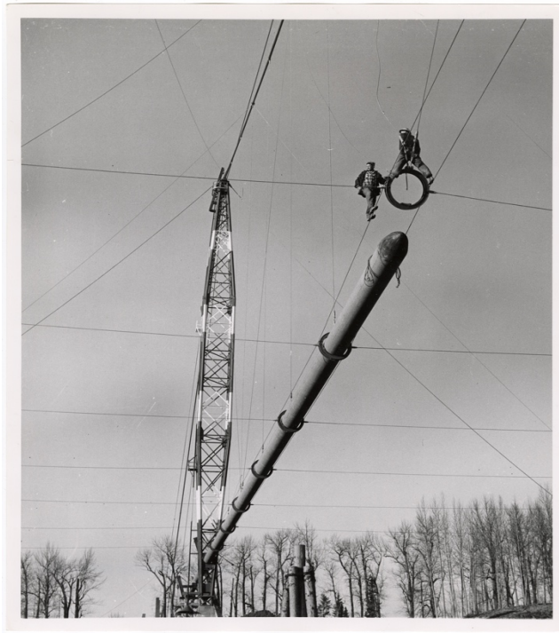
Image 25: Men balancing high above a river to string the Westcoast pipeline across.
