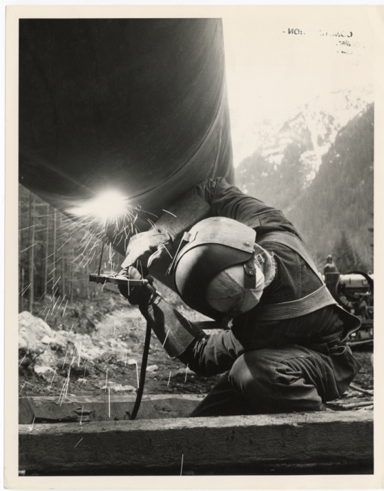
Image 12: Welding the pipe segments together.
