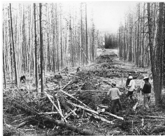
Image 8: At times, clearing the right-of-way required axes and chainsaws.
