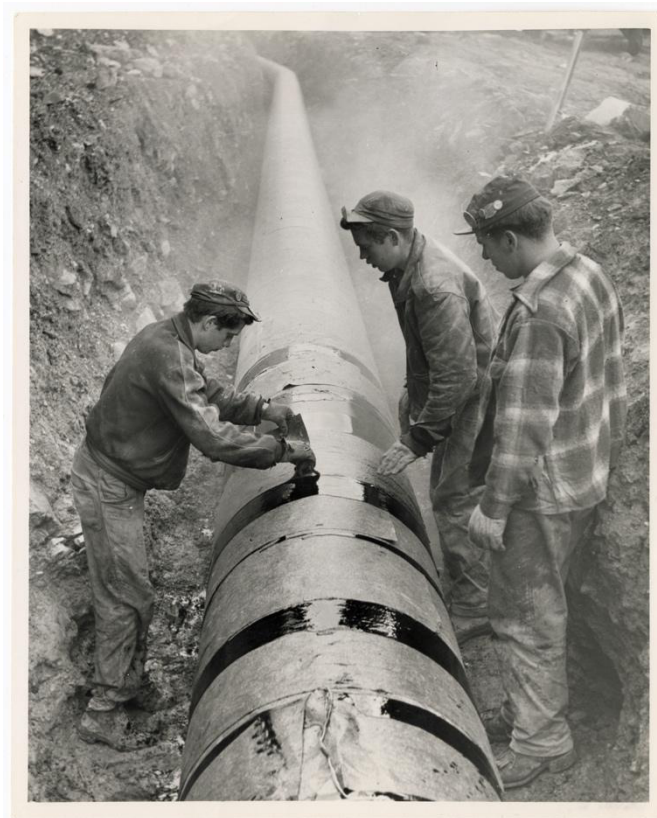
Image 14: Coating the pipeline (likely with coal tar epoxy) for protection.
