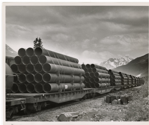
Image 9: Pipe in transit. Pipe was transported to holding locations along the right-of-way to prepare for construction.
