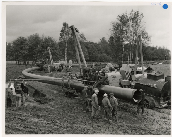
Image 13: Pipe is carefully bent to follow the route.
