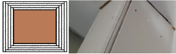
Figure 4.1 Encapsulation installation procedure of a stand-alone column (prior to gap sealing/wall finishing), representative of encapsulation used in Canadian tall timber structures (by permission).
