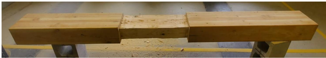
Figure B.1 Carved member before repair.
