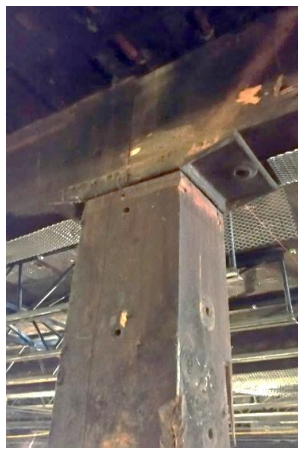
Figure 5.6 The timber column in the basement of the structure before removal.
