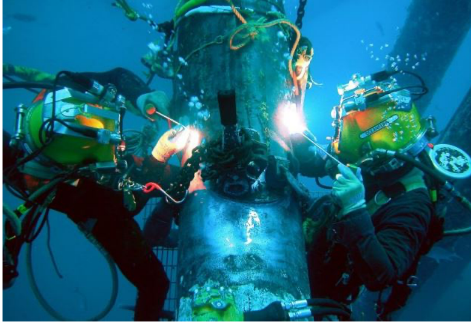
Figure 1.5: Commercial Divers at Depth A pair of commercial divers welding an underwater pipe.
