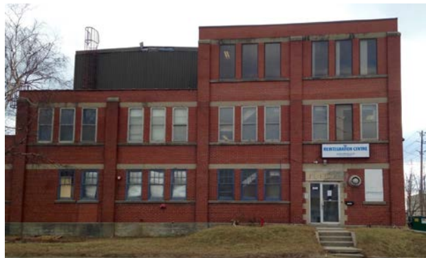
The Reintegration centre uses the first two floors of the old plastics facility—much of the building remains empty (Bahen, 2016).
