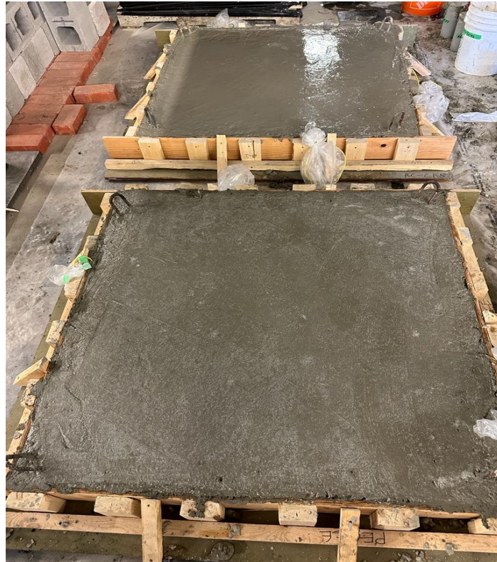
Figure B.24: Concrete Finishing
