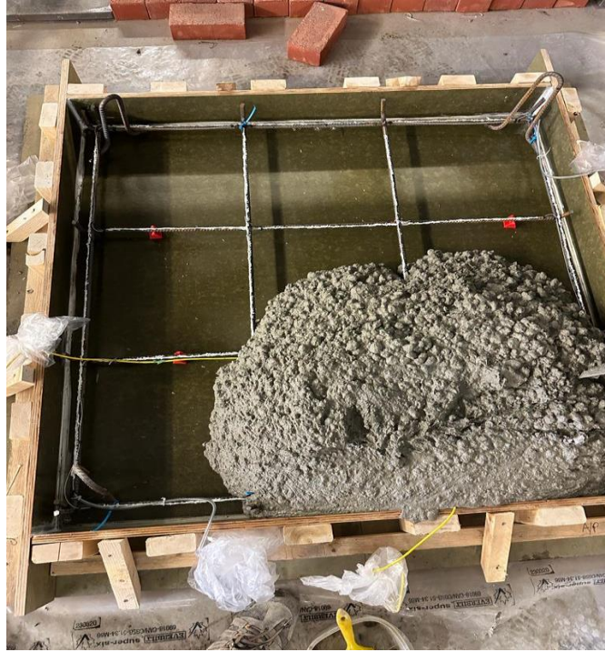
Figure B.23-Placement of the Concrete
