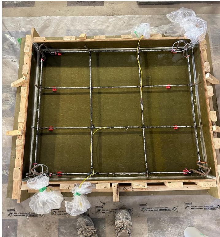
Figure B.22-Preparation for Concrete Placement into Formwork
