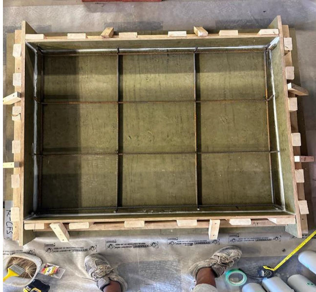
Figure B.4-The Erected Slab Formwork/As-built & Application of Sealant
