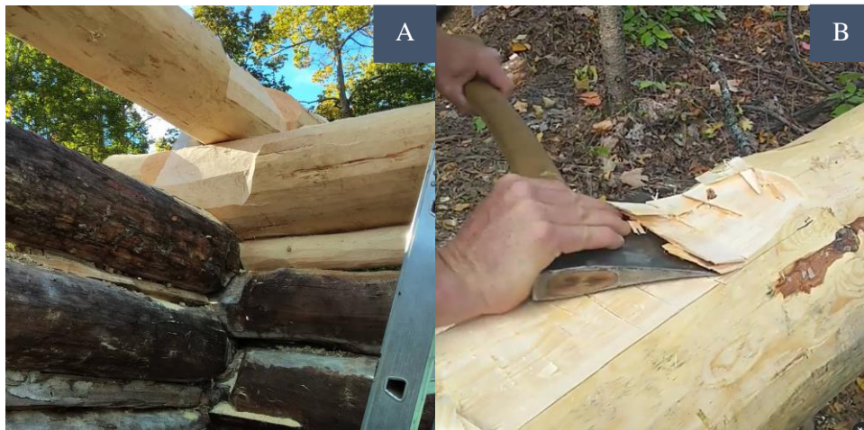
Figure 2-2: A. Replacing the top round of a heritage log cabin B. Employing traditional methods for constructing a saddle notch. Photos courtesy of Matt Davidson.
