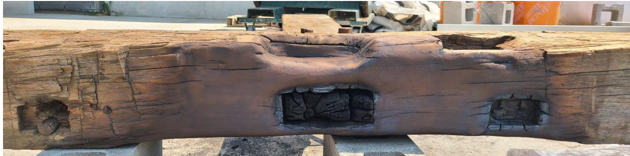
Figure 6-8: Connection with removed char
