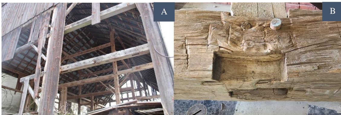
Figure 2-3: A. Dilapidated barn exposing timber frame B. Mortise and tenon connection.
