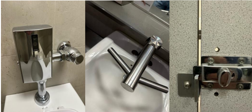
Figure 5.3a: Toilet Automatic Flush Sensor (Source: Author, 07/05/24). Figure 5.3b: Dyson 2-in-1 sink and hand dryer at Toronto's Union Station (Source: Author, 12/09/23). Figure 5.3c: Gap between stall door in toilet at Kensington Eye Institute (Source: Author, 07/05/24).
