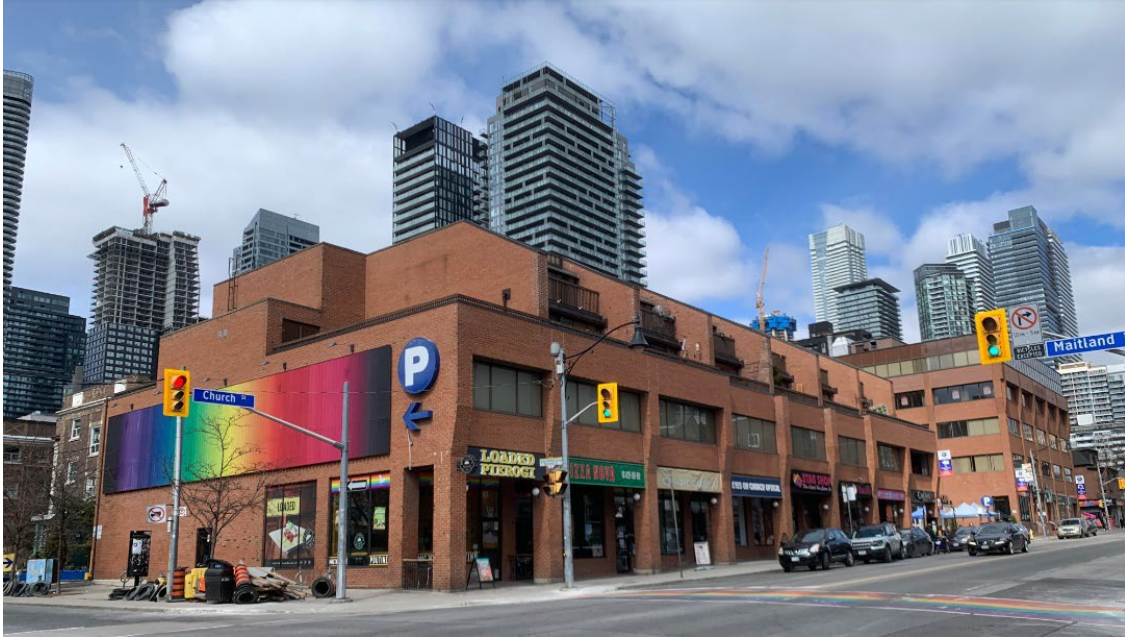
Image 50: Corner of Church and Maitland streets looking north-west with 524-540 Church Street retail residential building. Steamworks bathhouse occupies second-floor and apartments/condo units located on third and fourth floors. Source: Photo taken by author J. Gary Myers (31 Mar 2024).
