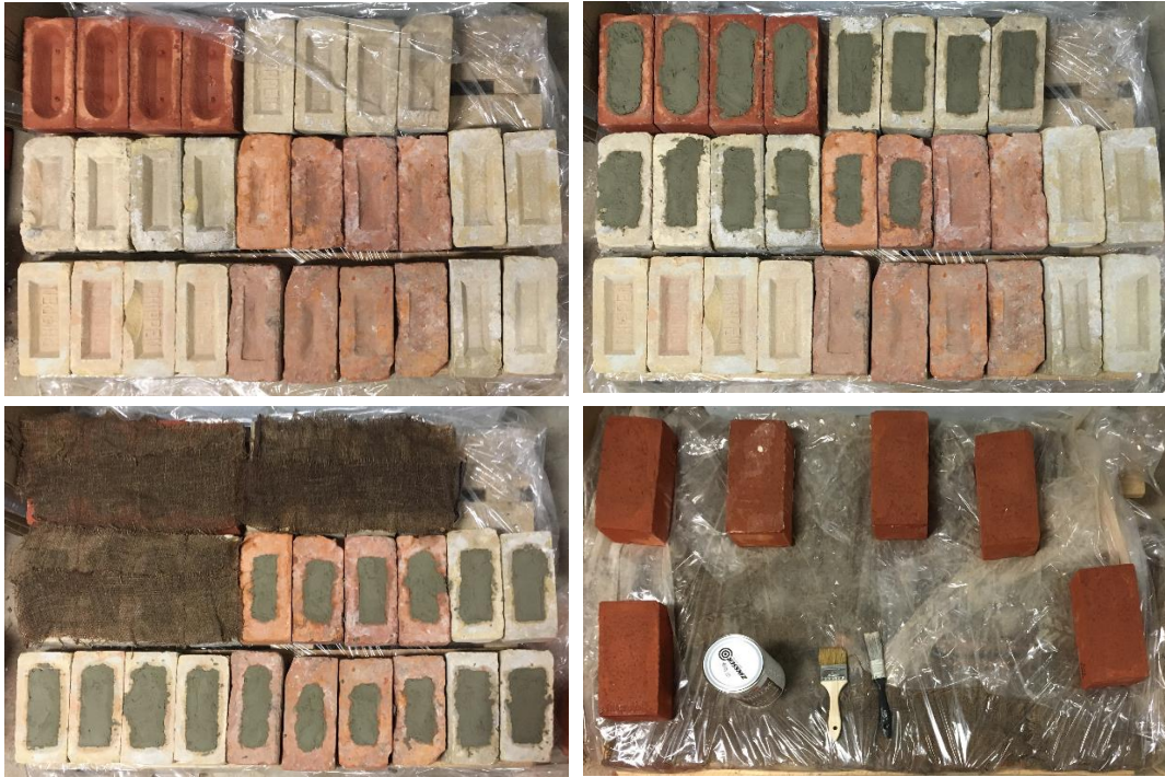
Figure 5.4. Process of filling frogs with mortar, covering with wet burlap and wrapping in plastic to moist cure for 48 hours.
