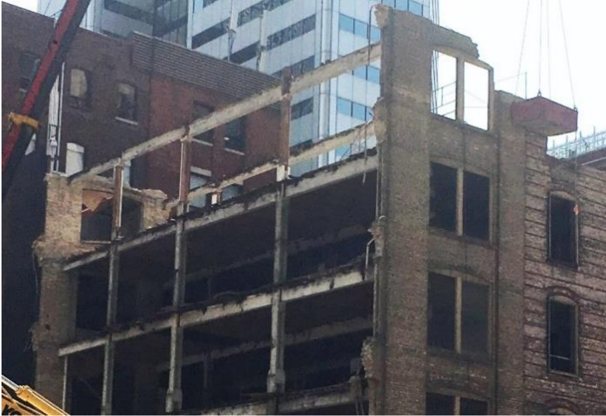
Figure 4.2. Material acquisition from an industrial building in Toronto, Canada.
