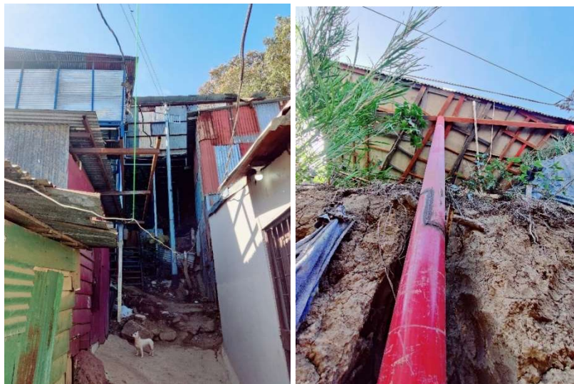
Figure 5.13. Houses built on steel piles in Bajo Zamora (Author's photos)
