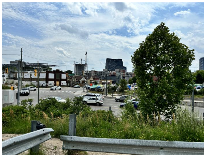
Figure 14. View of construction from the Kitchener GO parking lot. Image 3. (photo by William Overholt)
