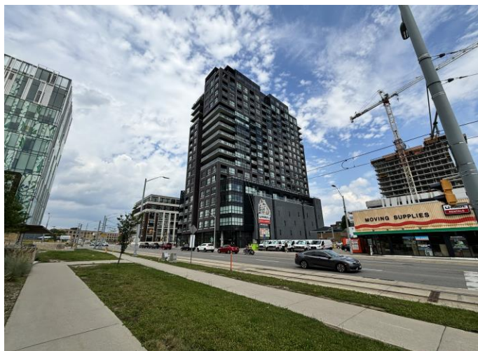
Figure 15. Newly constructed mixed-use tower and construction of a new tower. Image 4. (photo by William Overholt)
