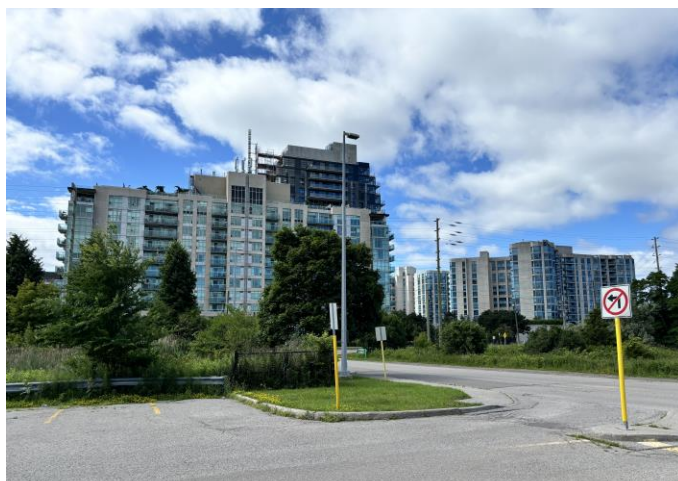
Figure 28. Recently built and currently under construction condominiums across from Whitby GO station. Image 2. (photo by William Overholt)
