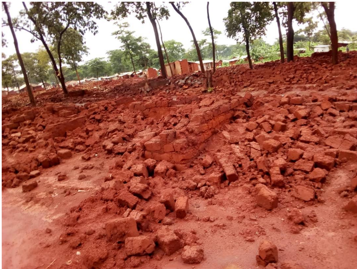
Figure 6 Nduta Zone Five Market destroyed; Sent via WhatsApp, Anonymous
