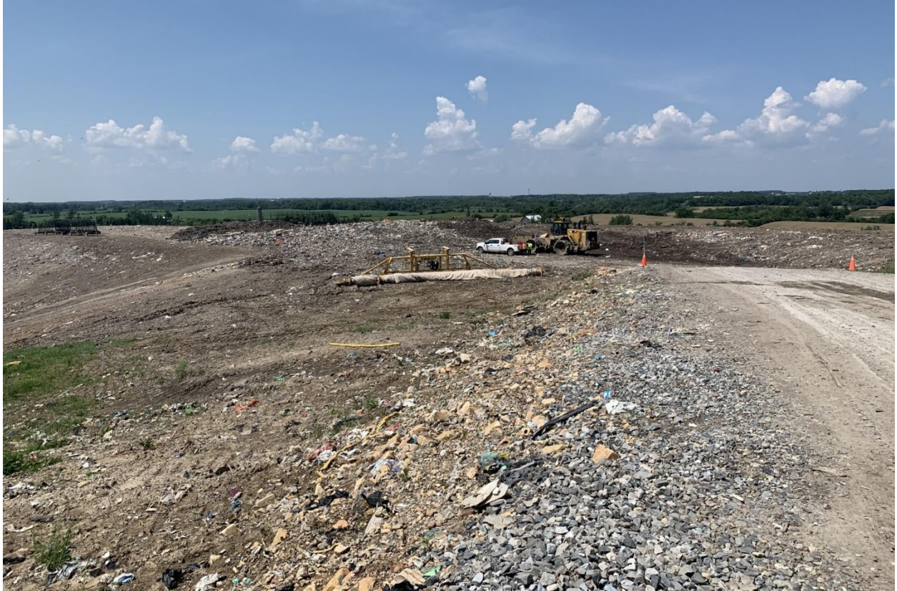
Supporting Figure 2: Close look from the top of the landfill
