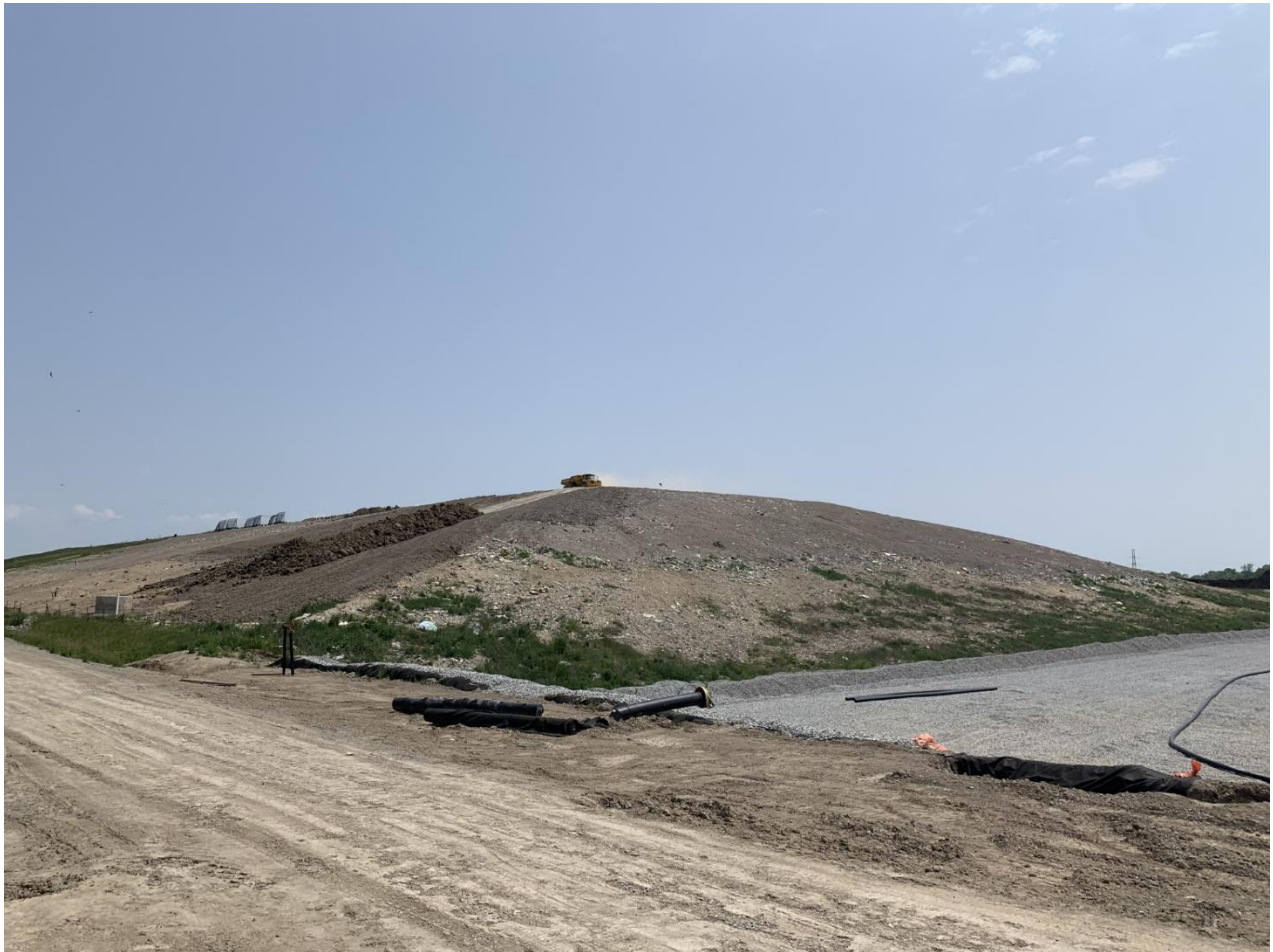
Supporting Figure 1: Landfill site view from road
