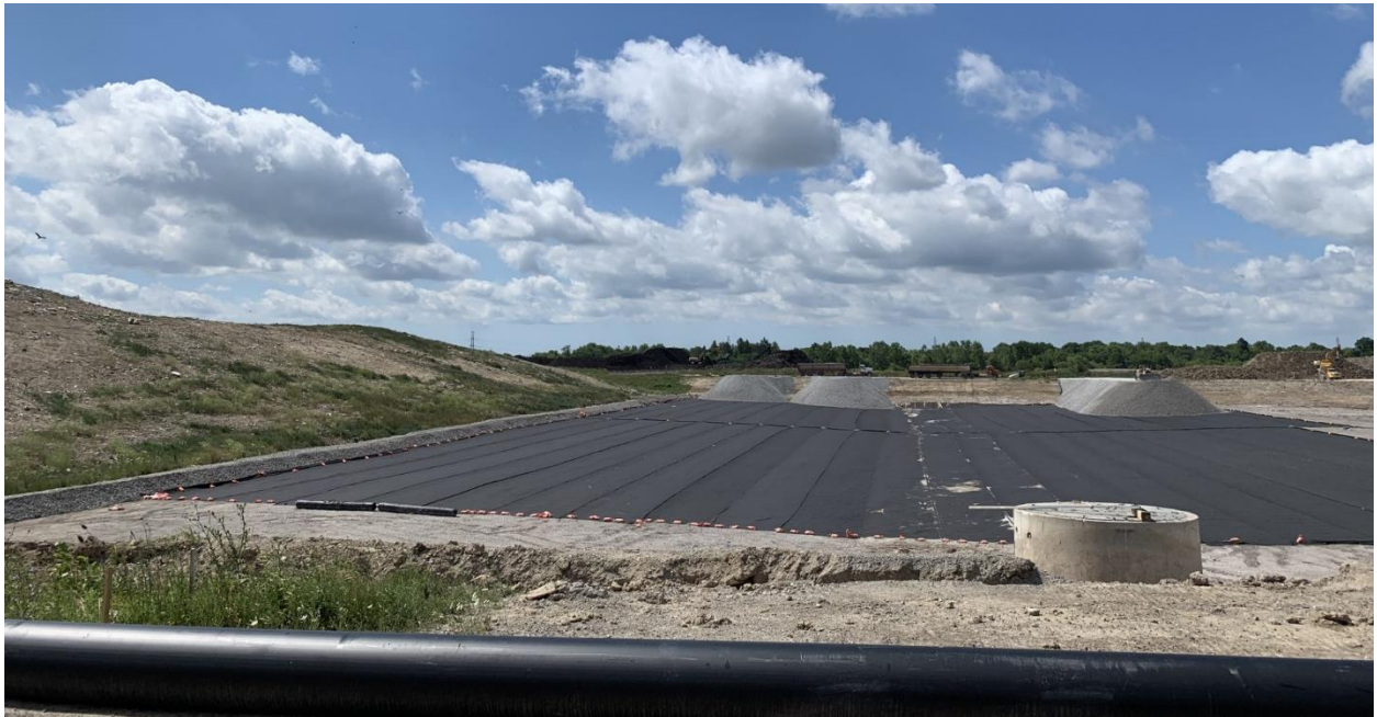
Supporting Figure 3: Constructing landfill with geotextile set on the bottom.
