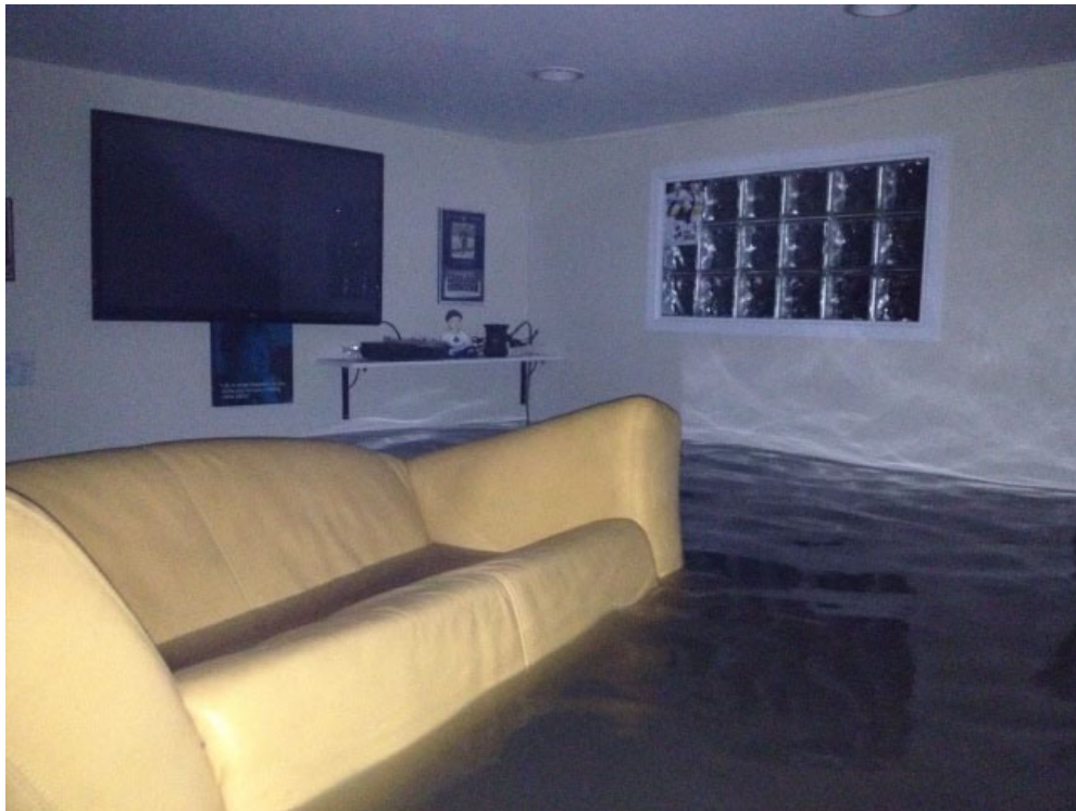
Lacaria, 2013: My basement flooded by rainwater. Personal belongings were damaged, including the couch.
