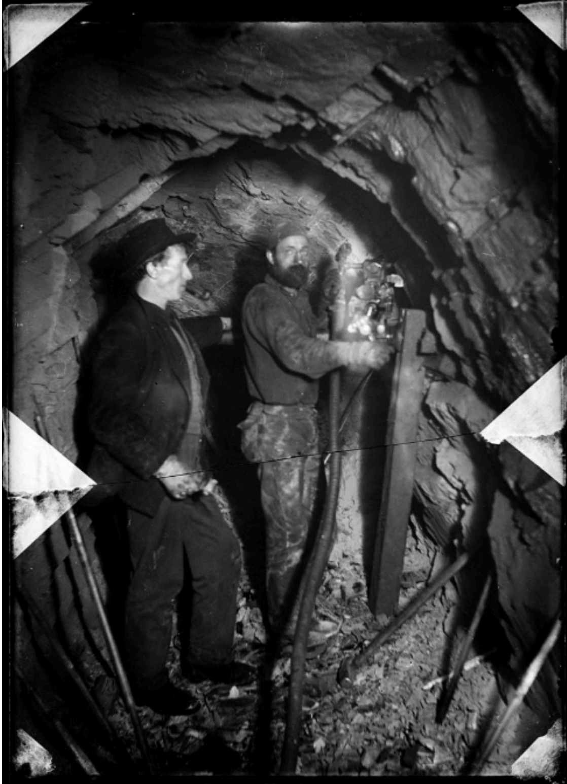
Figure 39: Mattie Gunterman, Two miners drilling inside the Nettie L. mine in Ferguson, 1902
