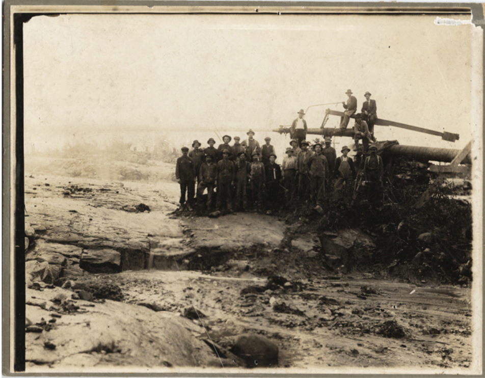
Figure 29: Hydraulic hoses used to clear off overburden, or surface material, Nipissing Mine, ca. 1906. Courtesy Cobalt Mining Museum
