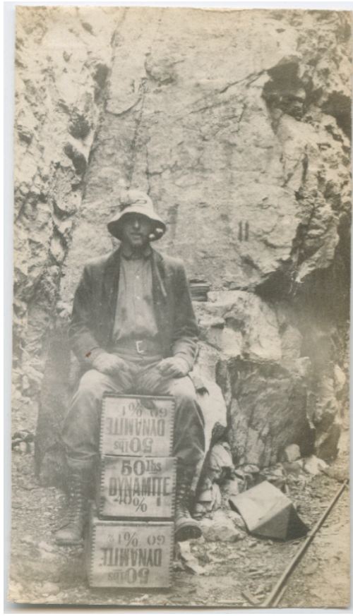
Figure 32: Worker posing with dynamite, Nipissing Mine, 1907. Courtesy Cobalt Mining Museum
