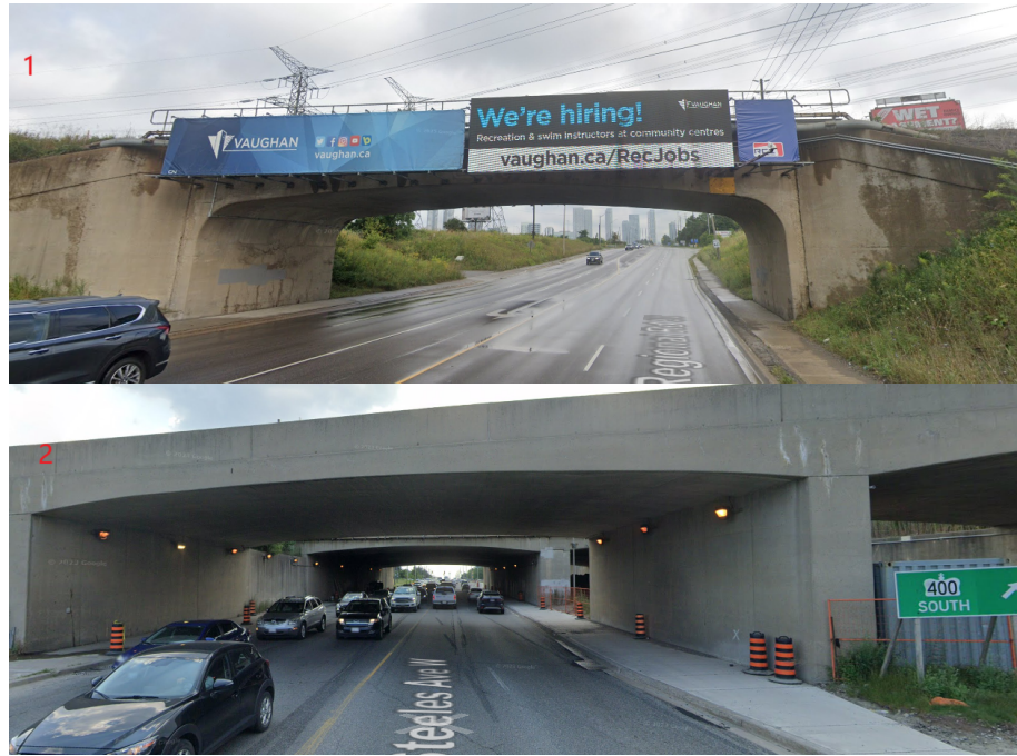
Figure 5.12: Google View of the underpasses involved in Run 3
