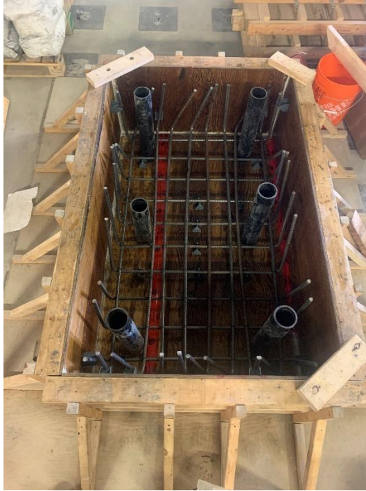
Figure 8.7: Base Formwork with Bottom Rebar Cage
