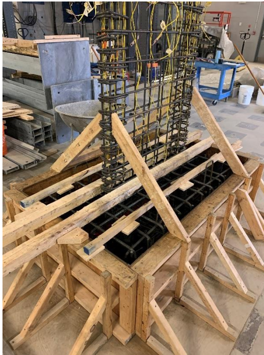
Figure 8.8: Base Formwork with Added Support Prior to Casting
