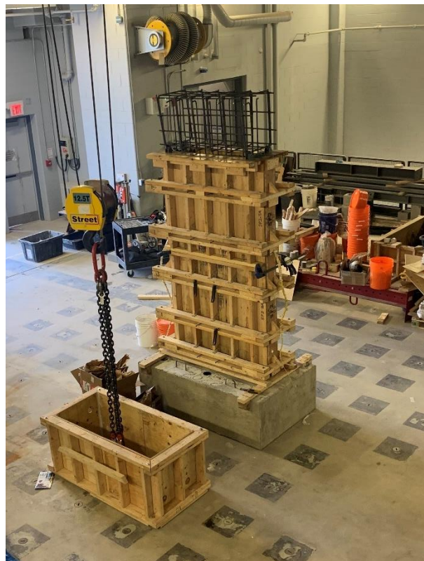
Figure 8.10: Fully Erected Wall Formwork
