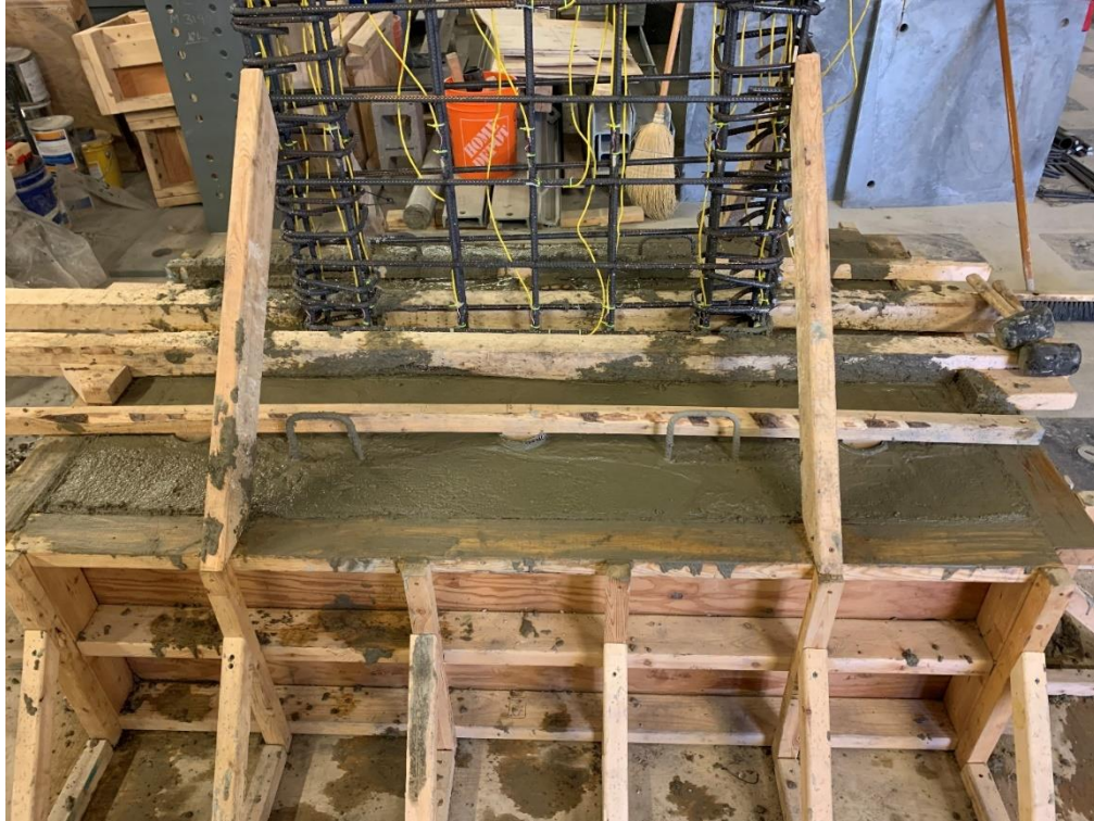
Figure 8.14: Completed Foundation Pour
