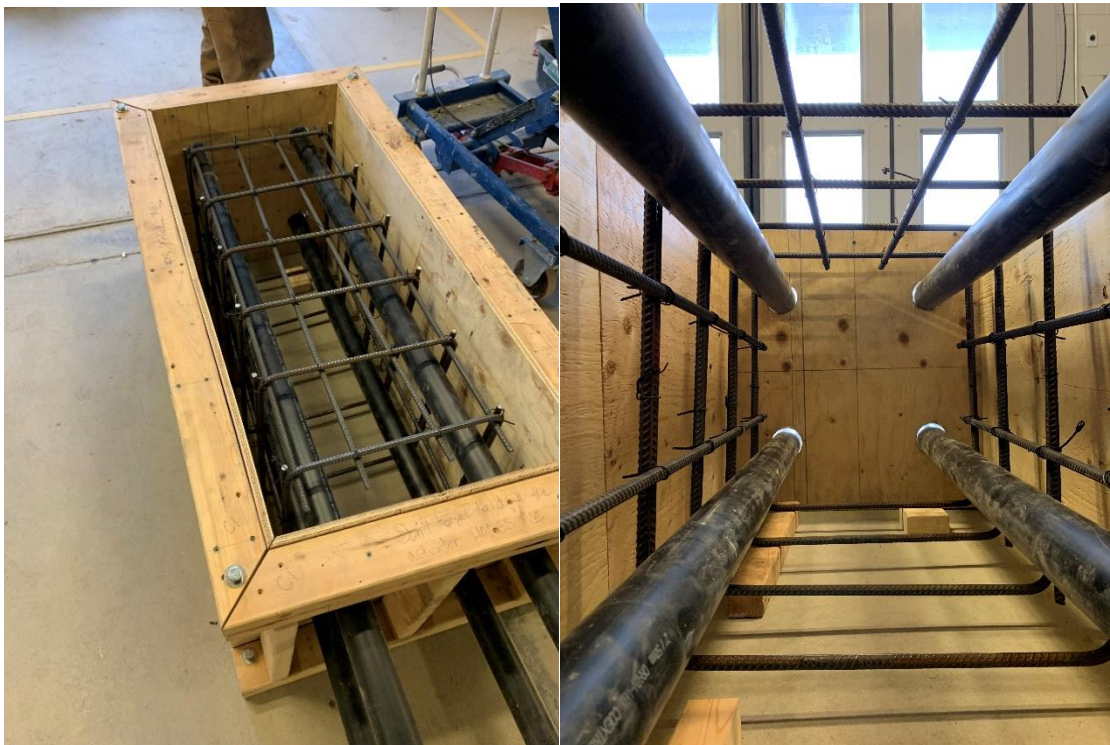
Figure 3.8: Cap Beam Formwork and Cage
