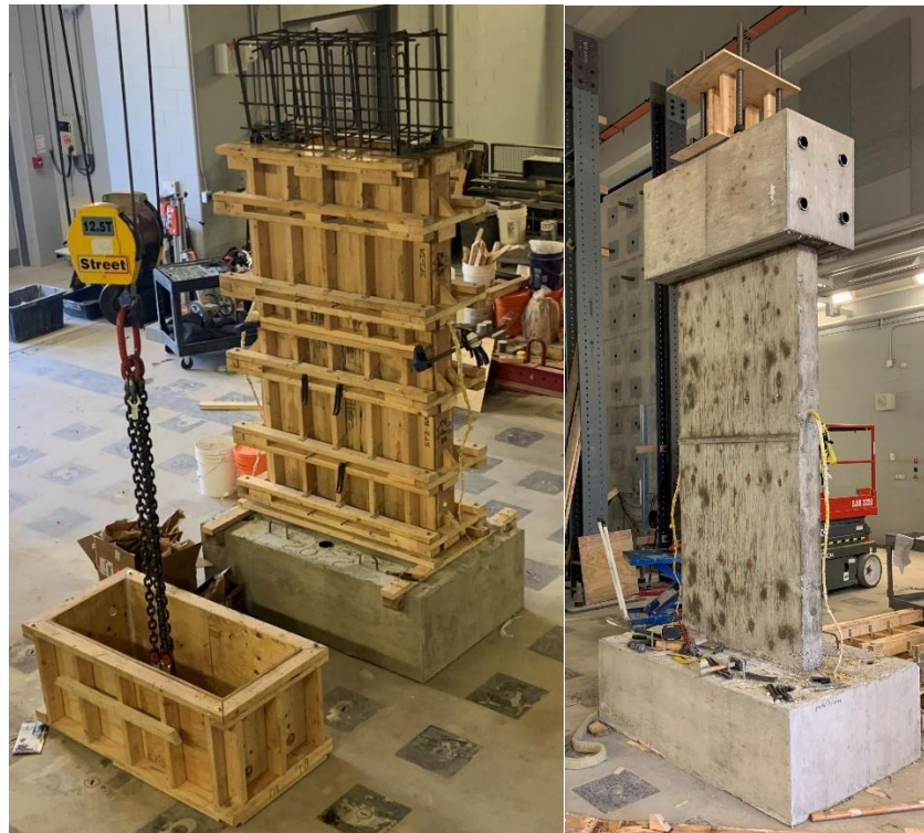
Figure 3.9: Wall and Cap Beam Formwork before (left) and after (right) Casting
