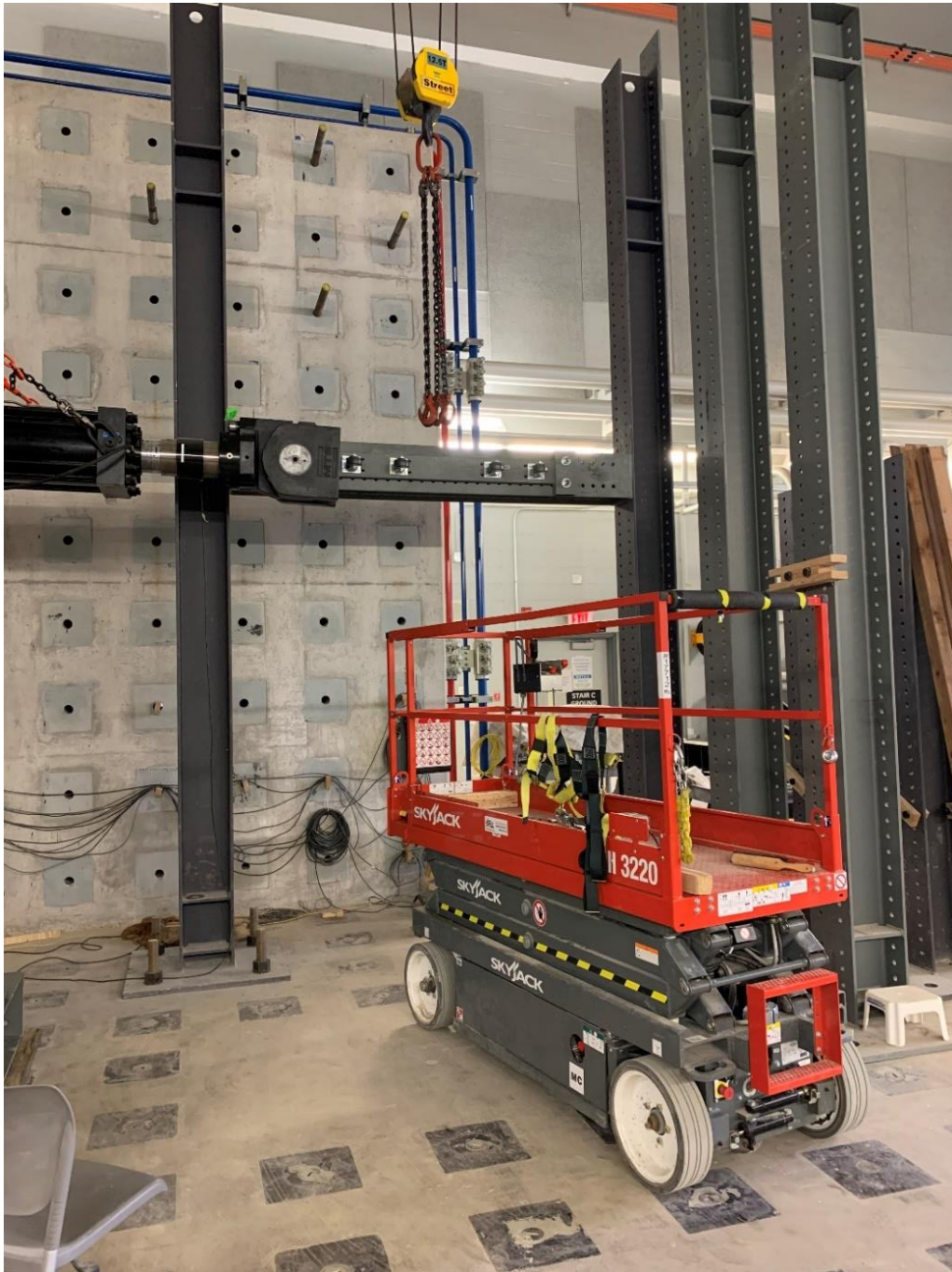
Figure 8.44: Adding First Cross Beam with Rollers
