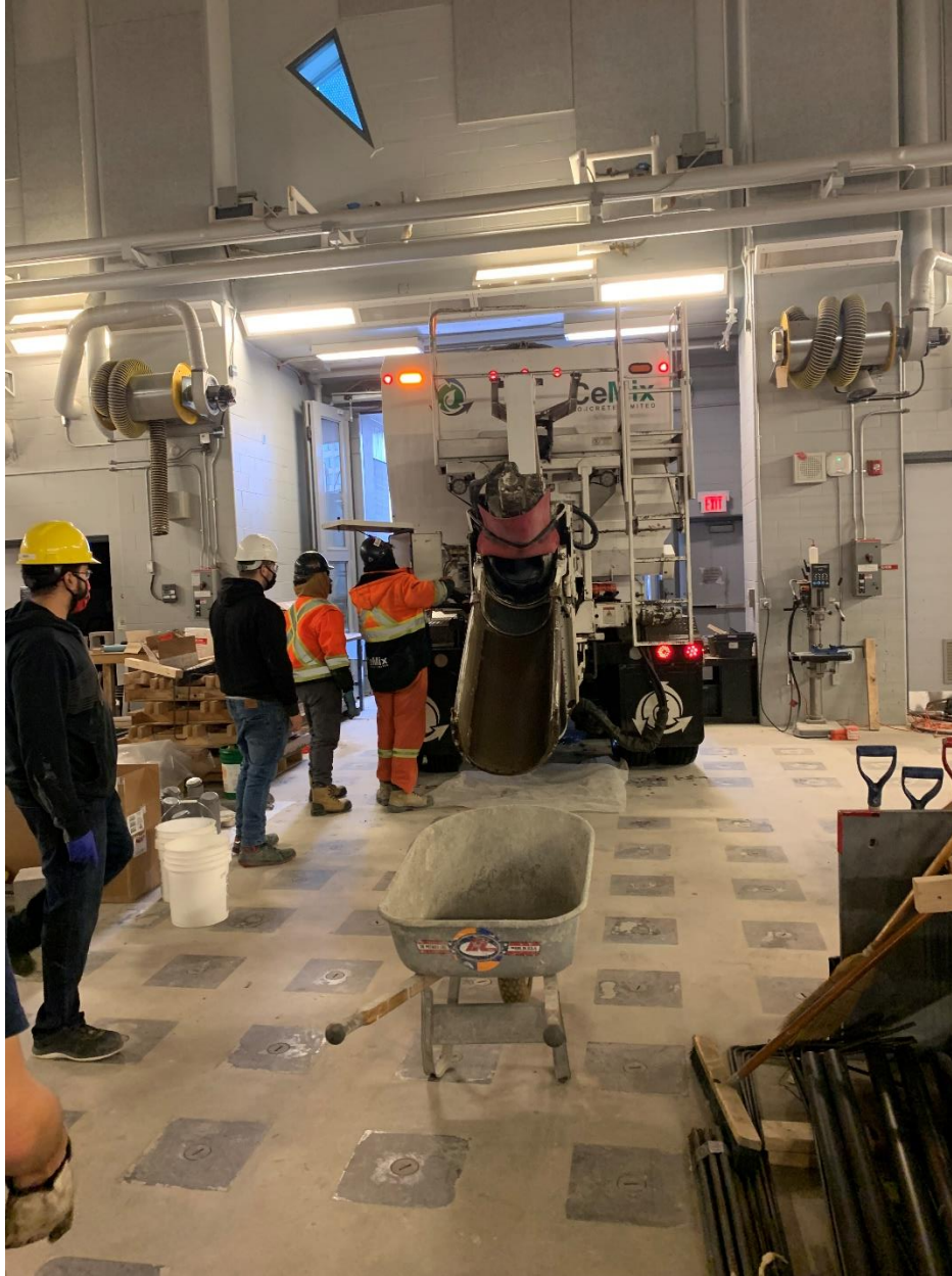
Figure 8.13: On Site Mixing for Foundation Pour provided by CeMix
