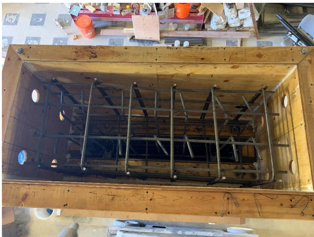
Figure 8.11: Cap Beam Formwork
