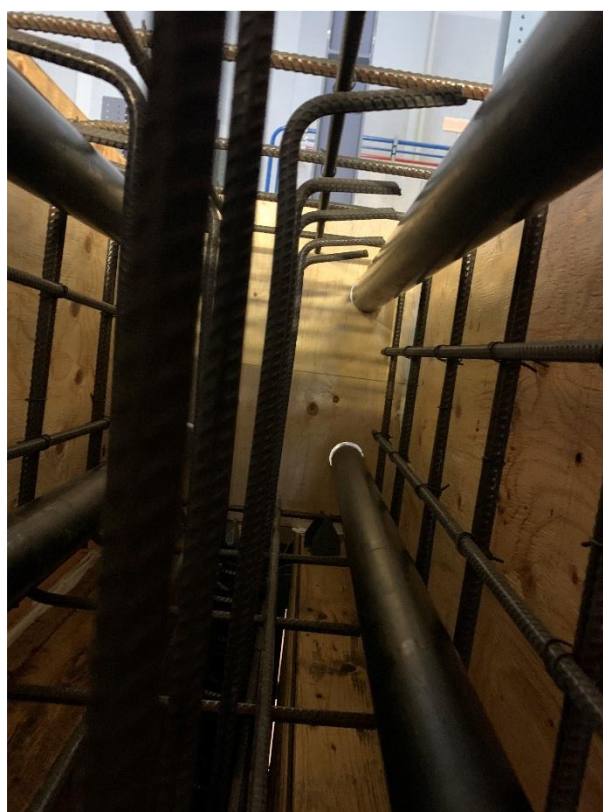
Figure 8.12: Internal View of Cap Beam Formwork
