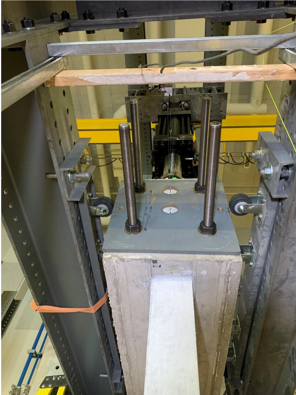
Figure 8.53: Steel Plate Modification, Below
