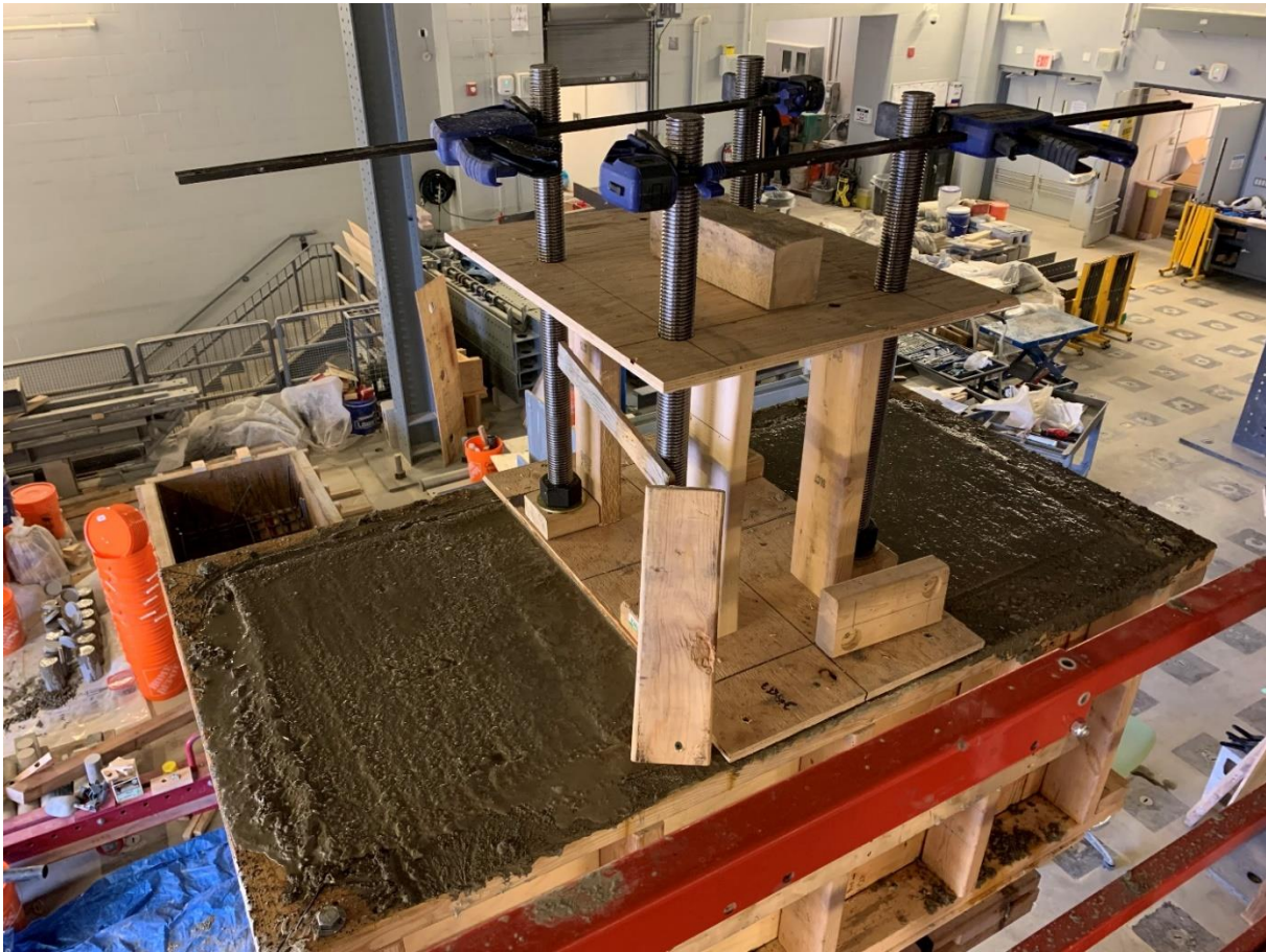
Figure 8.16: Completion of Cap Beam and Wall Pour
