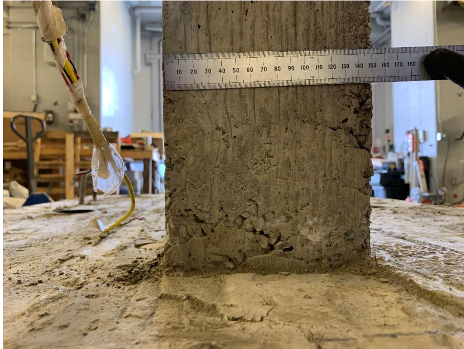
Figure 8.21: Honeycombing on Side of Wall, Actuator Side
