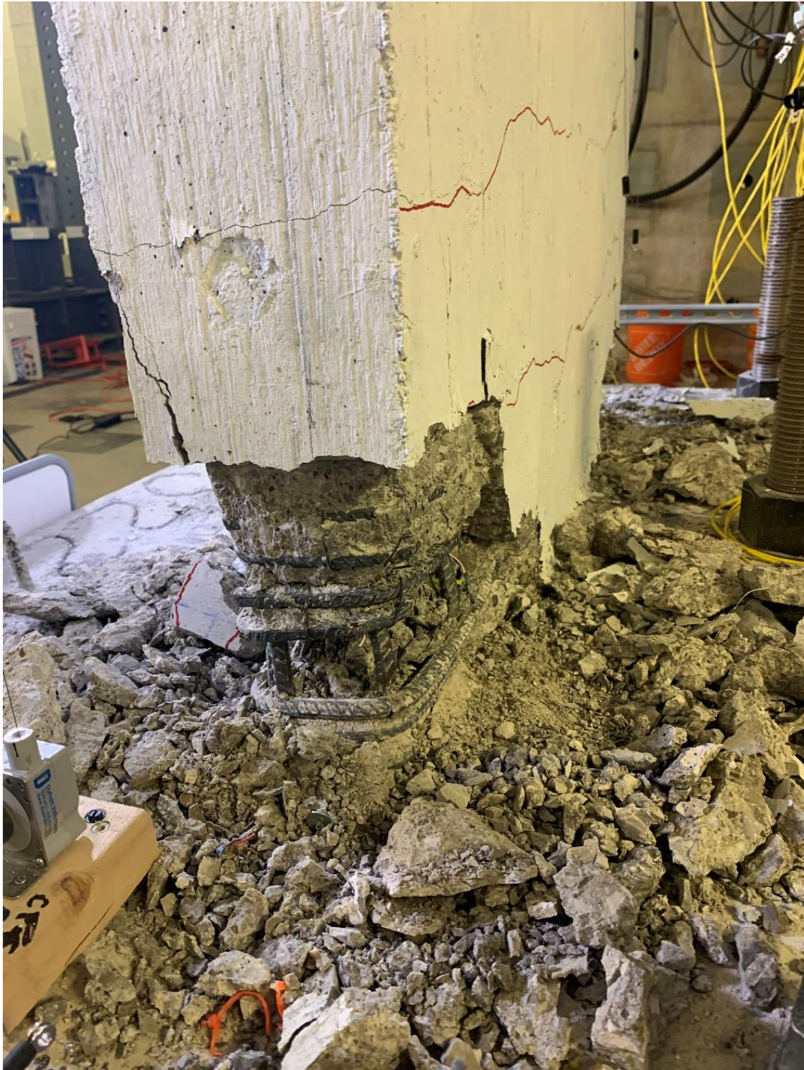
Figure 8.122: Spalling and Crushing of Concrete at Toe, Non-Actuator Side
