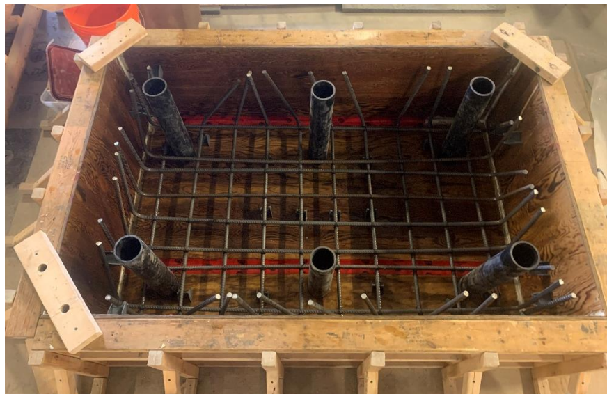
Figure 3.4: Bottom Foundation Reinforcement Cage
