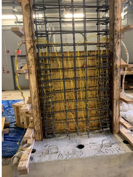
Figure 8.9: Bottom of Wall Formwork with Bulkheads
