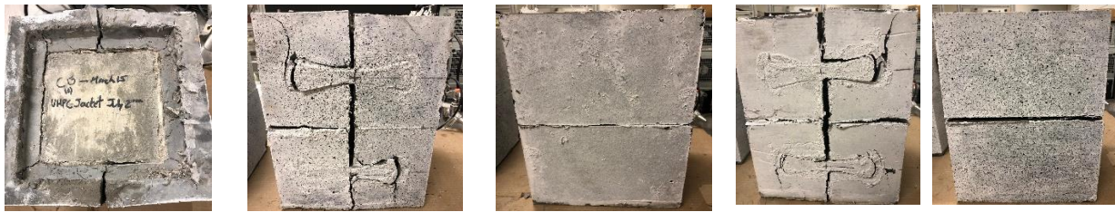
Figure 5.36. Specimen C13, precast UHPFRC Jacket with Curved Key, after testing.
