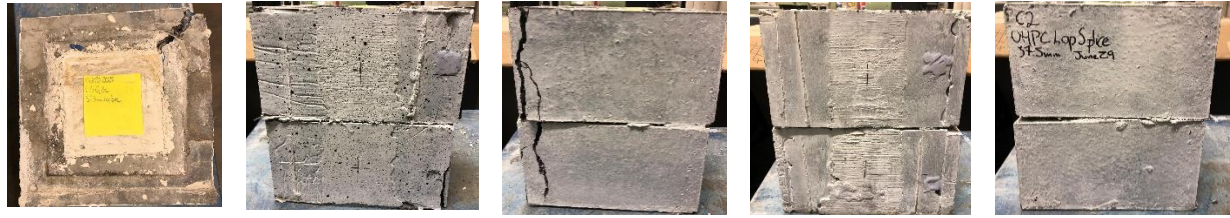
Figure 5.51. Specimen C2, precast jacket with Lap Splice Connection, after testing.
