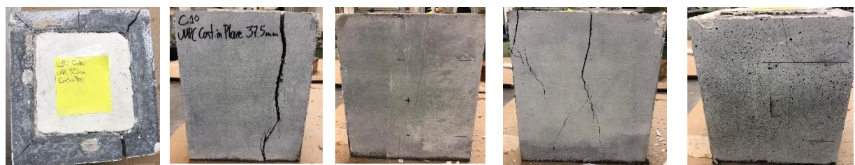
Figure 5.49. Specimen C10, cast-in place jacket, after testing.
