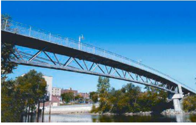
(a) Sherbrooke Pedestrian Bridge, Canada
