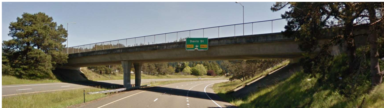
Figure 1-1 - Instrumented Painter Street Overcrossing (PSO) bridge (Goel and Chopra 1994)
