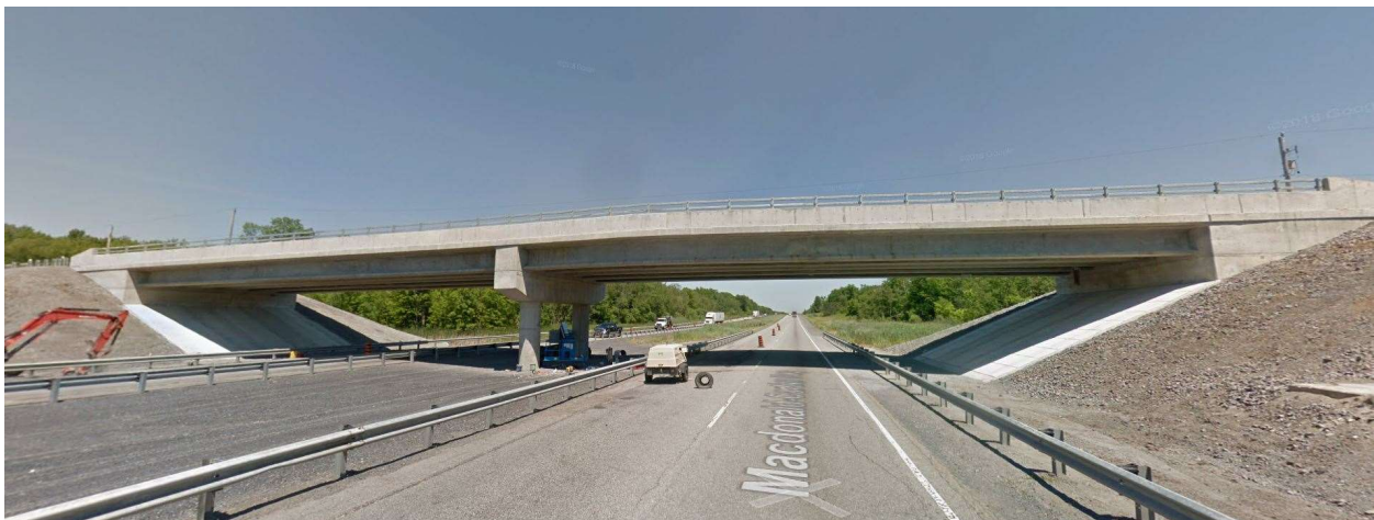
Figure 3-2 - Avonmore overpass (New structure) [Google map]
