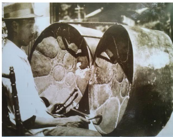
Tuner Percy "Lizard" Thomas with a double second he made with 23 notes in August 1952 from a design by Dixieland captain Ernest Ferreira
