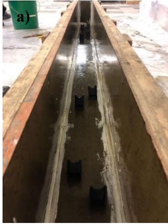
Figure 3-14. Oiled Formwork
