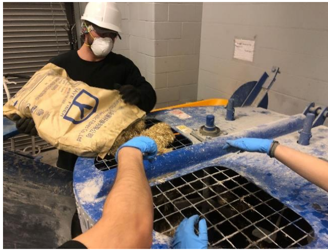
Figure 3-11. Mixing of Steel Fibres
