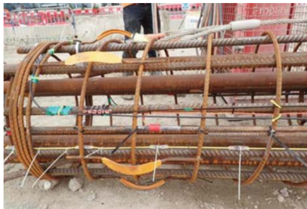
Figure 2-34. Reinforcement Cage Instrumented with Sensors (Pelecanos et al., 2018)
