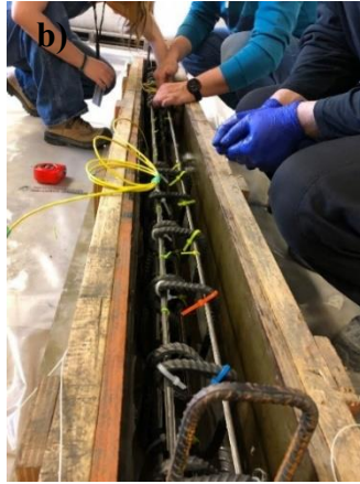
Figure 3-15. Placement of Cage in Formwork
