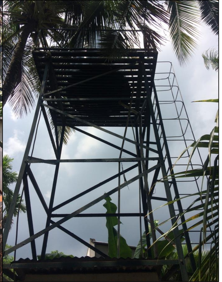
Image 2: Elevated water tank of the local water supply station in periurban district of Cần Thơ. Water is pumped up to this tank from the blue tank on the ground before it is delivered to households. Located on the property of the local water supply station manager. (personal photo)
