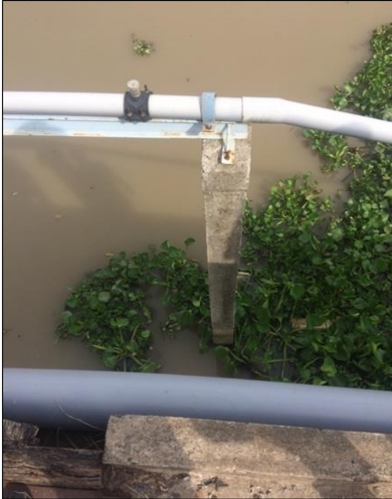
Image 5: Small and 'large' water pipe system. The small pipe goes to the commune water supply station and the large pipe goes to the district water supply station. Some periurban areas have access to both commune and district level stations. They are above ground and these are running alongside a bridge. (Personal photo)
