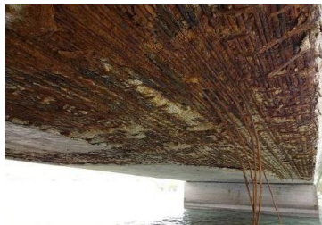
Figure 1.3: 20-year-old prestressed box-section concrete bridge over sea (Pantazopoulou et al., 2019)
