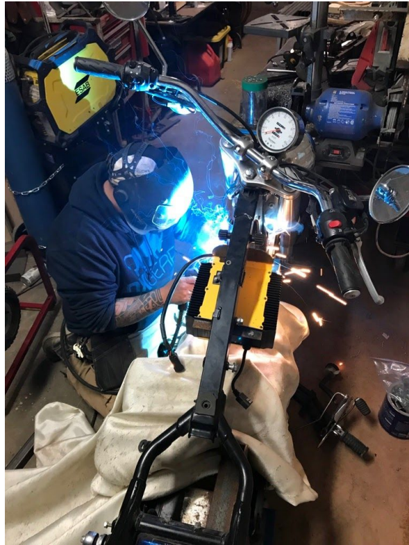
Figure 15: Delta Q charger (yellow) welded and mounted to the frame. Photo Source: Craig Stephens
