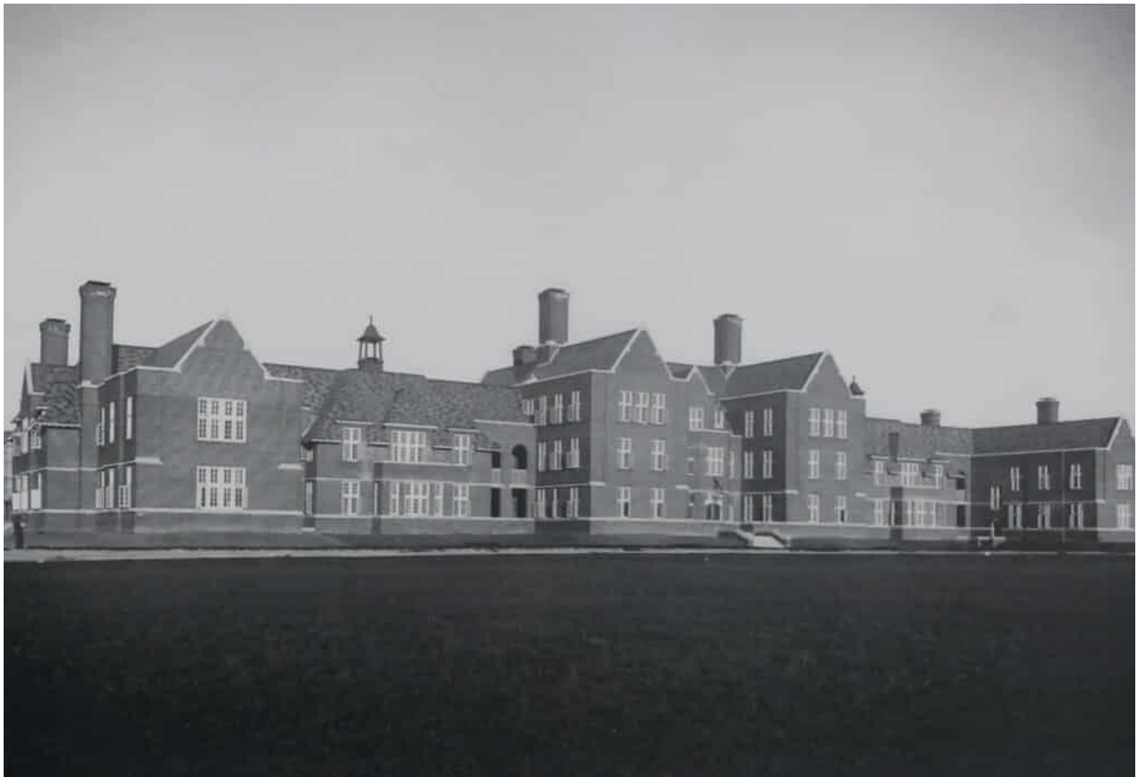
Figure 15: Reception Unit, 1923 Later Named the Dr. David Young Building in 2009, Archives of Manitoba. Accessed via the Selkirk Museum.
